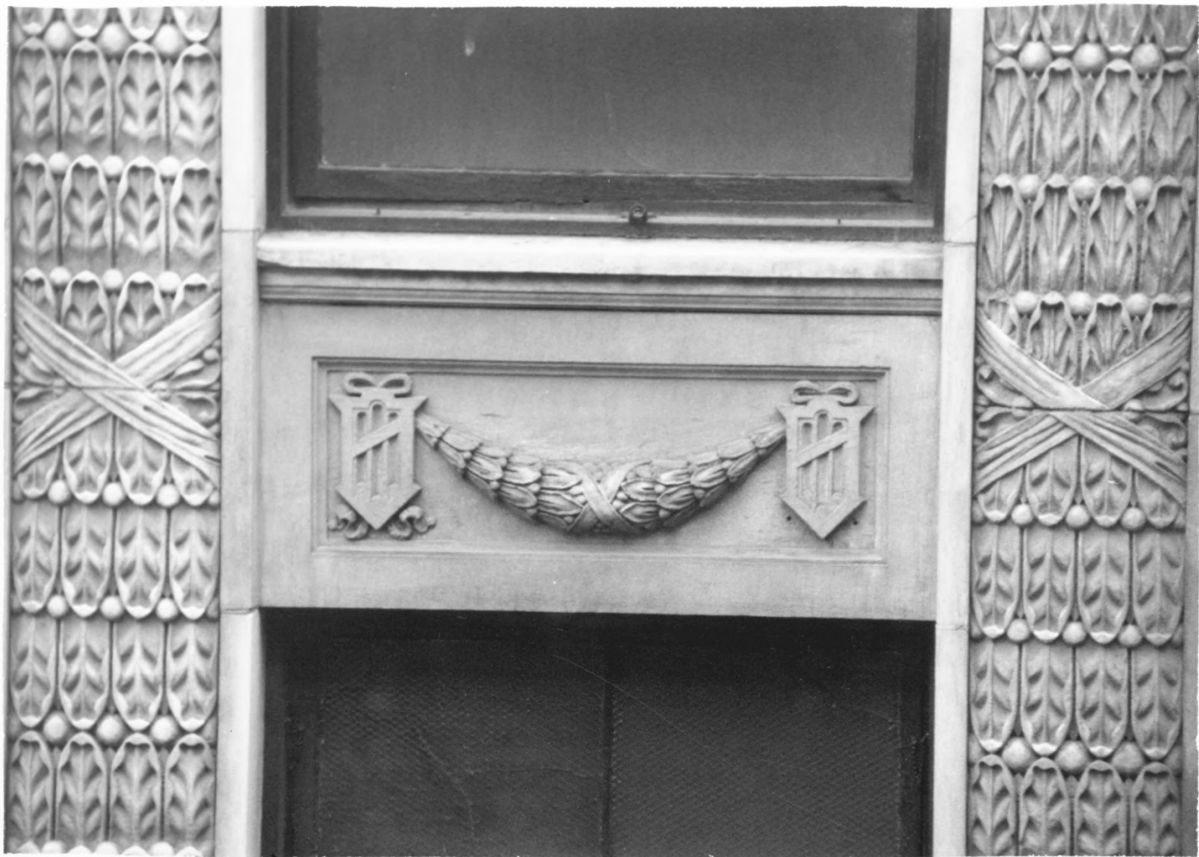
② MARMADUKE Building LOUISVILLE, JEFFERSON COUNTY, KENTUCKY
