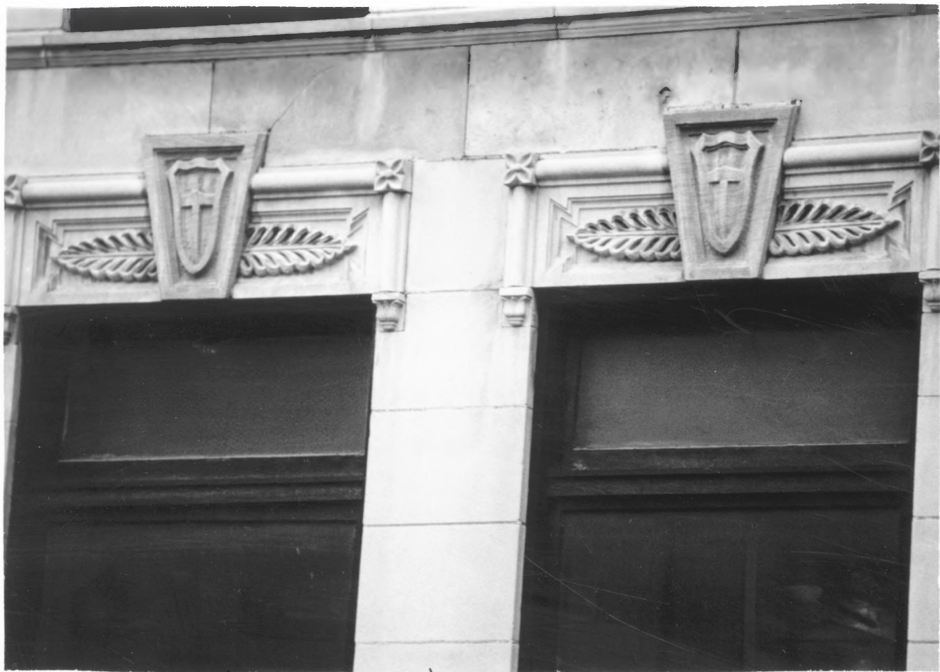
③ MARMADUKE Building LOUISVILLE, JEFFERSON County, Kentucky
