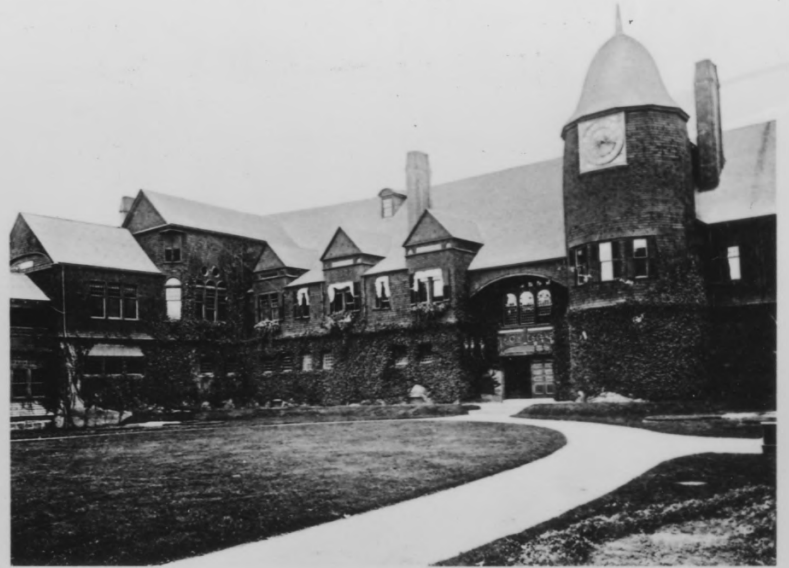
VIEW OF INTERIOR COURT
