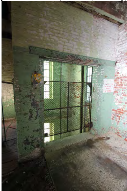
Photograph 24 – Section C, 5th floor, Elevator, view northwest
