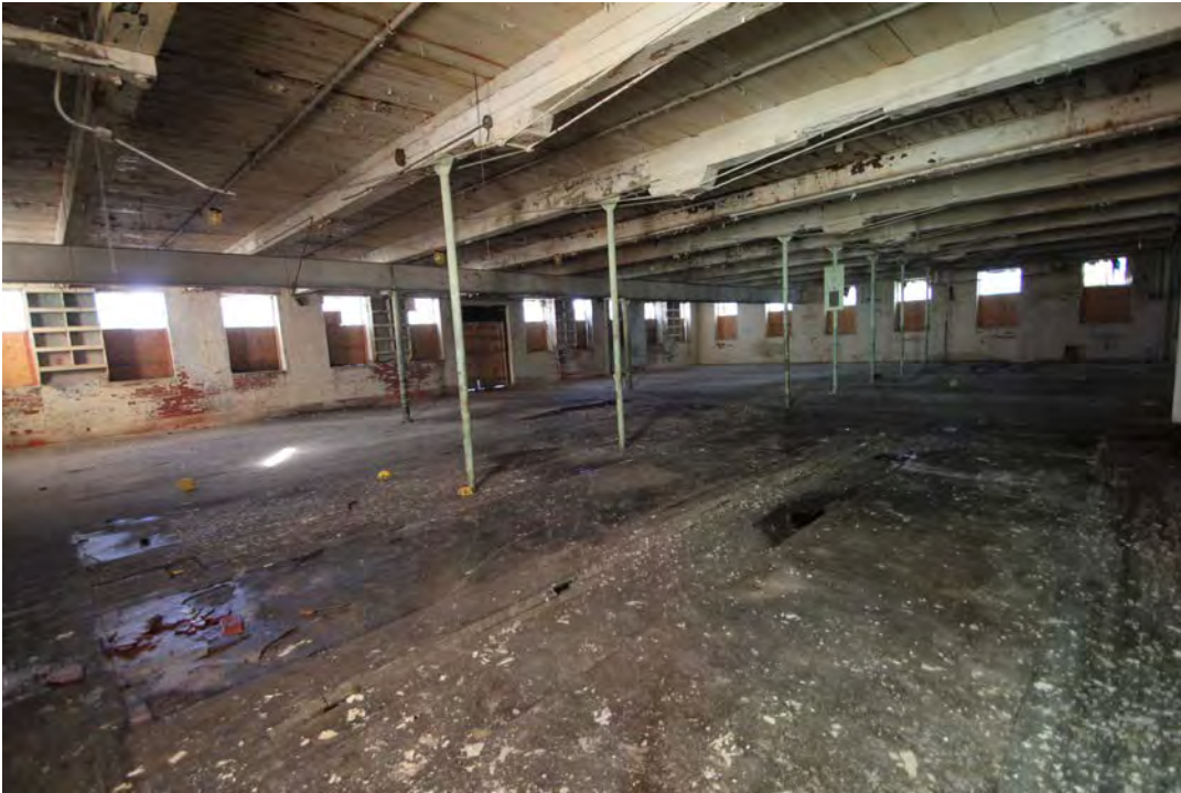
Photograph 11 – Section A, 1st floor, view northeast
