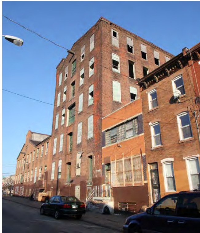
Photograph 5 – West and south elevations, view northeast
