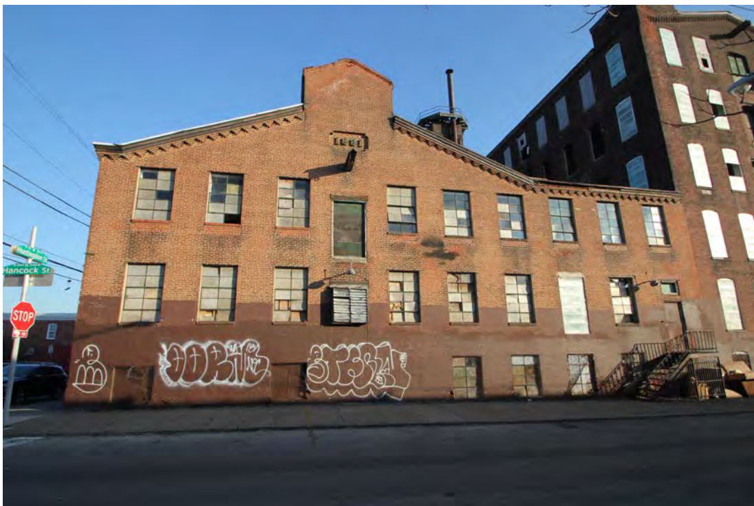
Photograph 2 – West elevation, Sections A and B, view east
