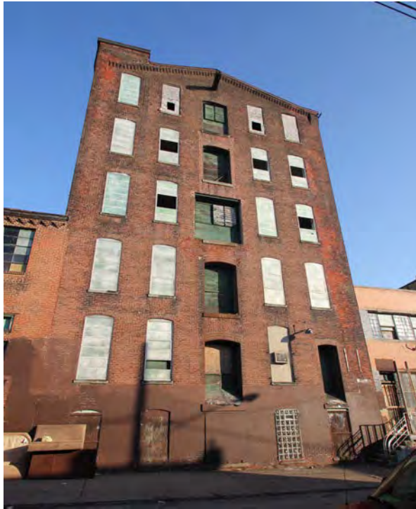
Photograph 3 – West elevation, Section C, view east
