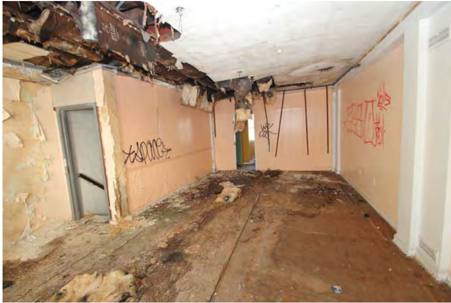
Photograph 27 – Section E, 1st floor, view east
