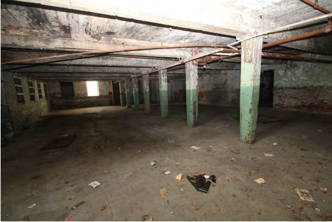
Photograph 17 – Section C, Ground floor, view west
