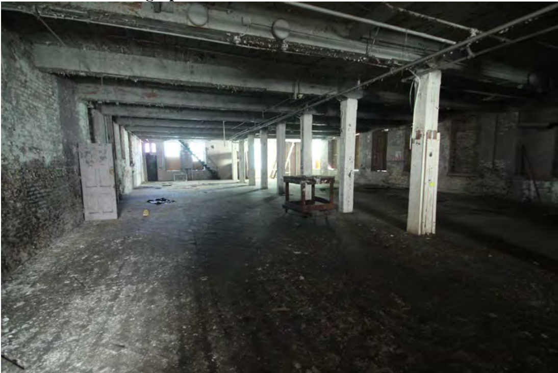
Photograph 18 – Section C, 1st floor, view east
