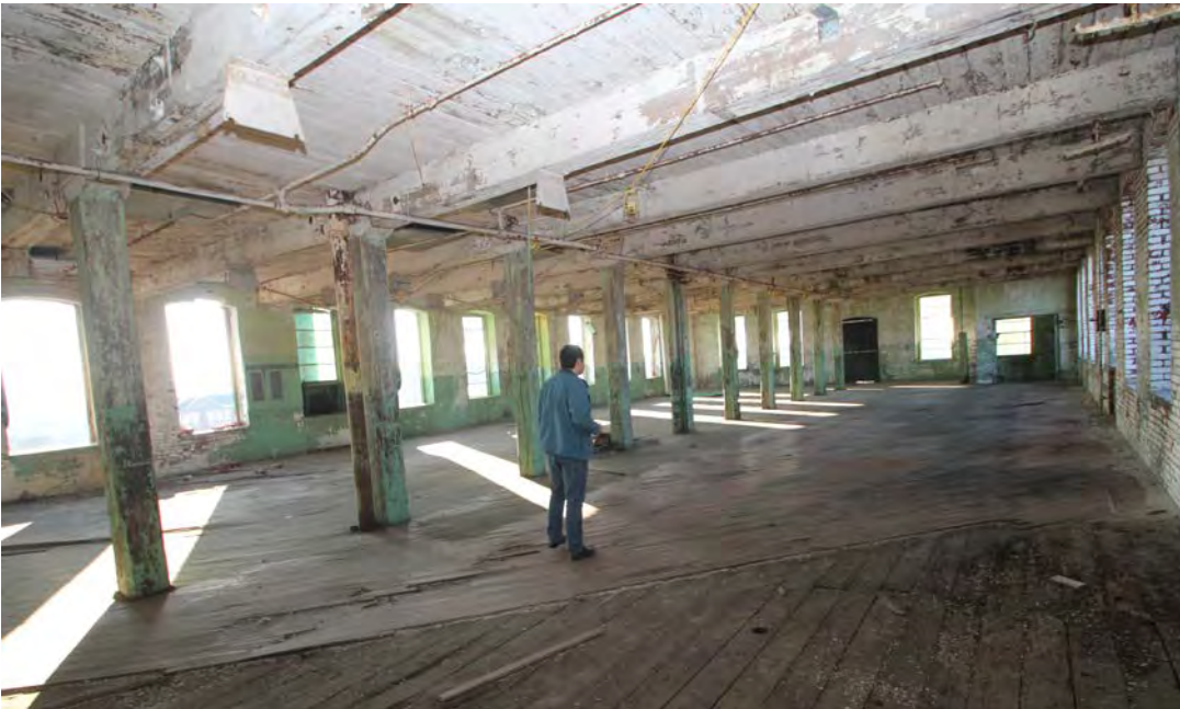
Photograph 22 – Section C, 4th floor, view southwest
