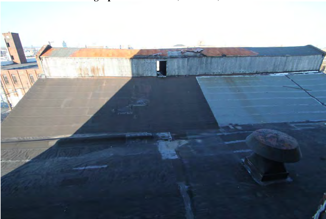
Photograph 20 – Section A, Roof, view north
