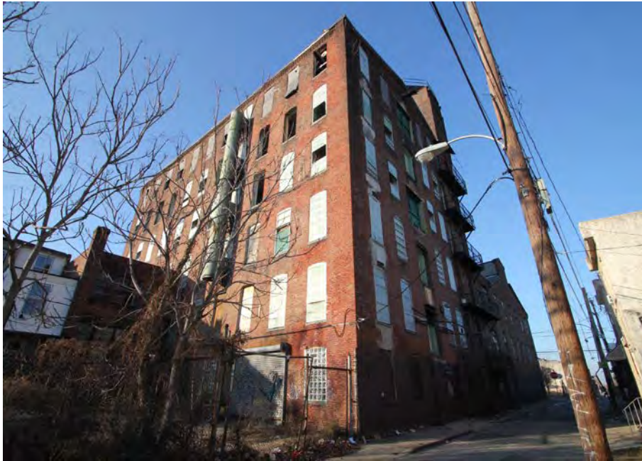
Photograph 7 – South and east elevations, Section C, view northwest
