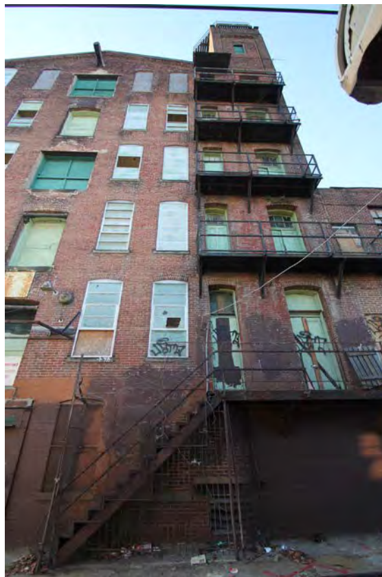
Photograph 8 – East elevation, Section C, view west
