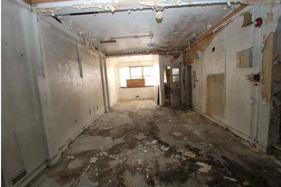
Photograph 29 – Section E, 2nd floor, view west
