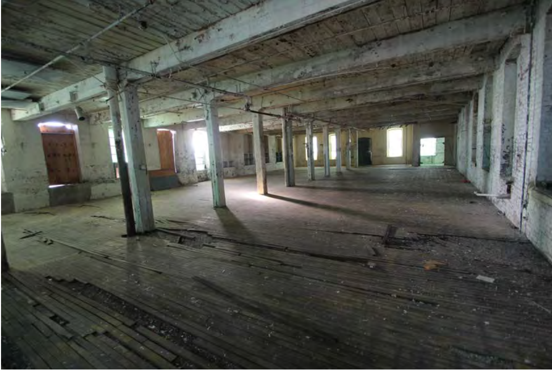
Photograph 21 – Section C, 2nd floor, view southwest
