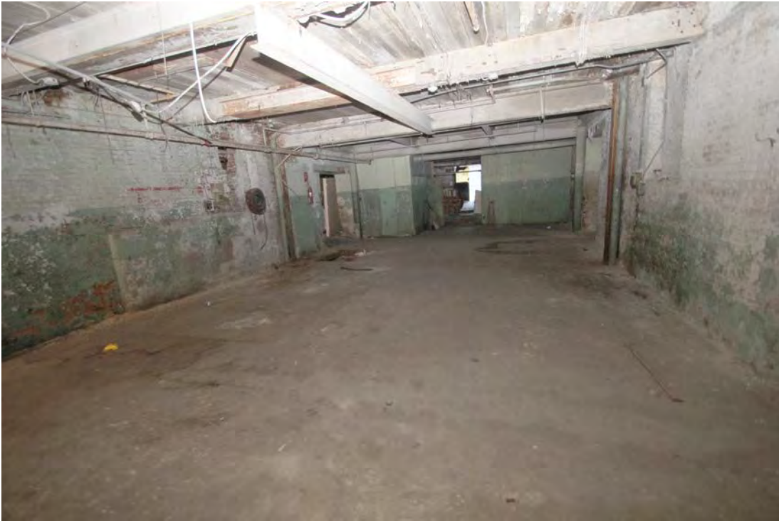
Photograph 13 – Sections B and D, Ground floor, view east
