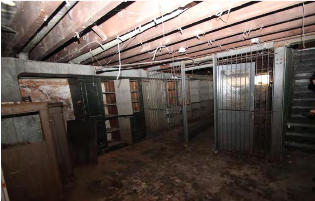
Photograph 26 – Section E, Ground floor, view southwest
