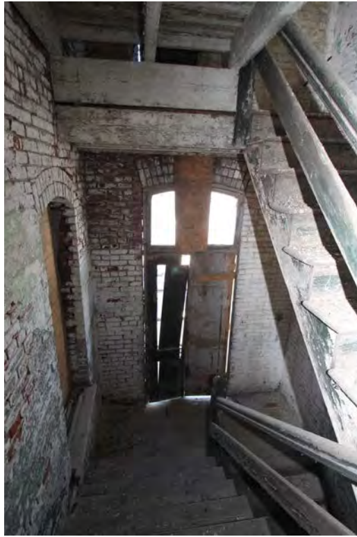
Photograph 23 – Section C, 4th floor, Stairway, view west
