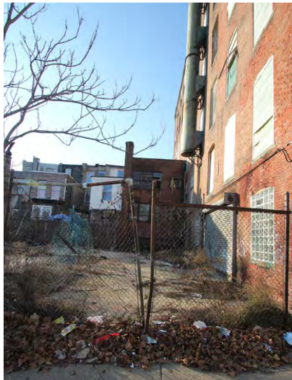
Photograph 6 – East elevation, Section E; South elevation, Section C, view west
