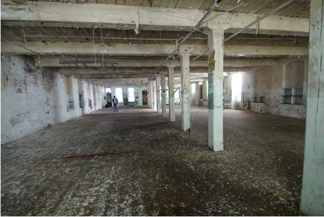
Photograph 19 – Section C, 2nd floor, view east
