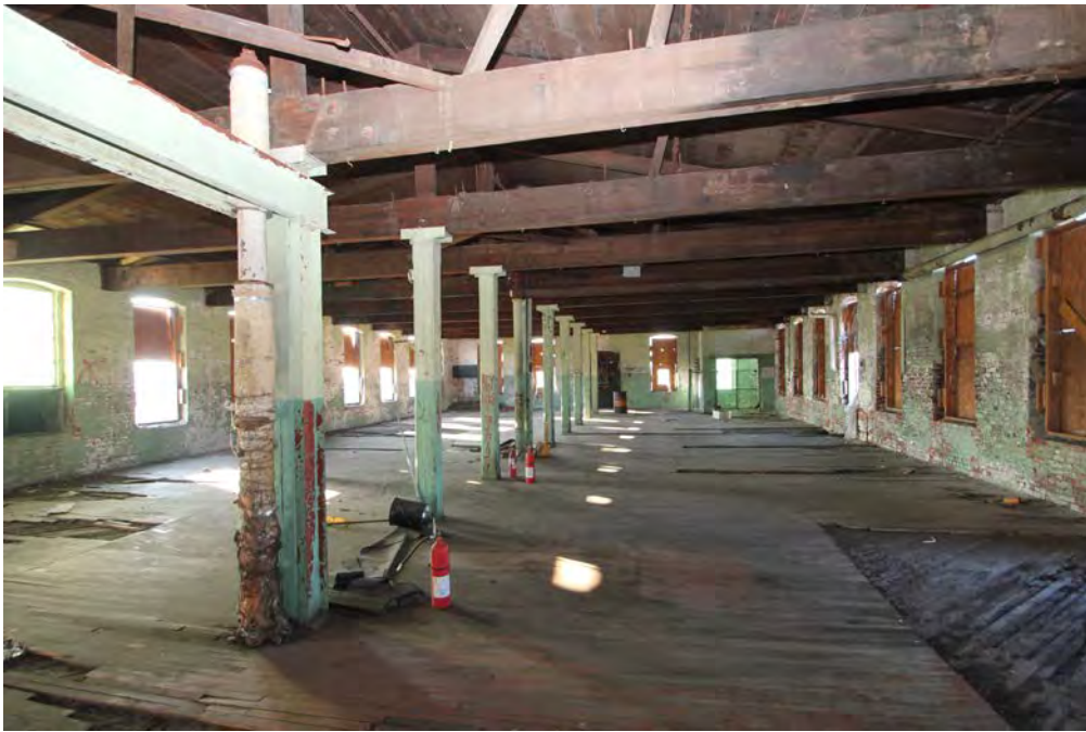
Photograph 25 – Section C, 5th floor, view west
