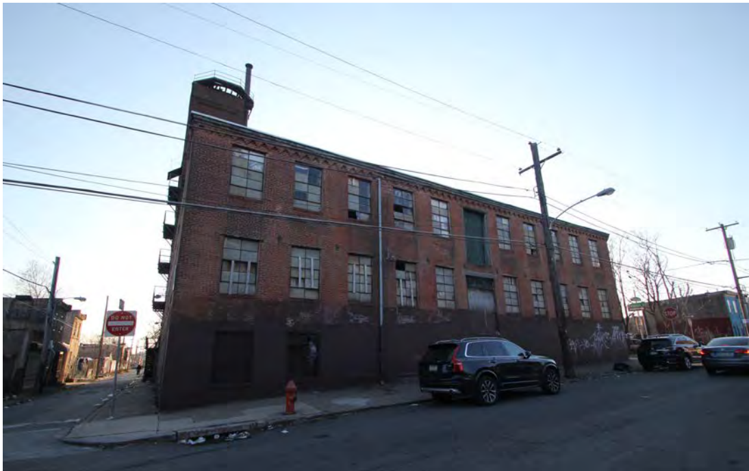
Photograph 10 – North elevation, Section A, view southwest
