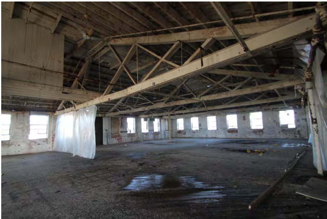
Photograph 12 – Section A, 2nd floor, view northeast
