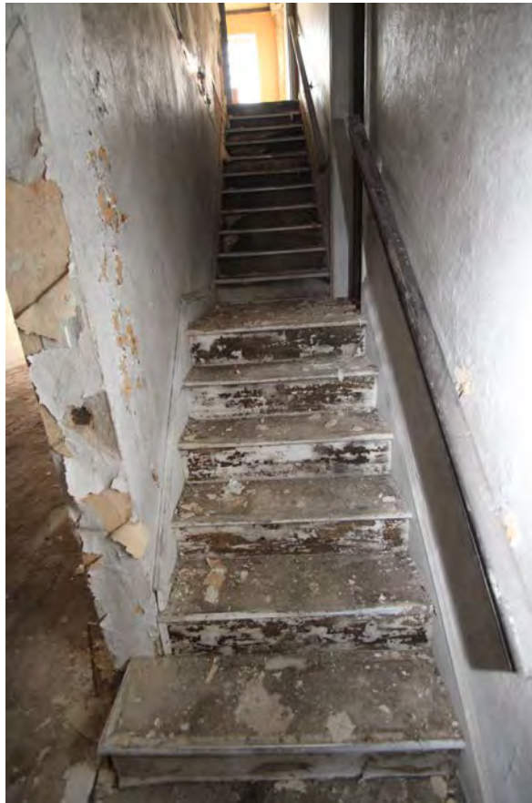
Photograph 28 – Section E, 1st floor, Stairway, view west
