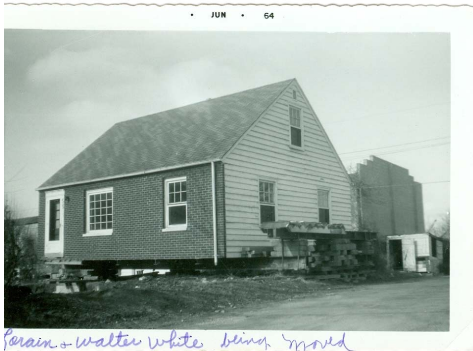
Figure 20: Carver Addition house being moved for highway construction
