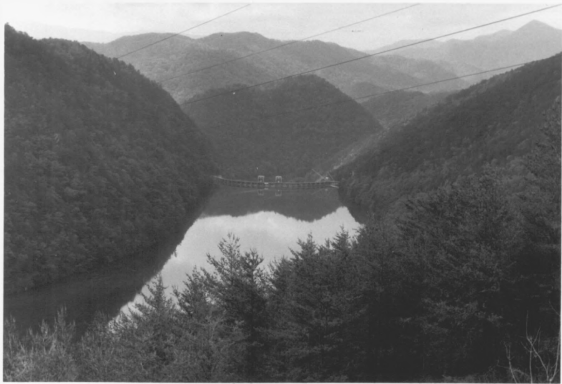
Calderwood Dam, Blount Co., TN Photo 2 of 2
