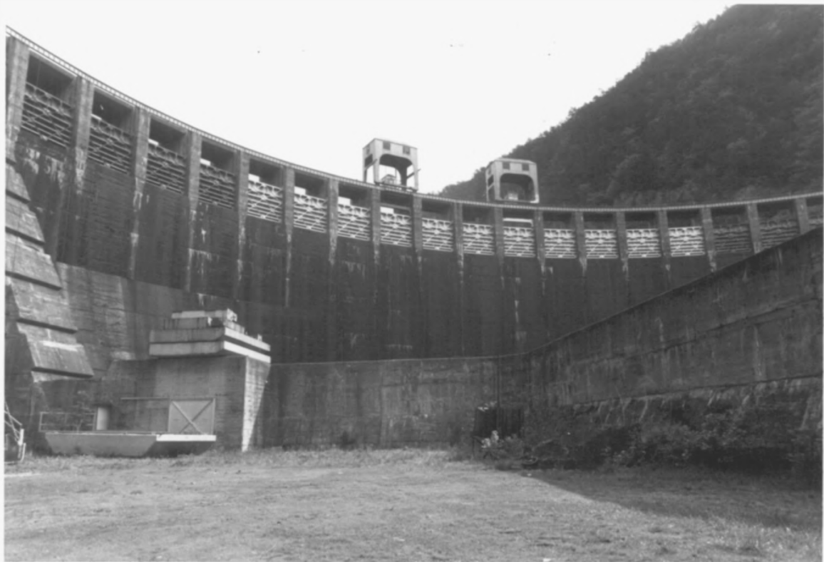
Calderwood Dam, Blount Co. TN
