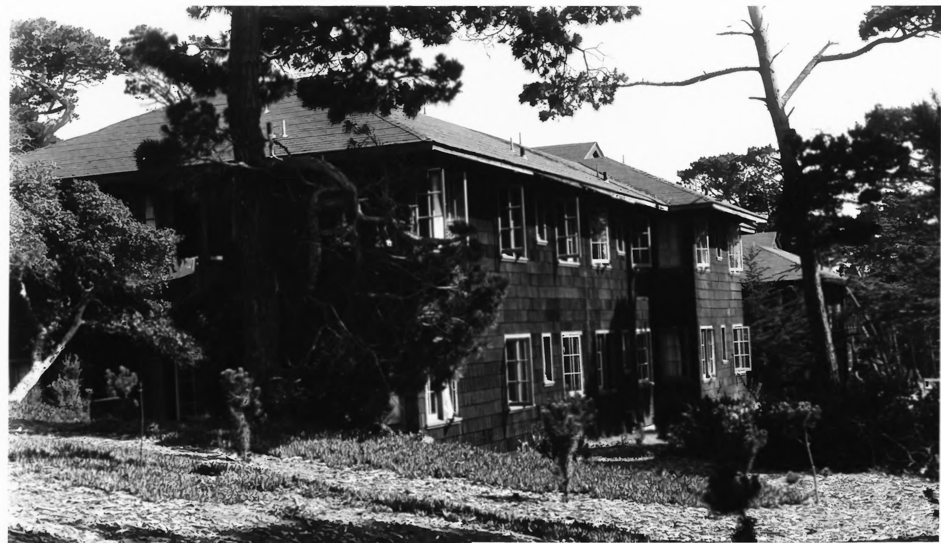
Scripps Lodge (1927-28), Asilomar Conference Grounds, west side, view toward south. (Aaron A. Gallup, California Office of Historic Preservation, 1984)
