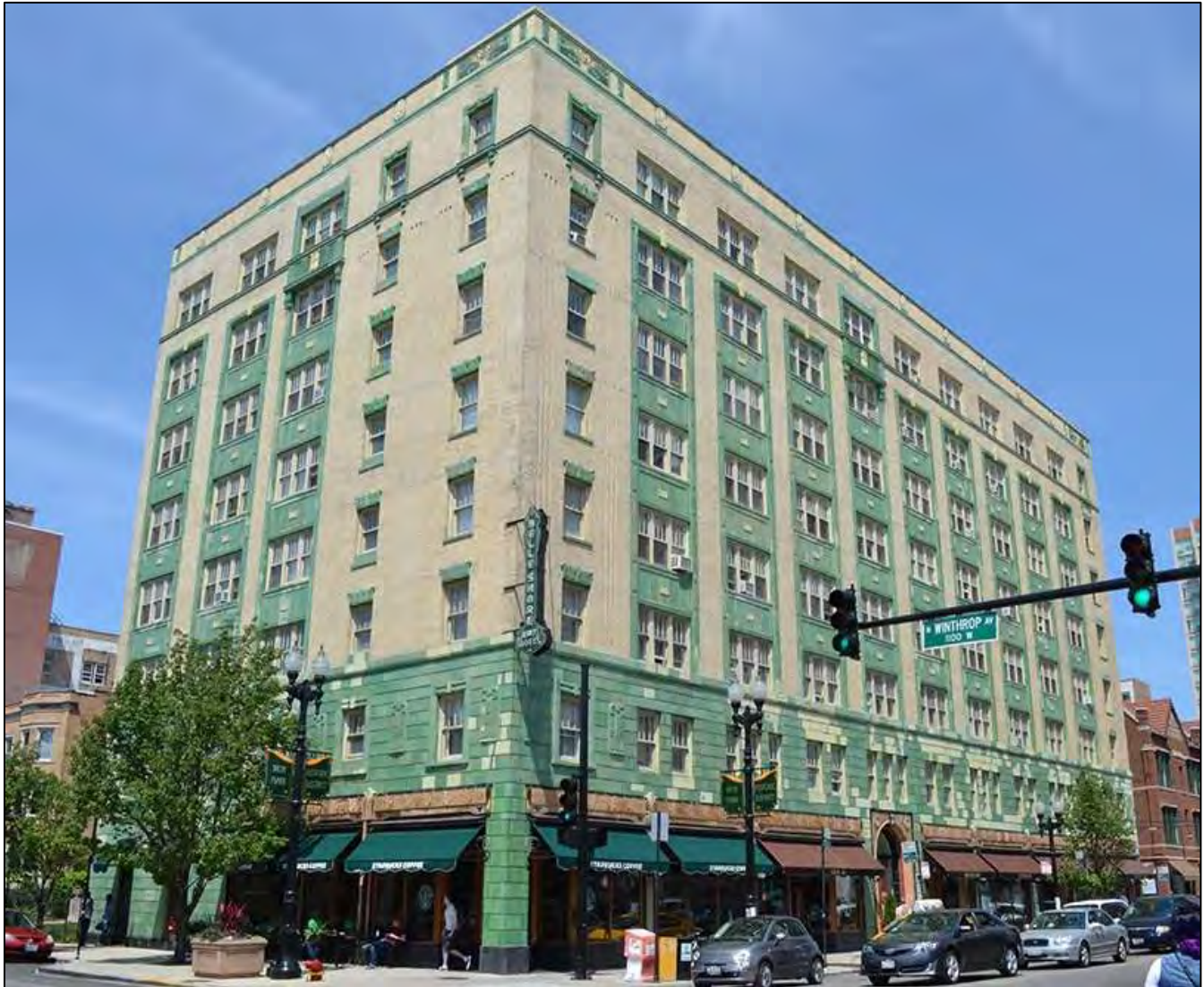
Figure 13: The Belle Shore Apartment Hotel (constructed 1929, Bryn Mawr Avenue National Register Historic District) is an example of elaborate terra-cotta ornamentation utilized for middle-income residential hotels
