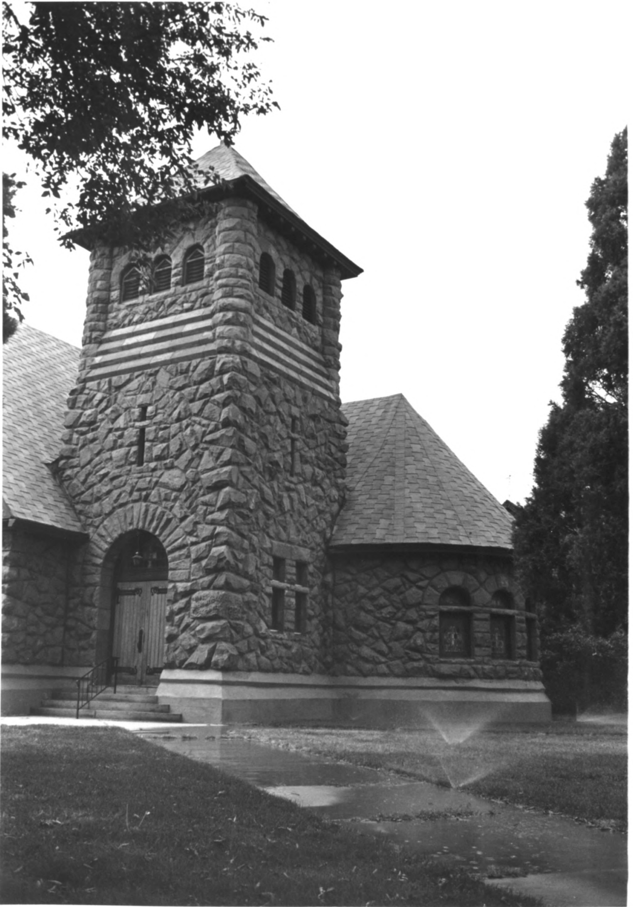
First Congregational Church - Northwest Corner
