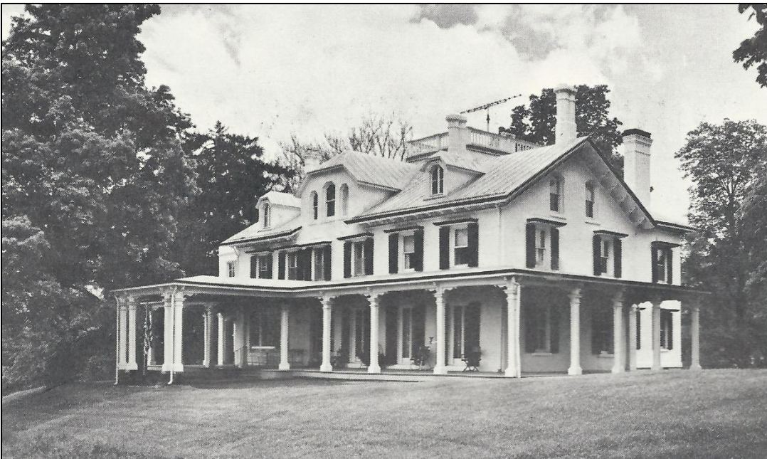
Fig.2: View of house from northeast, ca. 1926, showing metal roof, porte cochere , north piazza and new chimney in northwest corner, all added ca. 1909. From sales brochure in private collection.
