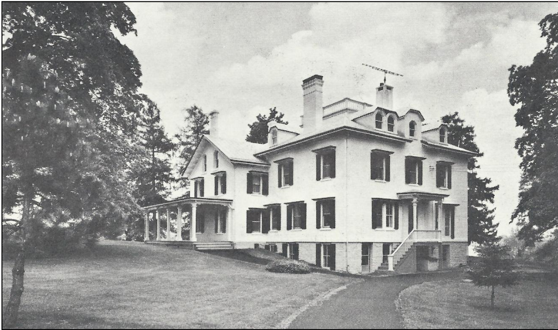
Fig.3: View of house from northwest , ca. 1926 showing north piazza and new chimneys added ca. 1909 and entrance porch with side stairs on west façade. From sales brochure in private collection.
