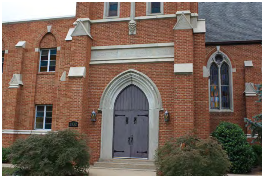
Photo 6 Main entrance, North side
