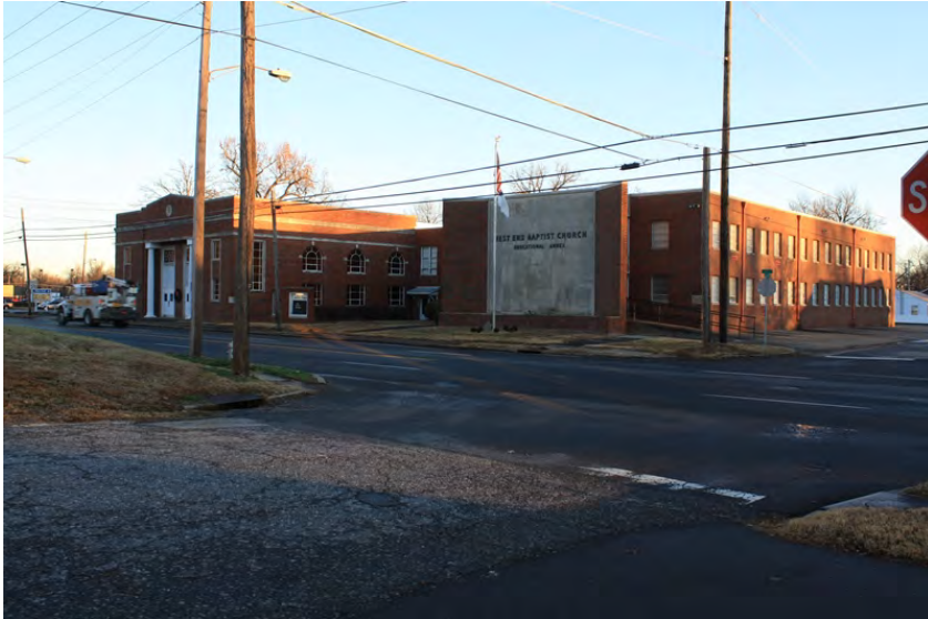
Figure 10, West End Baptist Church, Paducah
