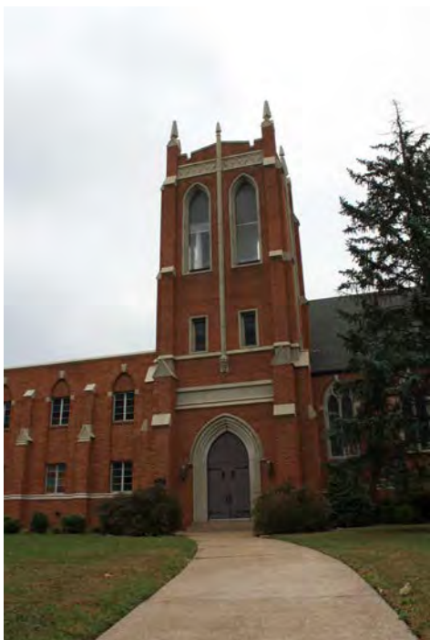
Photo 5, Main entrance, North side
