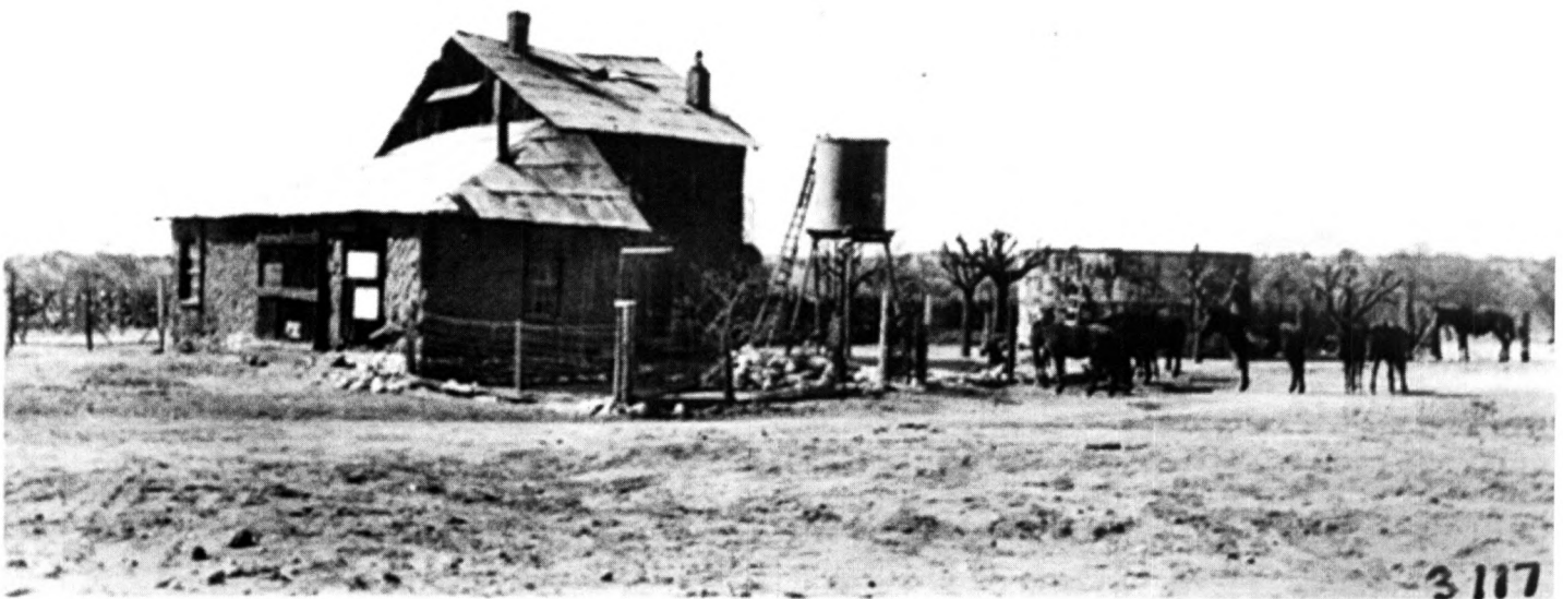
Figure 9. Steam Pump Building, 1929 (Source: Arizona Historical Society).
