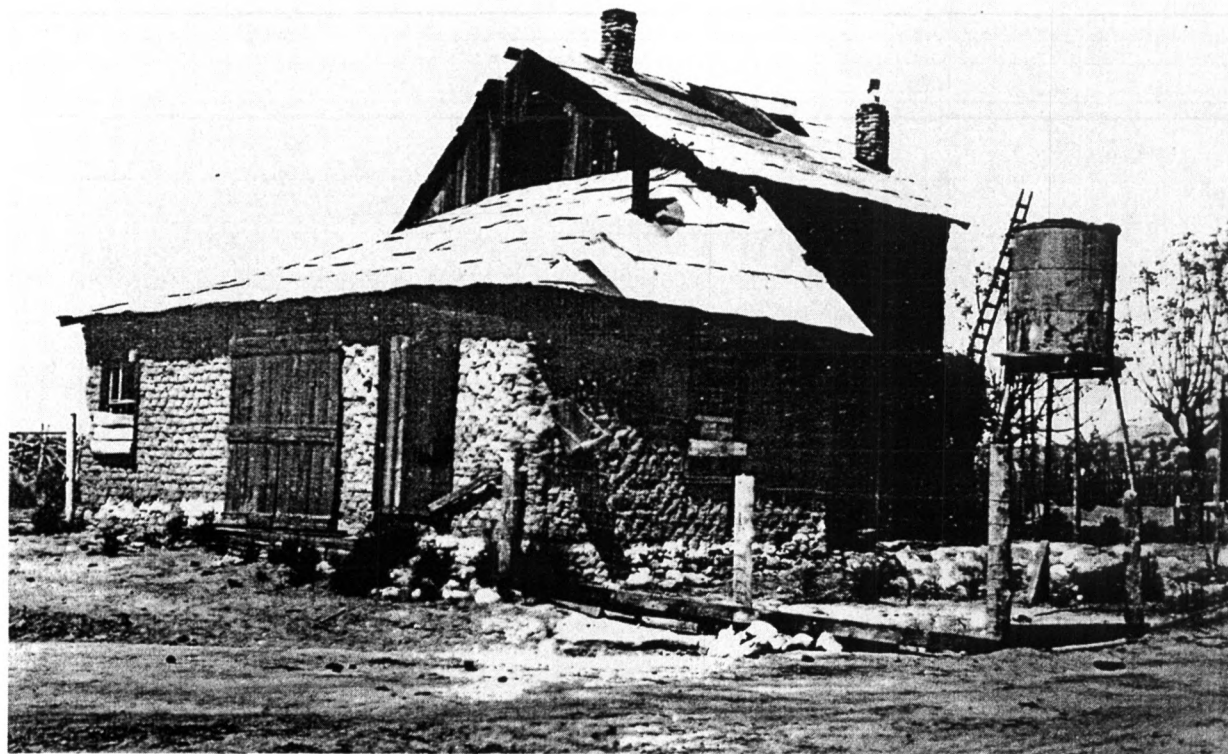
Figure 8. Steam Pump Building, 4/6/1923 (Source: Arizona Historical Society).
