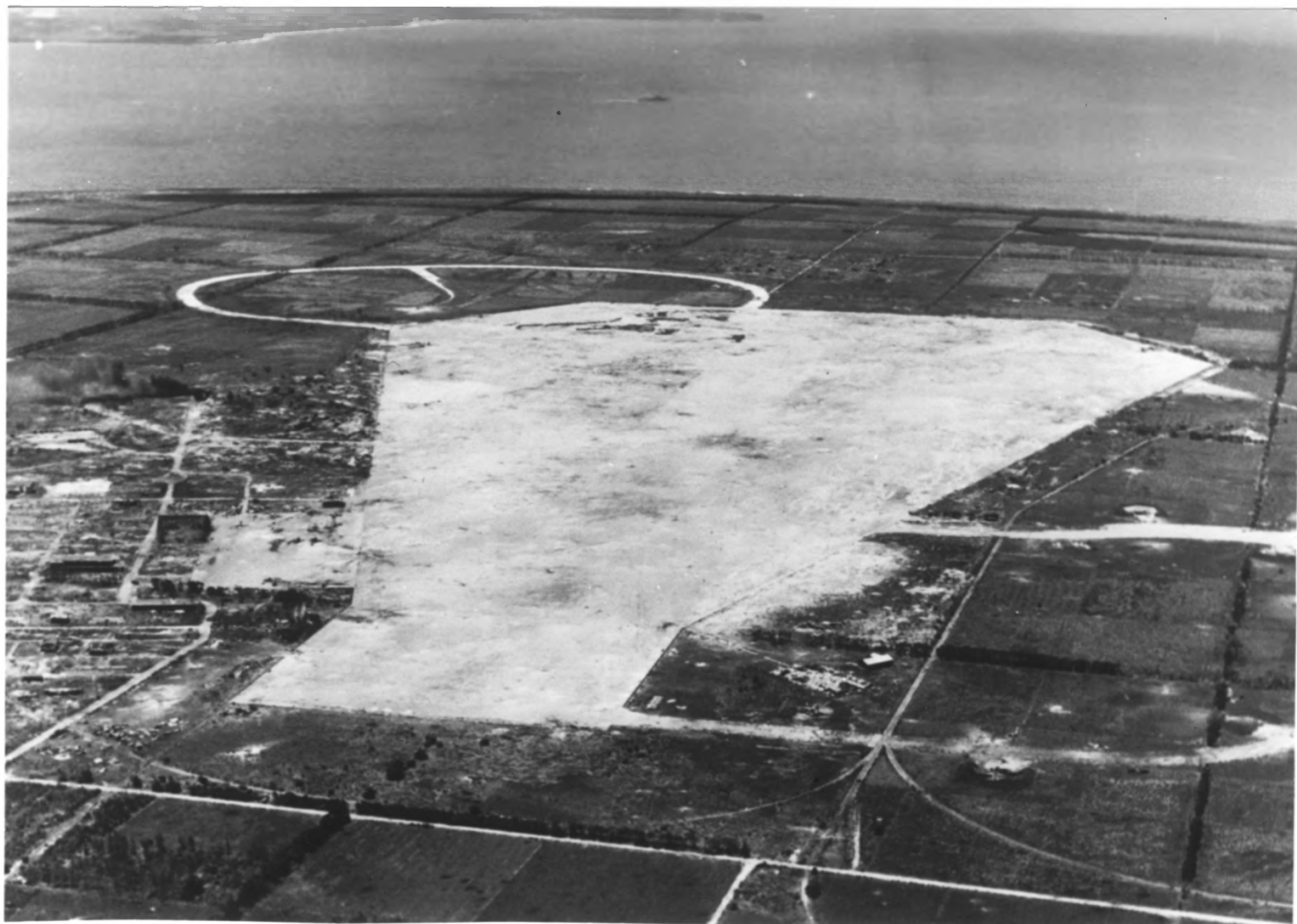
5. Aerial of Japanese Ushi Point Field at the time of the American invasion in July 1944. To the left is the existing Japanese service apron. On its upper right is the air operations building. The air administration building is in the extreme left of the photo.
