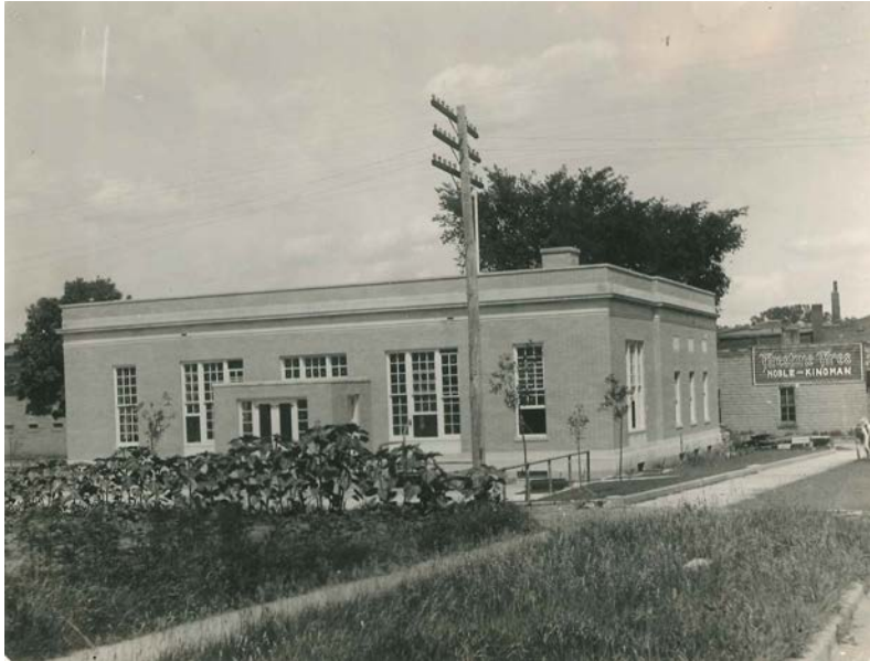
Figure 9. HISTORIC IMAGE - Looking northeast. Construction complete, 1918, Cedar Falls Historical Society.
