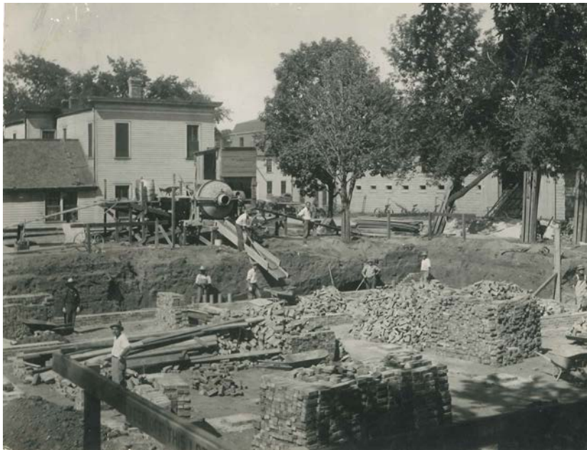
Figure 6. HISTORIC IMAGE - Basement excavation during construction, 1917, Cedar Falls Historical Society.
