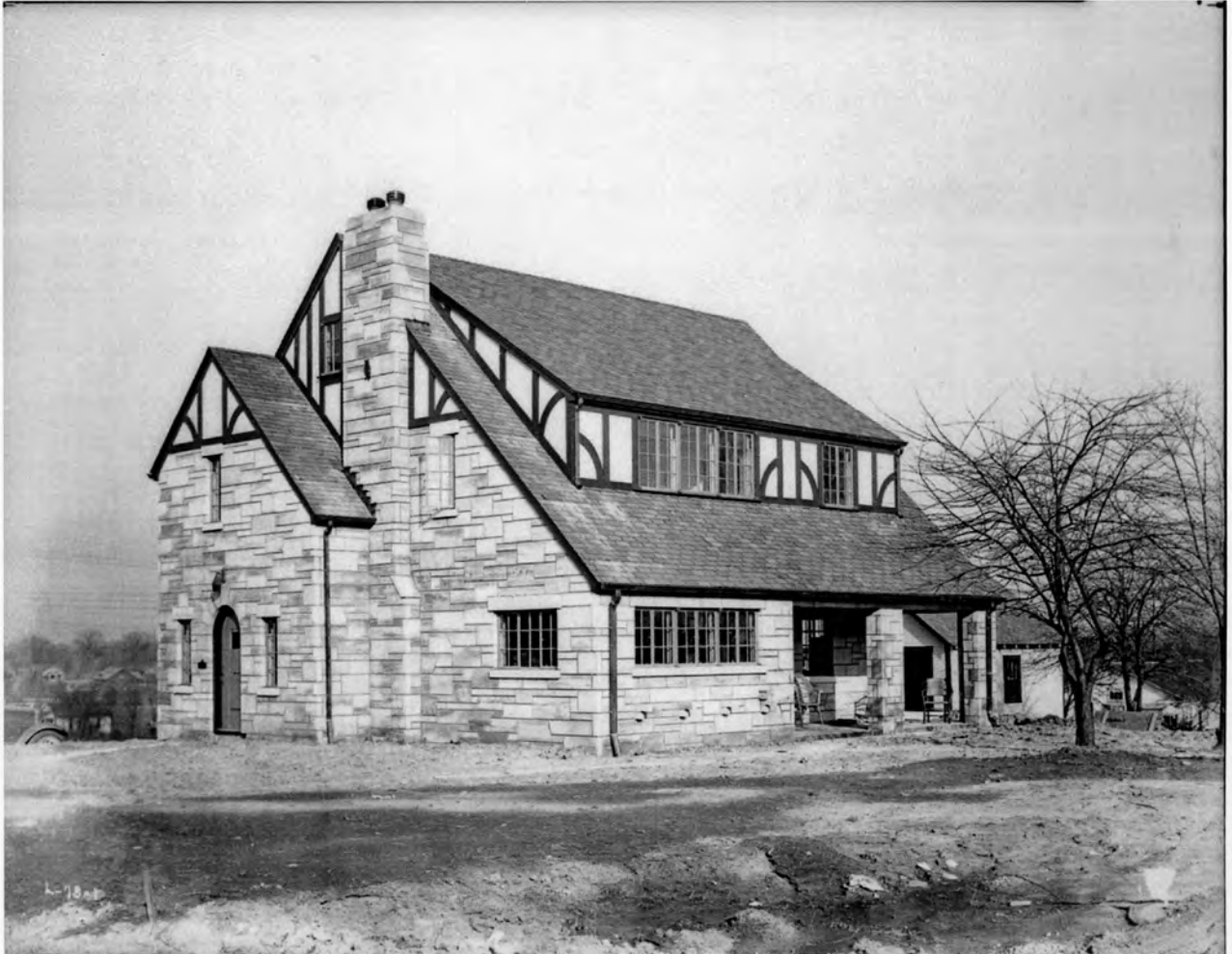
Alfred and Kathleen Evens House • 727 S. Jordan Ave. (52 c1930 camera facing northeast
