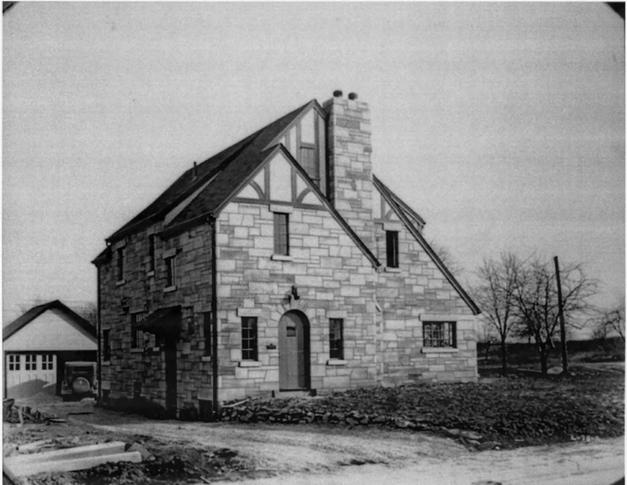
Alfred and Kathleen Evens House • 727 S. Jordan Ave. (52) c1930 camera facing southeast
