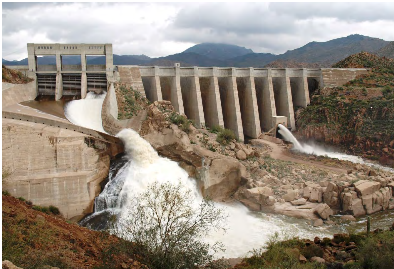
Photo 2. Bartlett Dam looking east.
