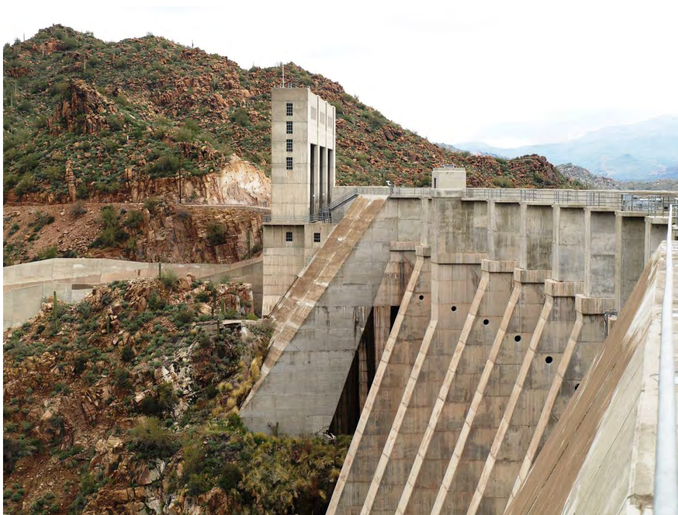
Photo 4. Bartlett Dam looking north toward gate house.
