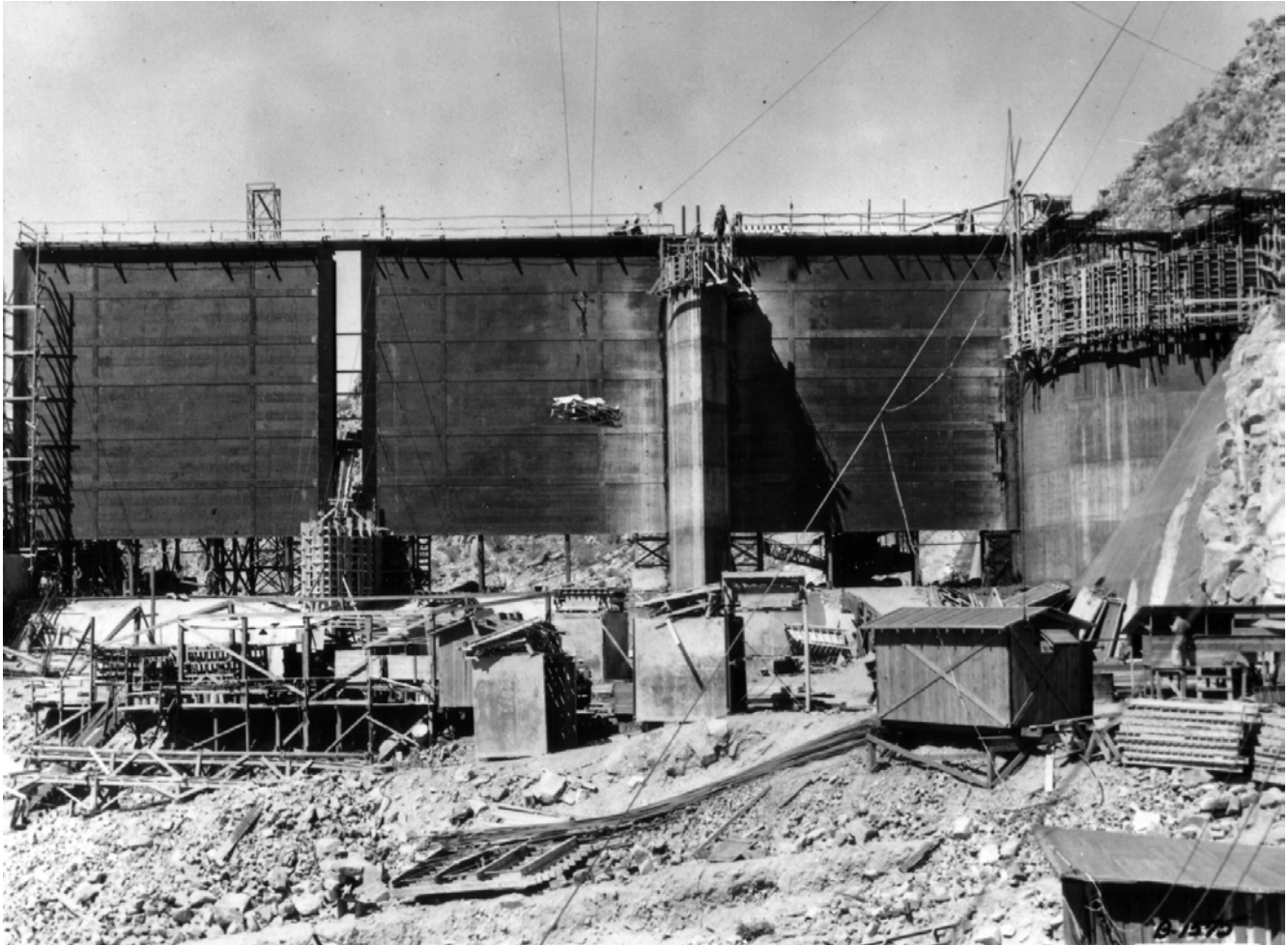
Historic Photo 7. Looking downstream toward three 50 by 50 foot spillway gates. Photo taken September 20, 1938. Photo courtesy of the SRP.
