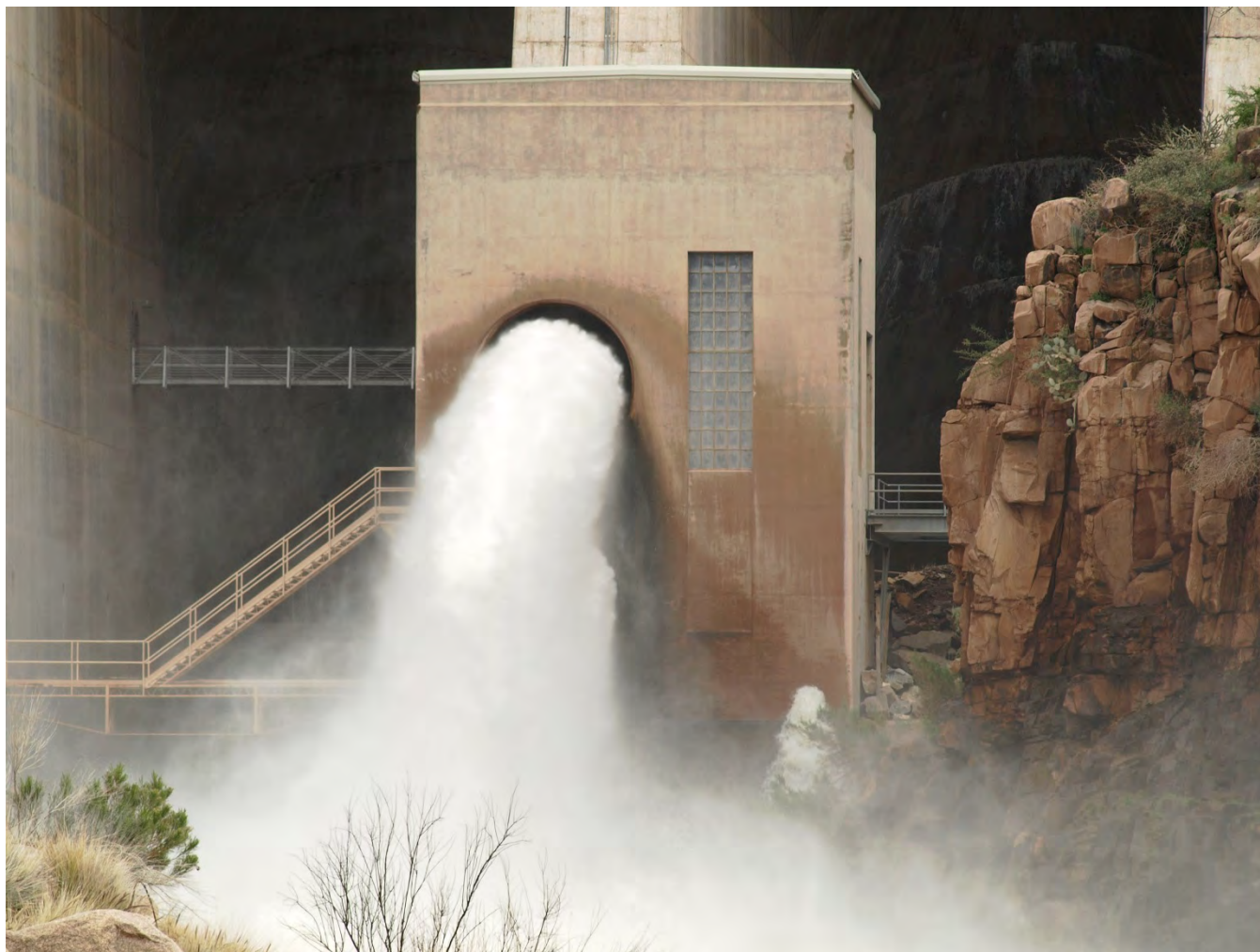
Photo 9. Bartlett Dam river outlet works looking east.
