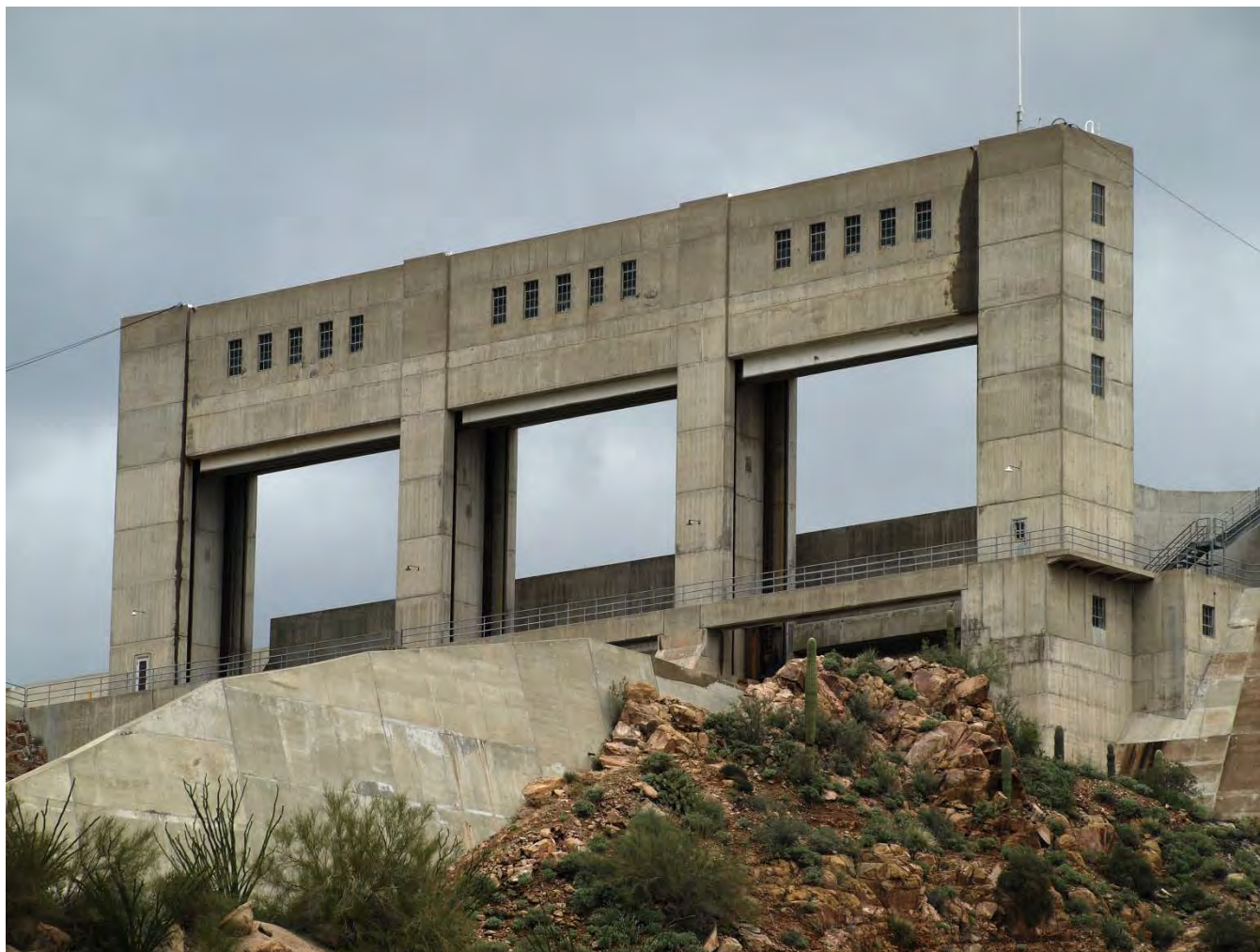
Photo 5. Bartlett spillway gate house looking northeast.
