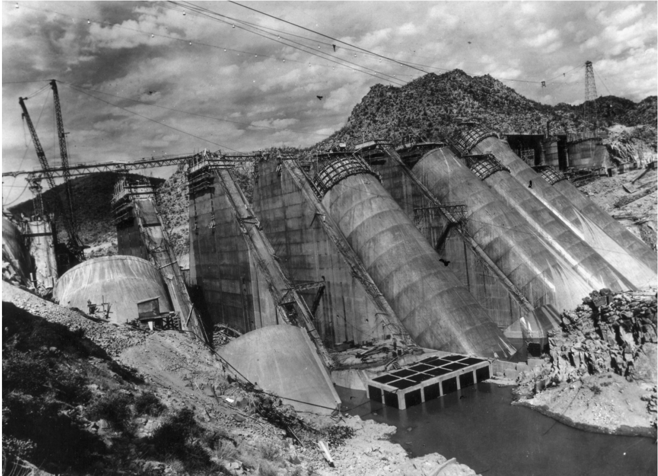
Historic Photo 8. Looking downstream toward right abutment. Crown of highest arch is within eight feet of top of dam. Photo taken September 29, 1938. Photo courtesy of the SRP.
