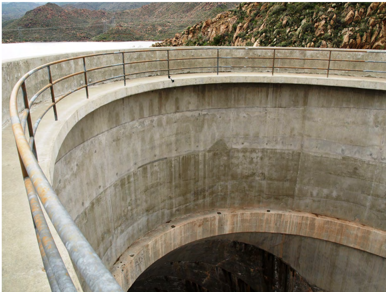
Photo 8. Bartlett Dam crest (buttress B3) detail.
