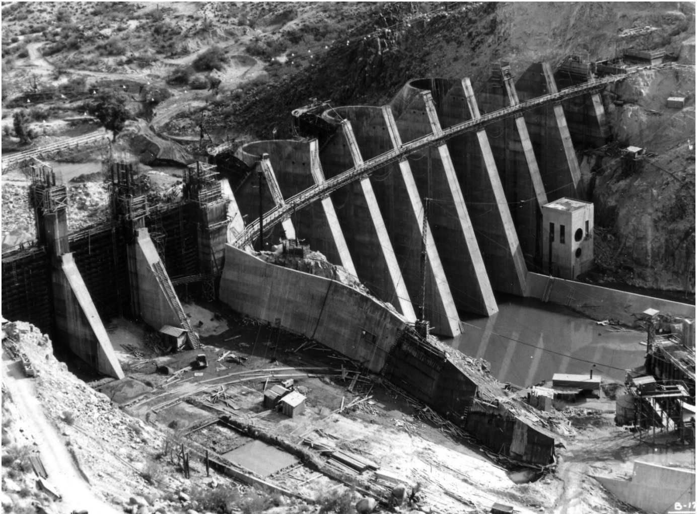
Historic Photo 10. Looking upstream toward left abutment. Note forms for left gravity abutment at upper right corner of picture. Photo taken November 29, 1938. Photo courtesy of the SRP.
