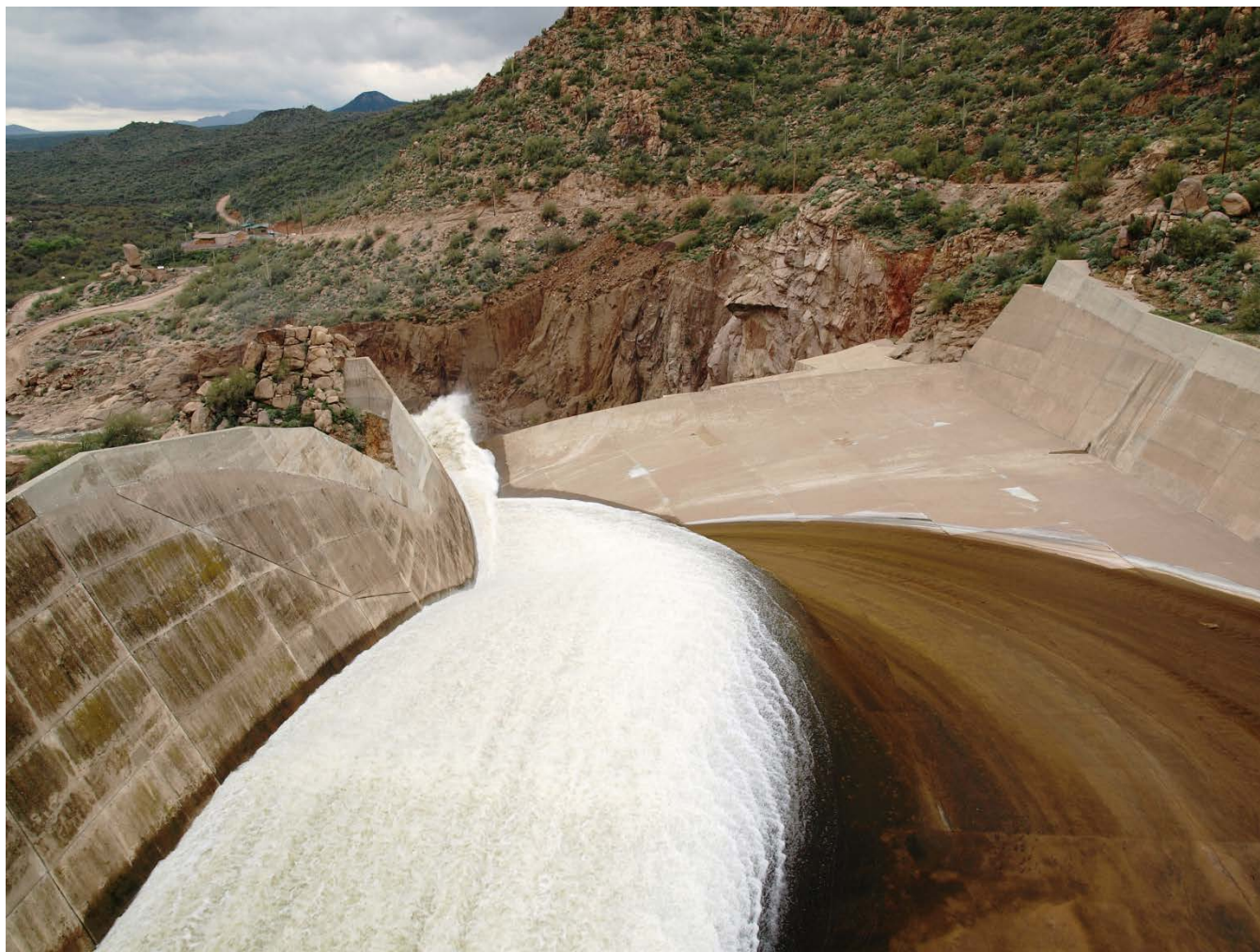
Photo 6. Bartlett spillway looking west from gate house.
