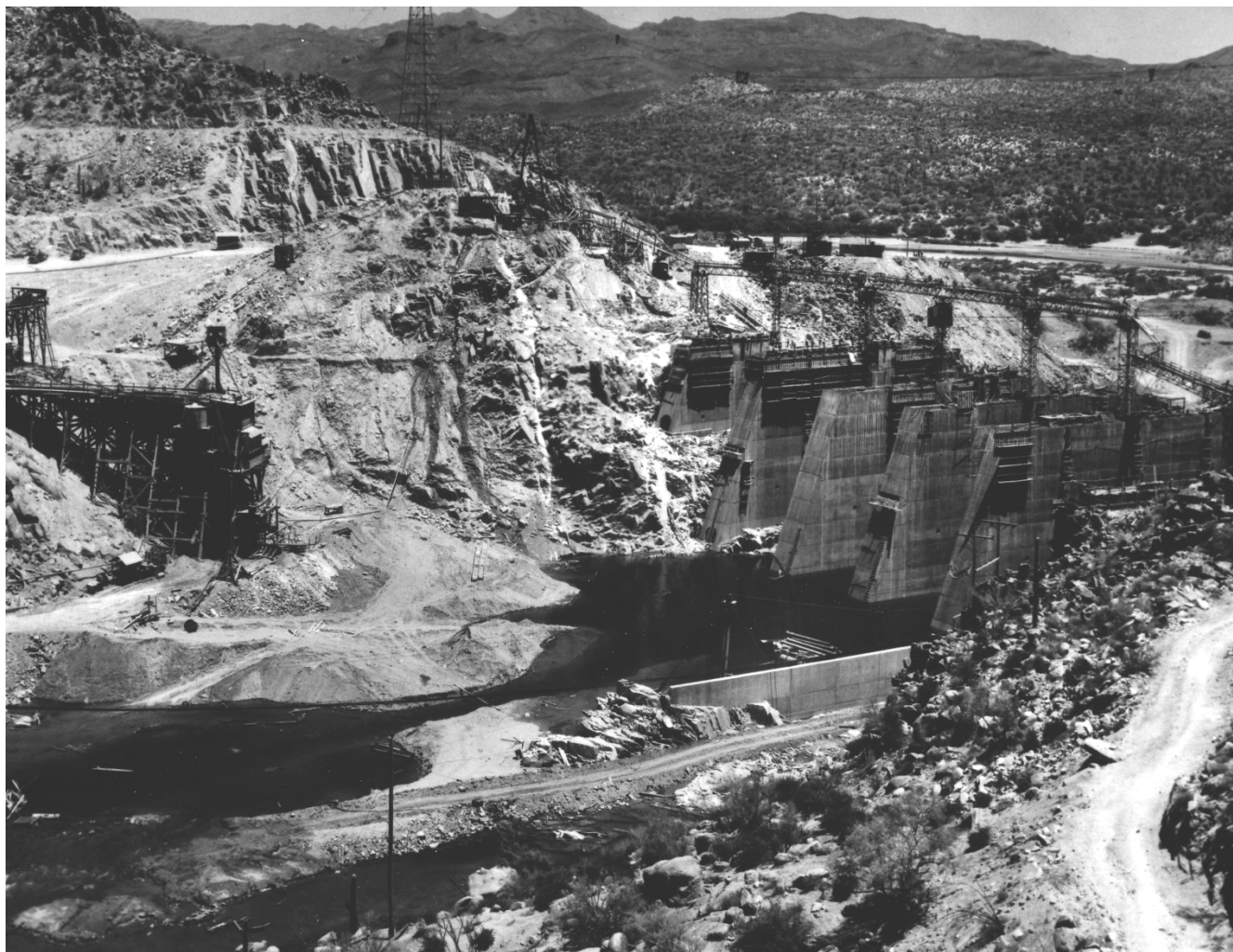
Historic Photo 3. General view looking upstream and toward right (south) abutment. Level part of trussed walkway is at elevation 1740. Buttresses 3 (on extreme left), 4, 5, 6, 7, completed to elevation 1690. Photo courtesy of the SRP.
