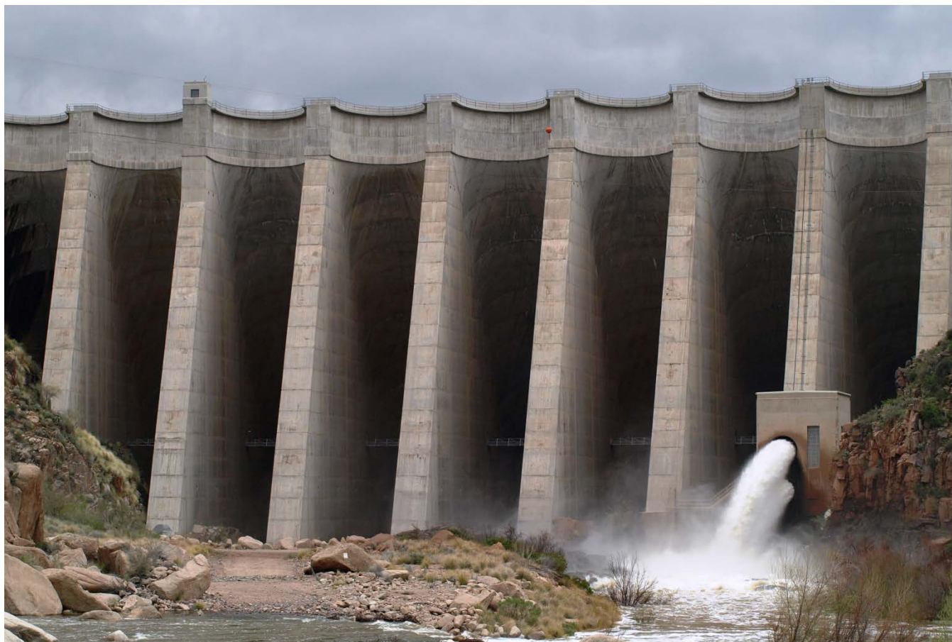
Photo 7. Bartlett Dam buttress detail looking east.
