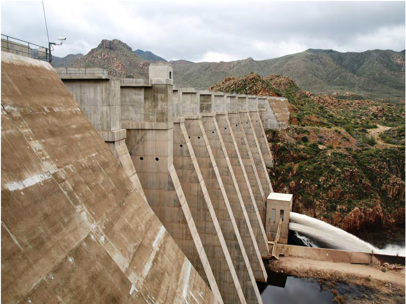
Photo 3. Bartlett Dam looking south toward left abutment.
