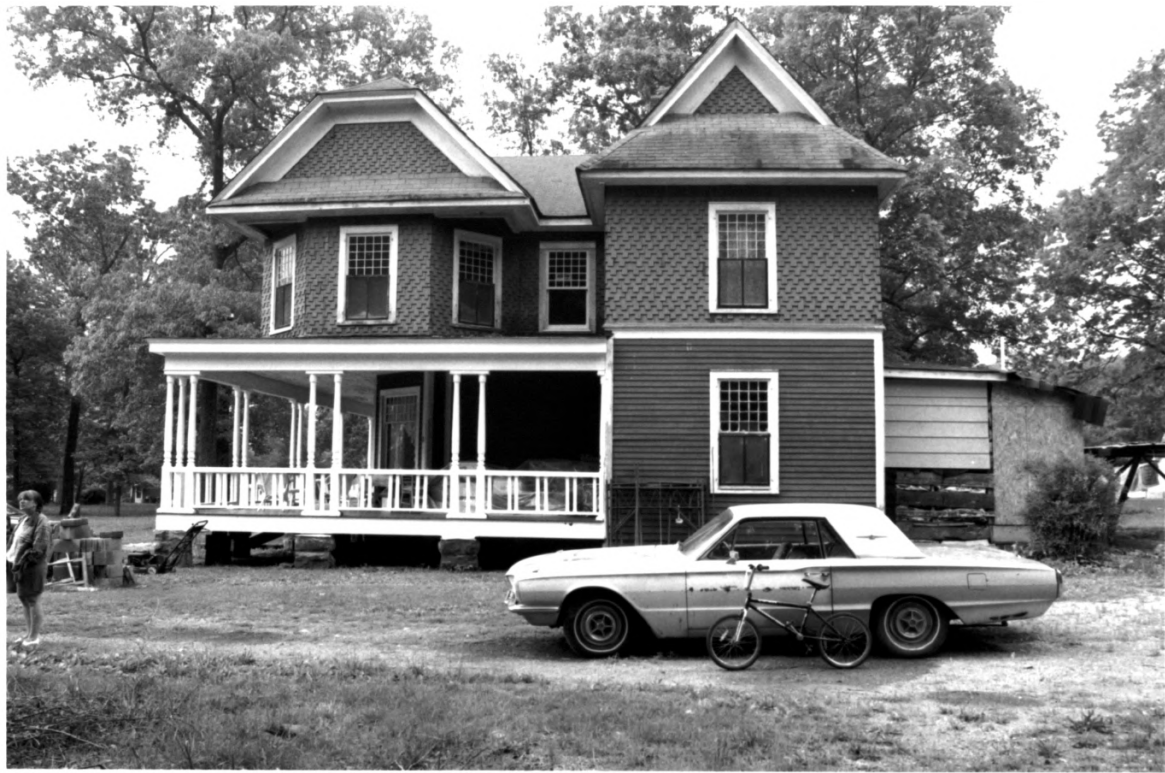
Douglas Coal and Coke Company Club house Sequatchie Co. TN
