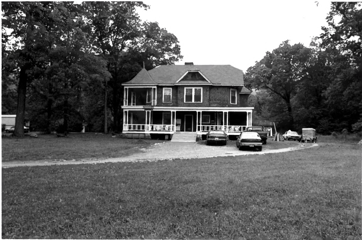
Douglas Coal and Coke Company Clubhouse Sequatchie Co. TN 1 of 24
