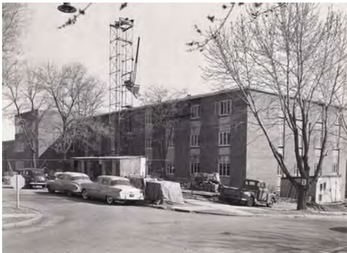
Figure 2: Nurses' Home addition under construction, 1954 (Alegent Health Immanuel Medical Center, memories.nebraska.gov)
