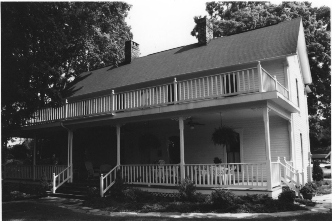
Broyles - Darwin House Rhea Co. TN
