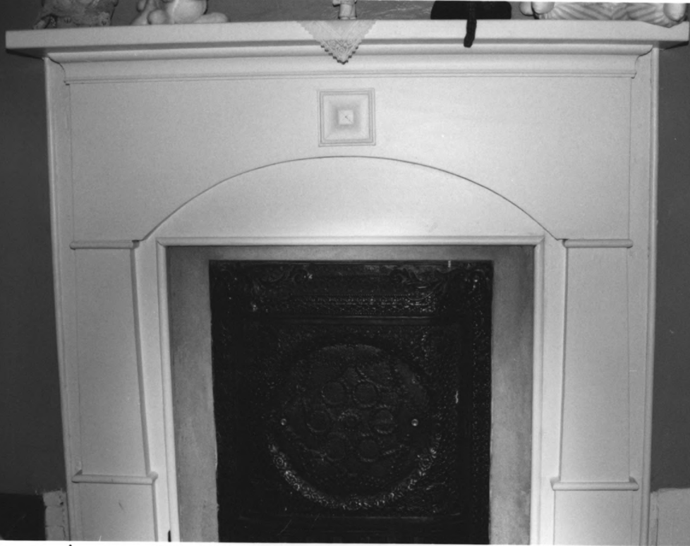
Broyles-Darwin House Rhea Co. TN
