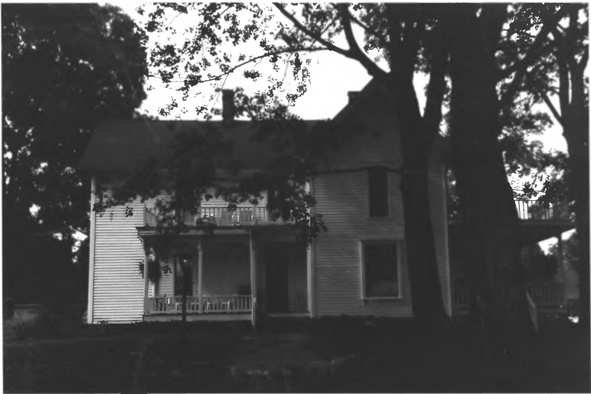
Broyles-Darwin House Rhea Co. TN
