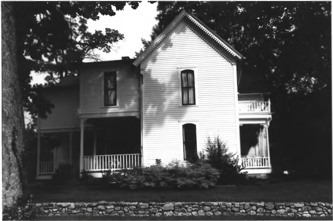
Broyles-Darwin House Rhea Co. TN
