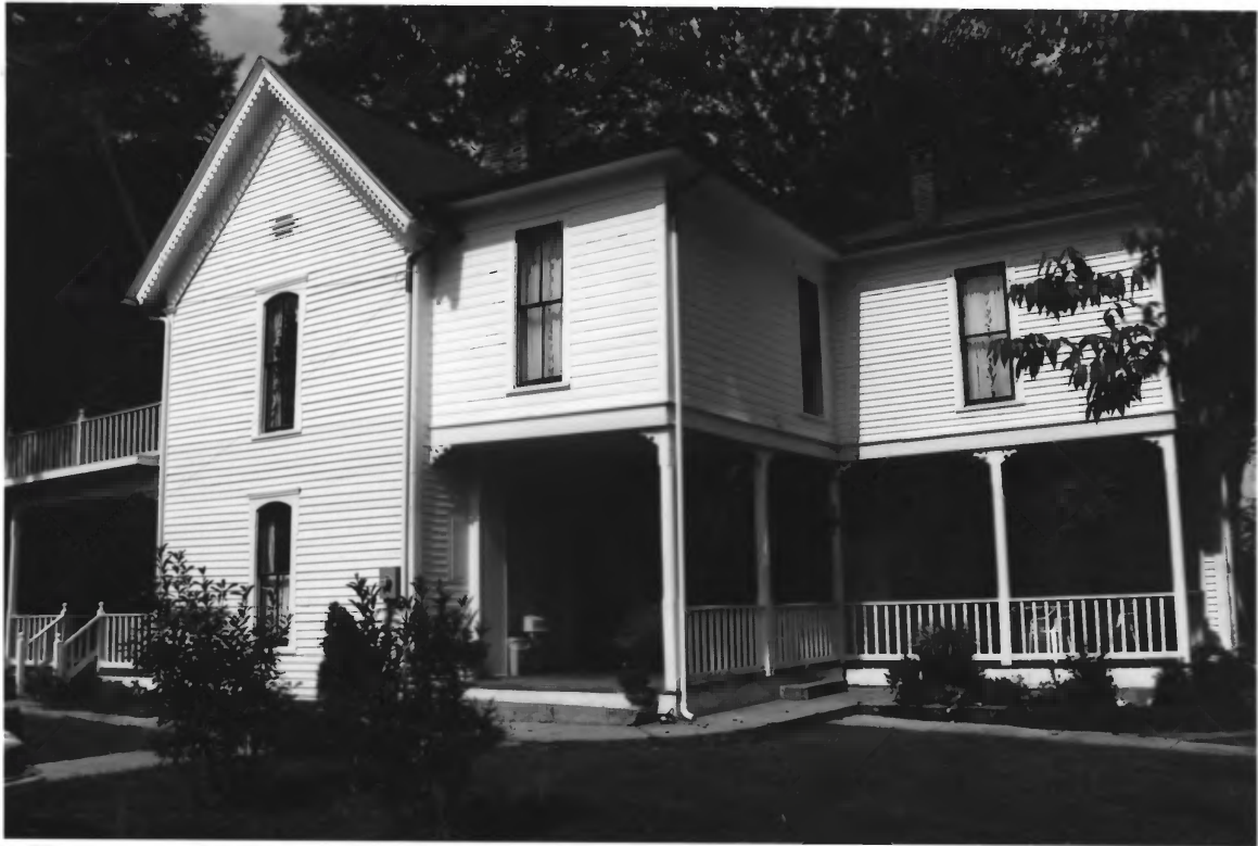
Broyles - Darwin House Rhea Co. TN
