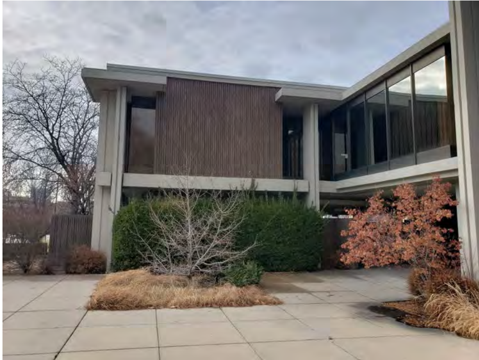
South elevation of Steiner American Building. Camera facing north.
