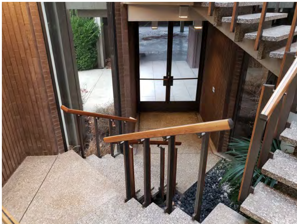
Photograph 25 of 29 Stairs of Steiner American Building. Camera facing west.
