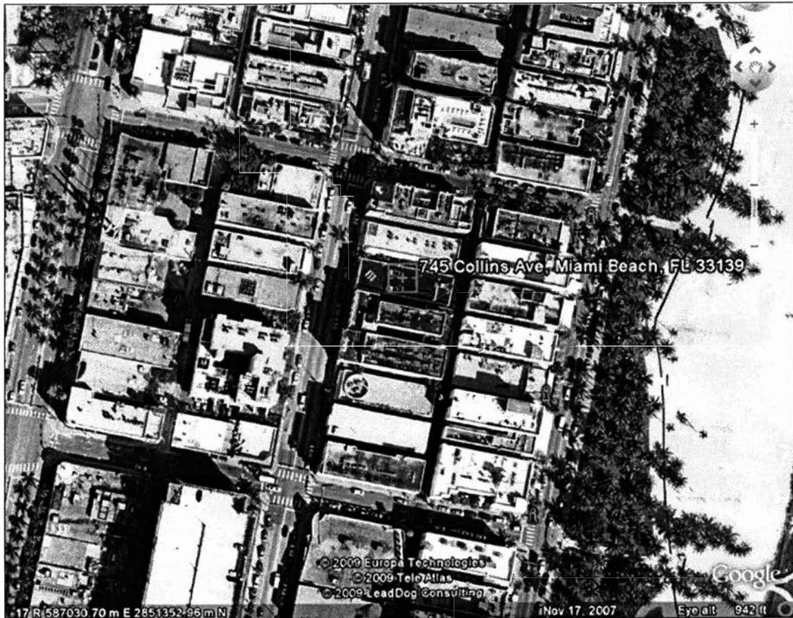
Aerial View: Former Premier Hotel, 745 Collins Avenue, Miami Beach Florida
