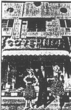
UNPROTECTED: The Governor is one of nine buildings preservationists want saved.
