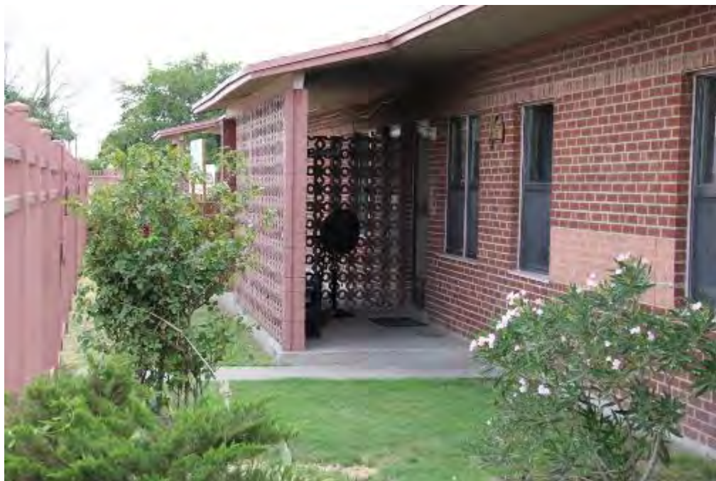
Photograph 5 – Entry facade of Apartment Building Type B. Camera facing northeast. (June 29, 2016)
