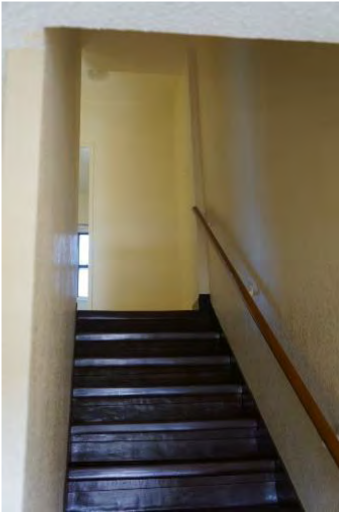
Photograph 23 – Interior view of a typical two-story apartment with stairwell at entry. (March 1, 2016)
