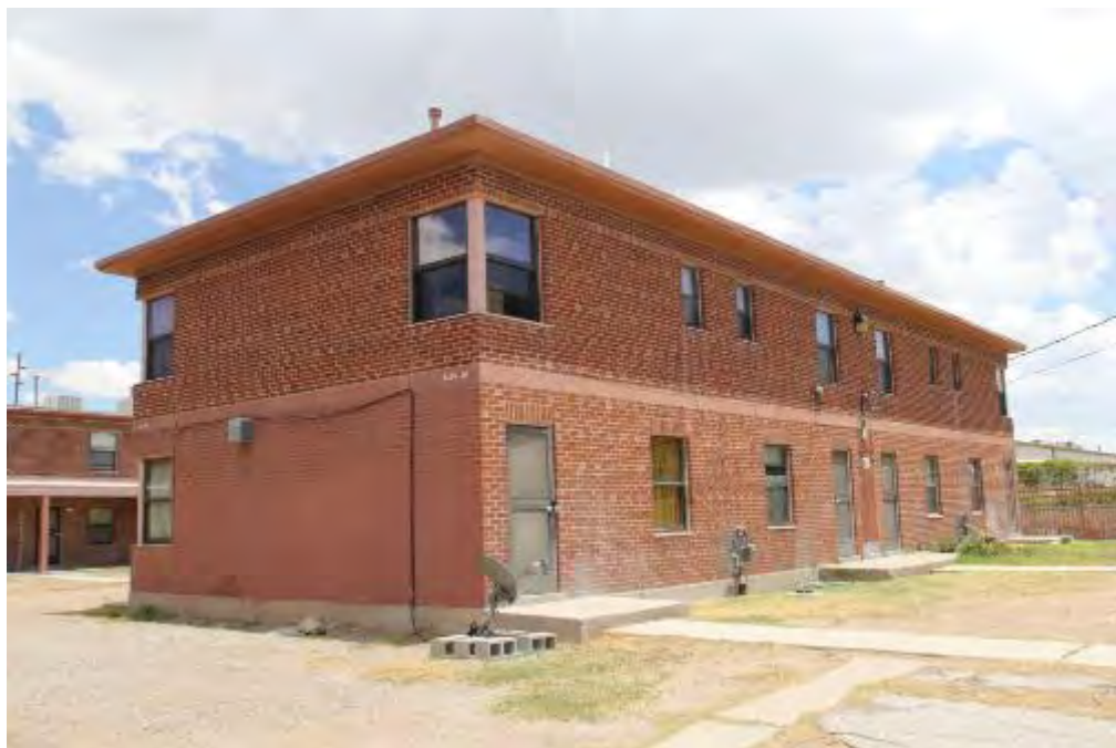
Photograph 8 – Rear façade of Apartment Building Type C. Camera facing east. (June 29, 2016)
