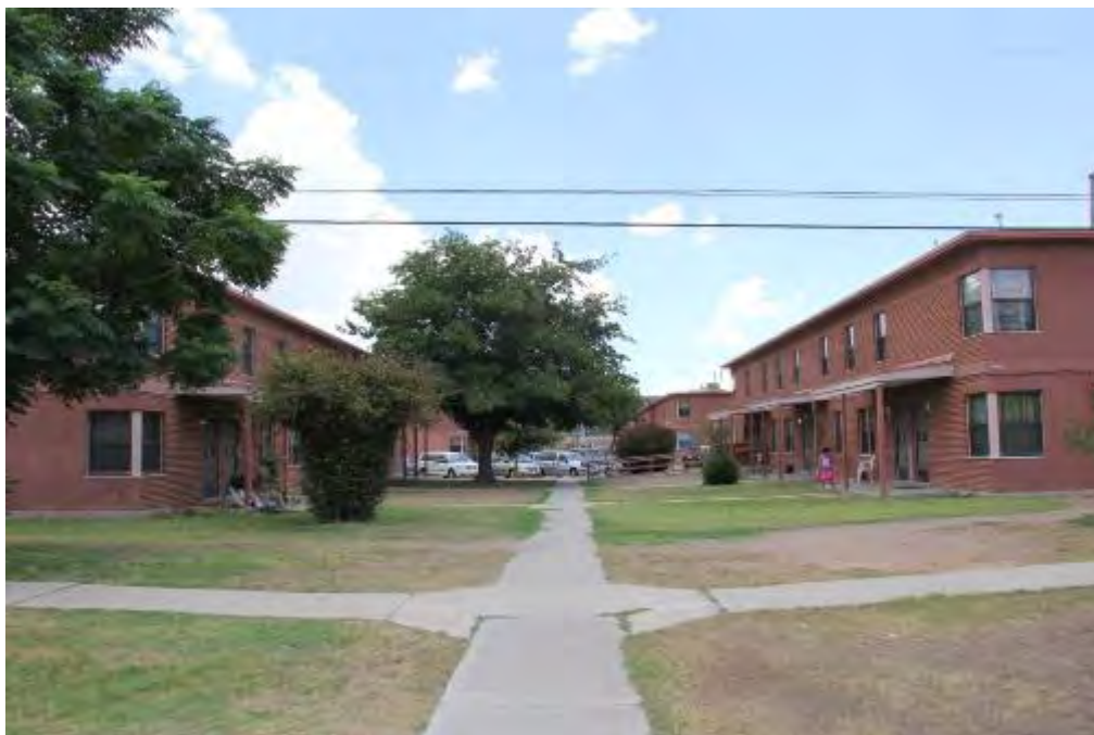
Photograph 14 – Concrete sidewalk with octagonal design. Camera facing southeast. (June 29, 2016)
