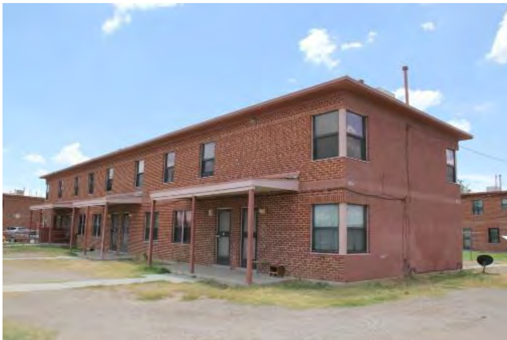
Photograph 1 – Entry facade of Apartment Building Type A. Camera facing south. (June 29, 2016)
