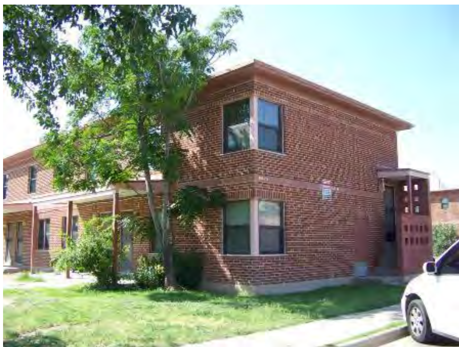
Photograph 3 – Enlarged photo of Apartment Building Type A and A1. Camera facing north. (September 2, 2015)
