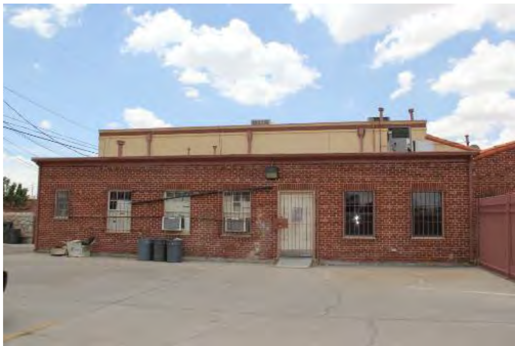
Photograph 18 – East façade of Community Activity Center (left side). Camera facing southwest. (June 29, 2016)
