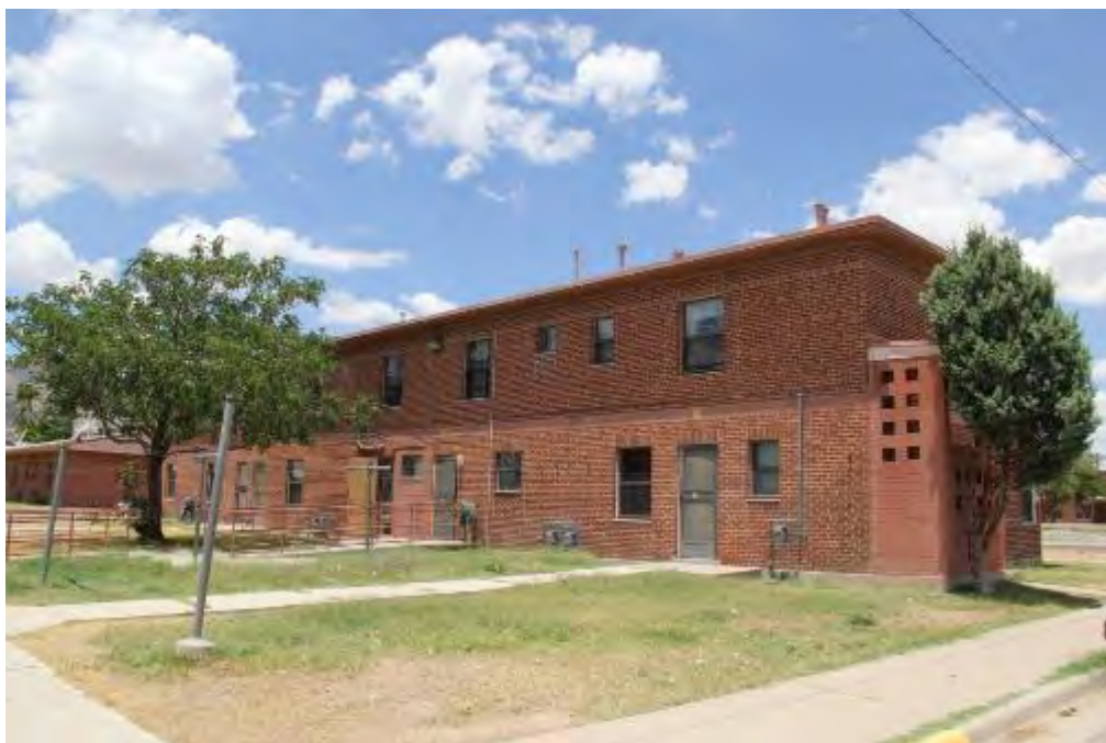
Photograph 2 – Rear facade of Apartment Building Type A1. Camera facing north. (June 29, 2016)
