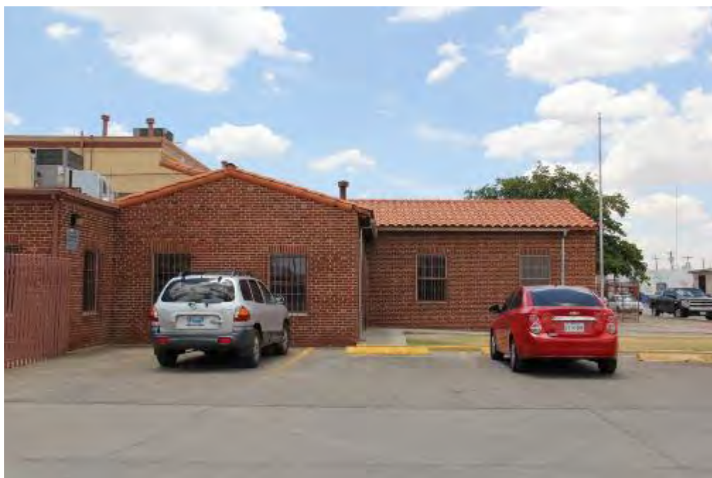
Photograph 17 – East facade of Community Activity Center (right side). Camera facing southwest. (June 29, 2016)
