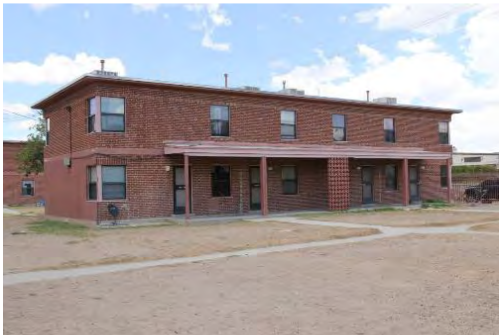
Photograph 7 – Entry façade of Apartment Building C. Camera facing east. (June 29, 2016)
