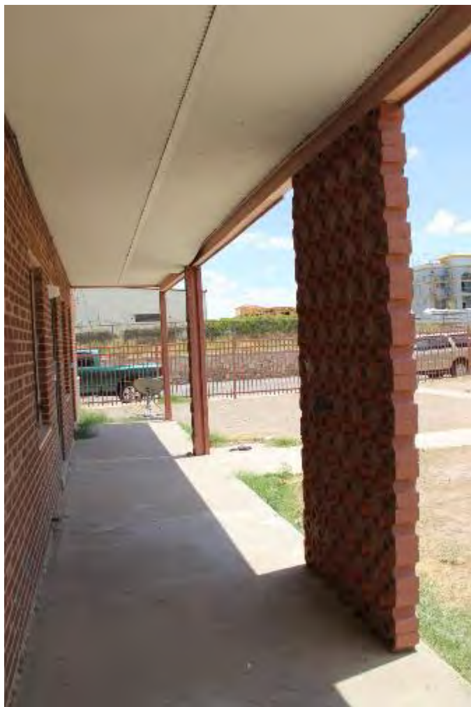
Photograph 9 – Porch view with decorative concrete block screen wall of Apartment Building Type C. Camera facing southeast. (June 29, 2016)
