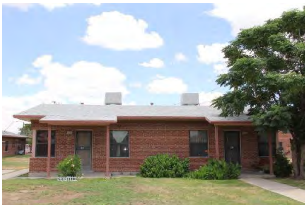
Photograph 11 – Entry façade Apartment Building Type D. Camera facing southwest. (June 29, 2016)
