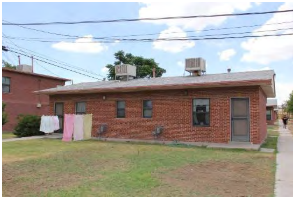
Photograph 12 – Rear facade of Apartment Building Type D. Camera facing northeast. (June 29, 2016)
