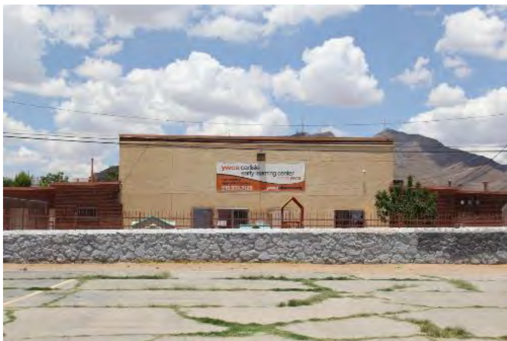
Photograph 19 – South facade of Community Activity Center. Camera facing northwest. (June 29, 2016)
