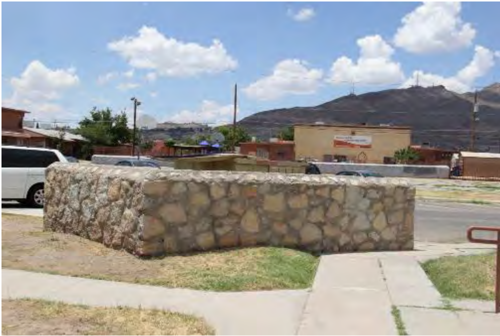
Photograph 24 – Non-contributing native stone dumpster enclosure. Camera facing north. (June 29, 2016)
