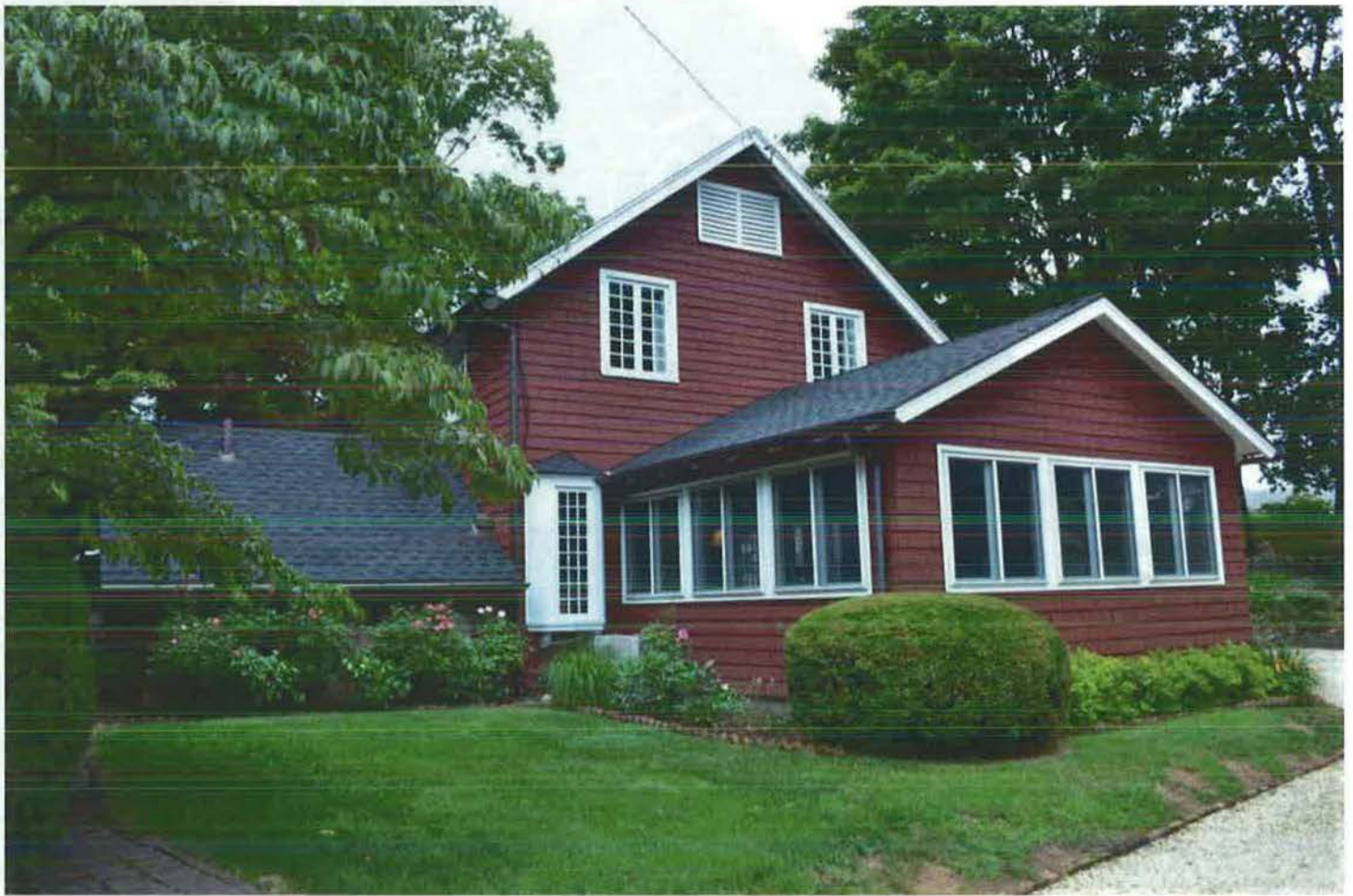
West (front) and north (side) elevations of 8 Weathervane Lane, 1874, showing elevation, roof, and window details. Camera facing east. Photograph 9 of 22.
