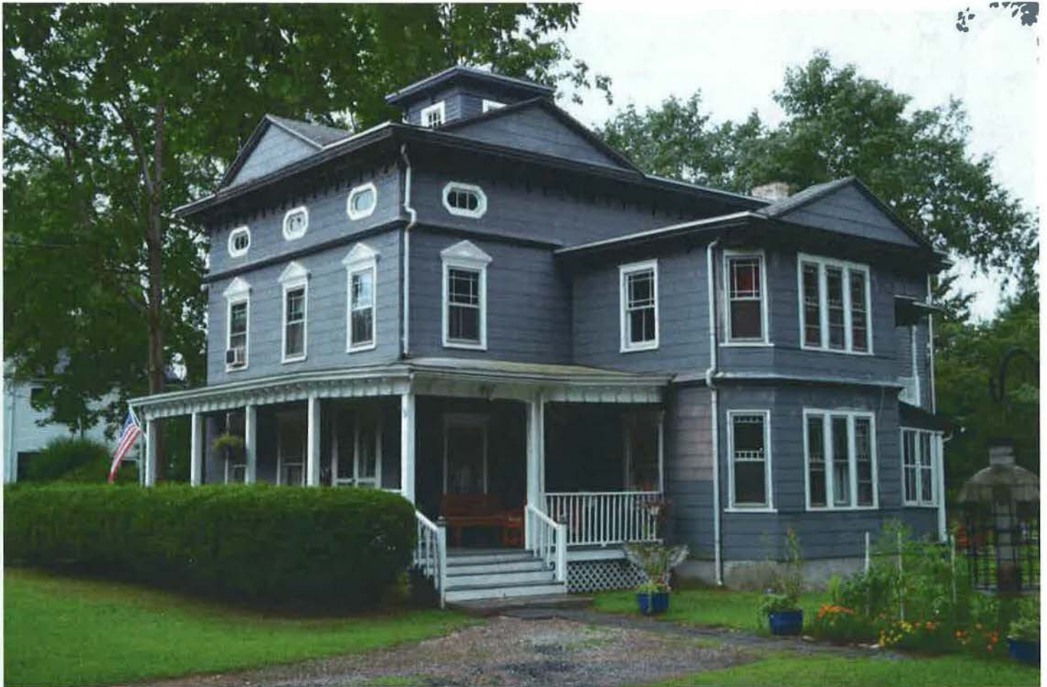
East (front) and north (side) elevations of 29 Mead Avenue, 1862, showing façade, porch, roof, and window details. Camera facing southwest. Photograph 10 of 22.
