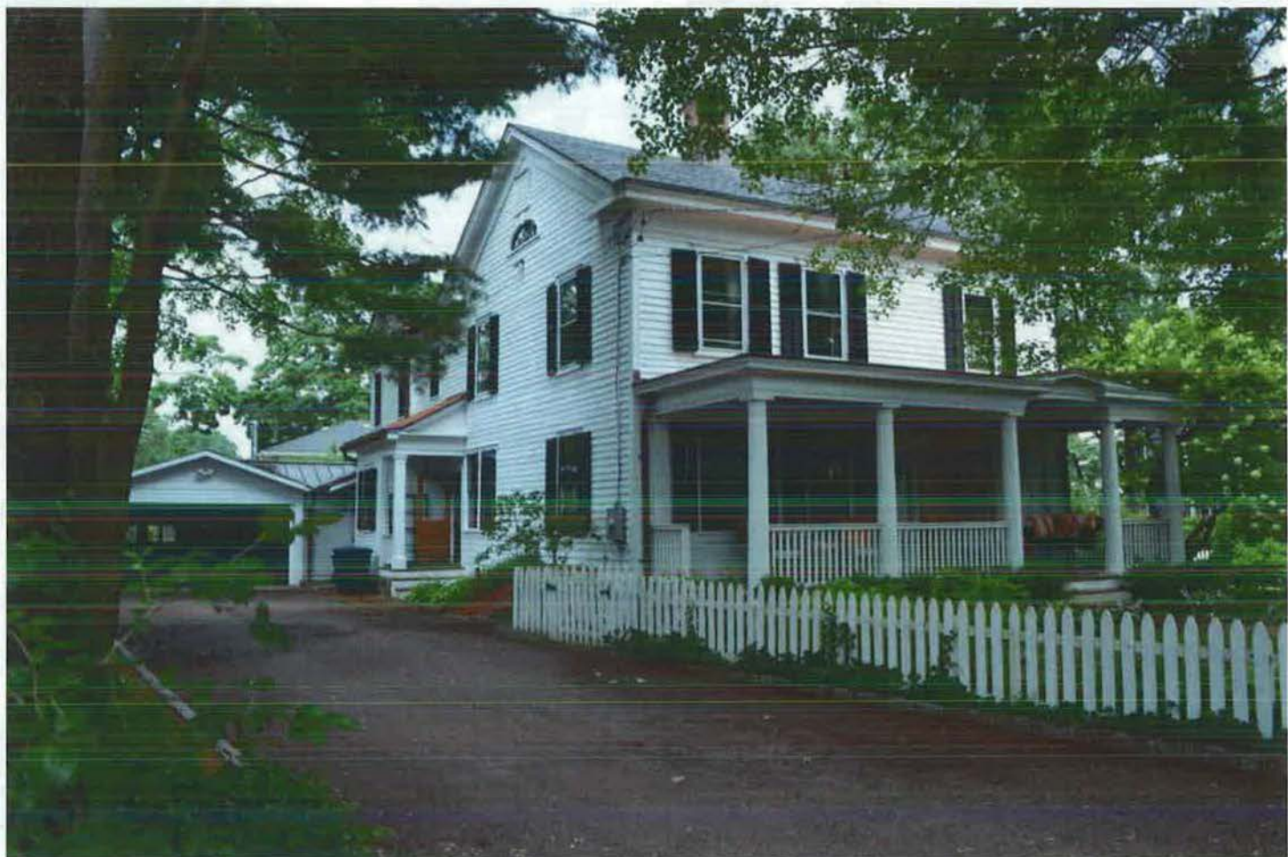
East (front) and south (side) elevations of 33 Mead Avenue, 1835, showing façade, porch, roof, and window details.
