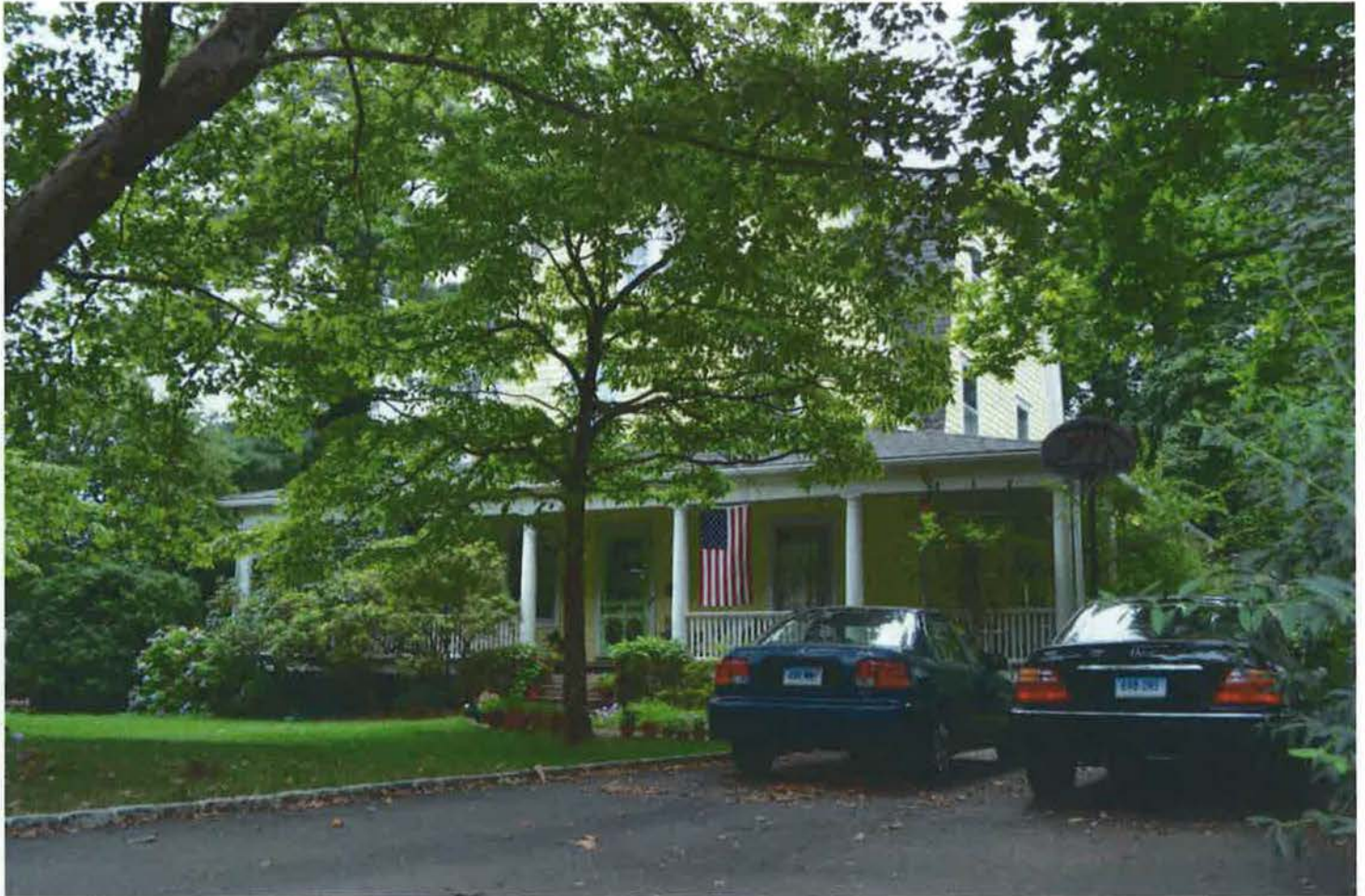
West (front) and south (side) elevations of 12 Mead Avenue, 1907, showing façade, porch, roof, and window details.
