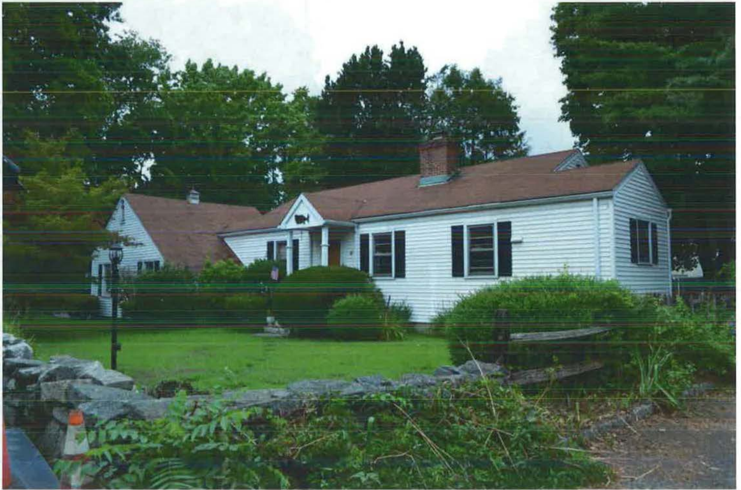
West (front) and south (side) elevations of 18 Mead Avenue, 1955, showing façade, roof, and window details. Camera facing northeast. Photograph 15 of 22.
