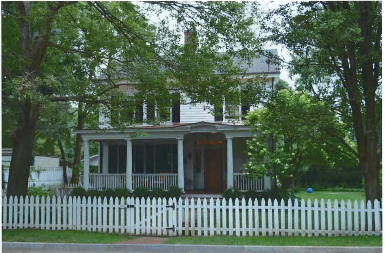
East (front) elevation of 33 Mead Avenue, 1835, showing façade, porch, roof, and window details. Camera facing west. Photograph 12 of 22.
