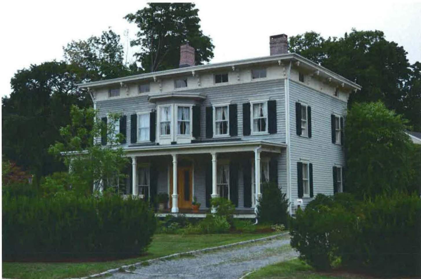
South (front) and east (side) elevations of 60 River Road, 1873, showing façade, porch, roof, and window details.
