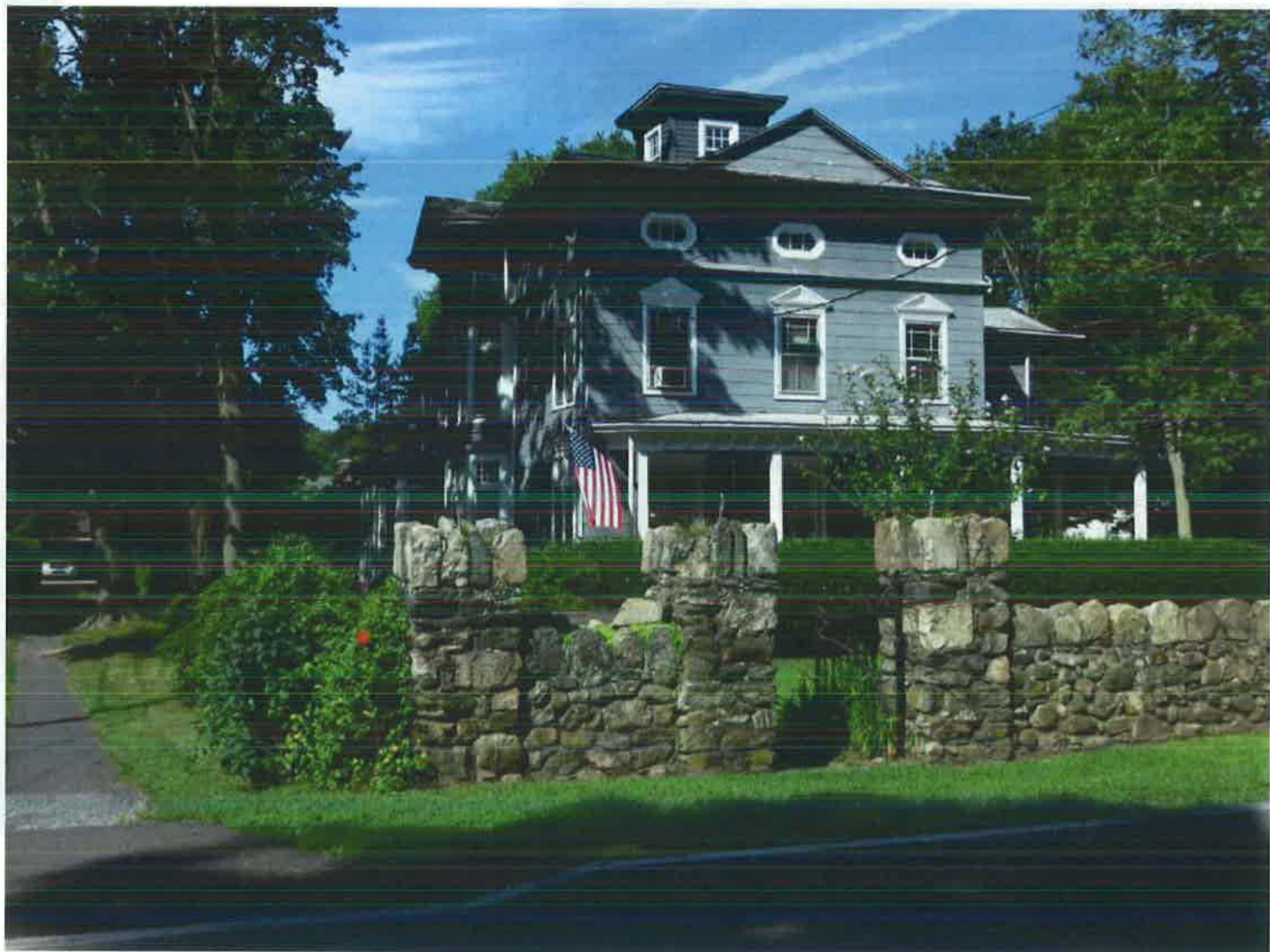
Detail of stone wall in front of 29 Mead Avenue, 1862; wall c. 1890. Camera facing northwest. Photograph 11 of 22.
