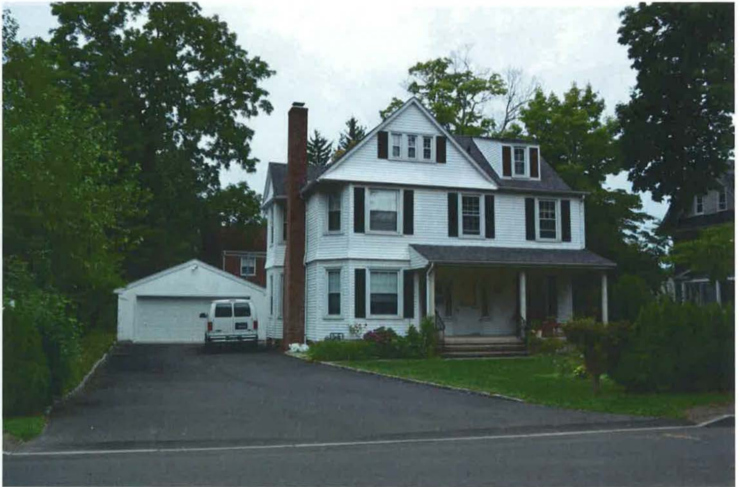
East (front) and south (side) elevations of 11 Mead Avenue, 1906, showing façade, porch, roof, and window details. Camera facing northwest. Photograph 2 of 22.
