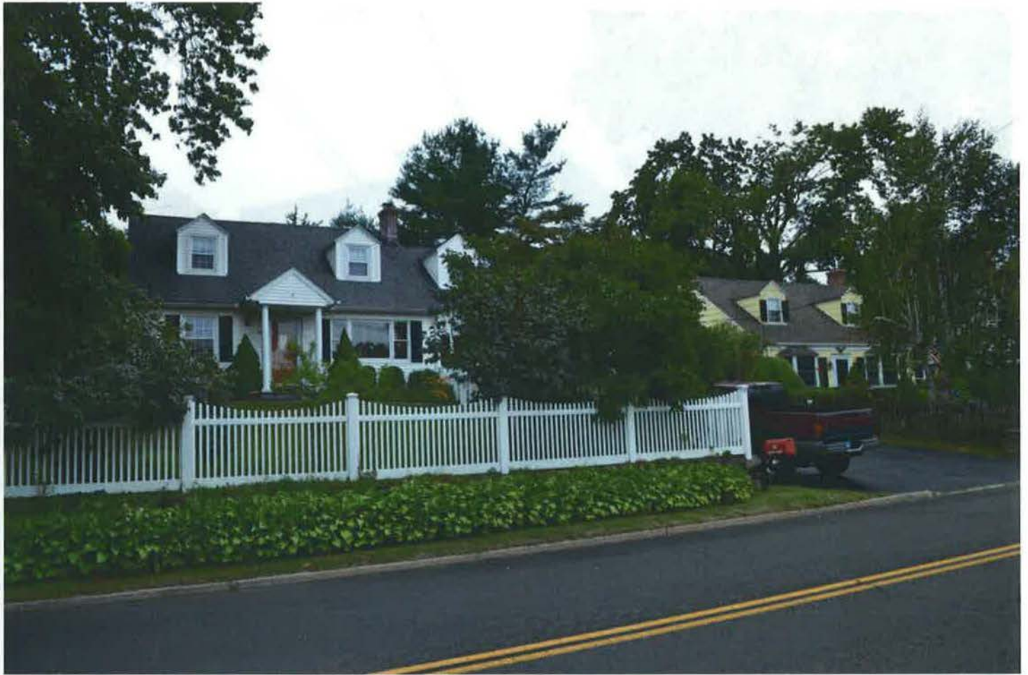
South (front) and west (side) elevations of 46 and 48 River Road, 1949, showing façade, porch, roof, and window details. Camera facing northeast. Photograph 18 of 22.
