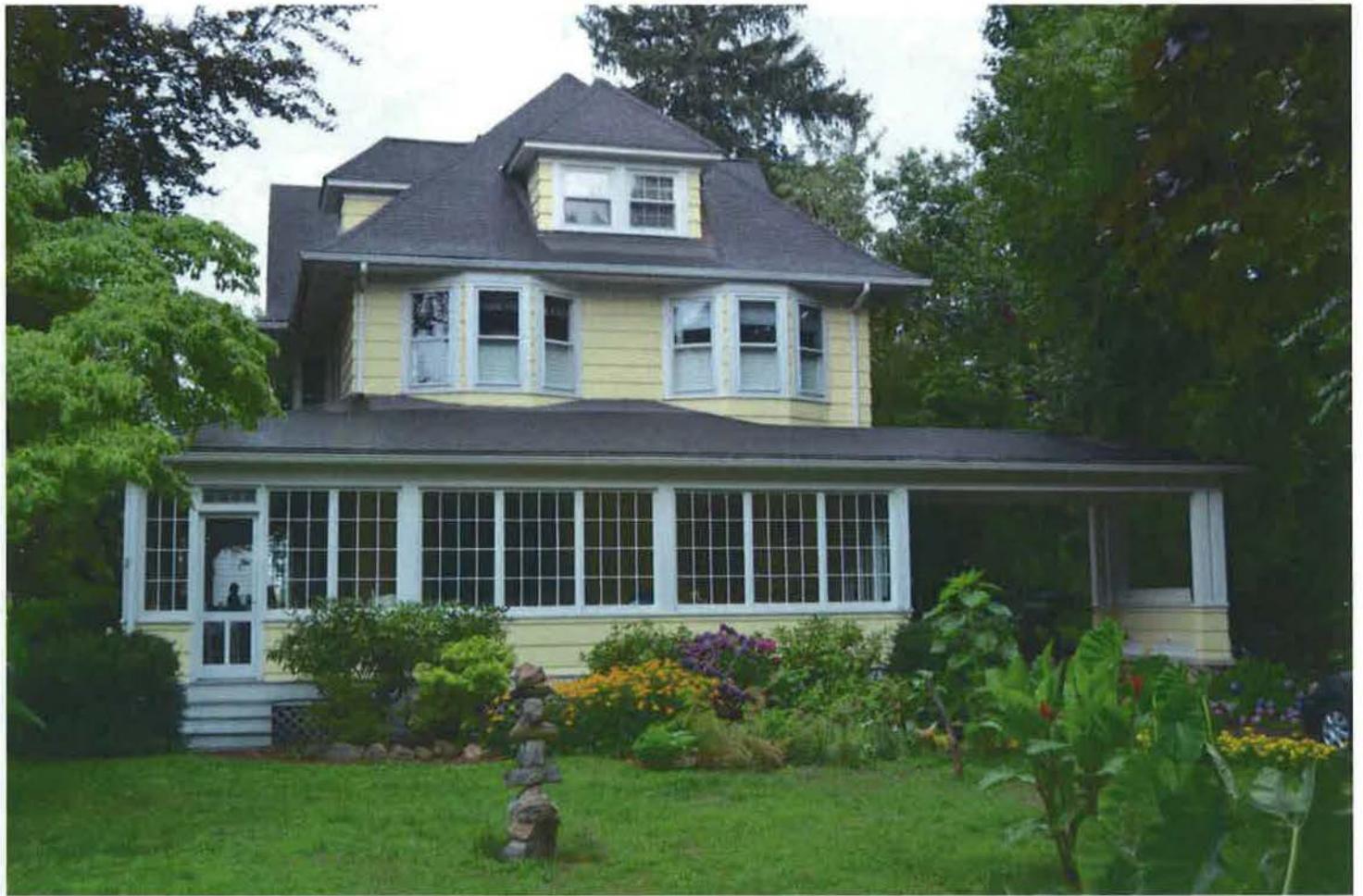
East (front) and south (side) elevations of 17 Mead Avenue, 1906, showing façade, porch, roof, and window details. Camera facing northwest. Photograph 4 of 22.
