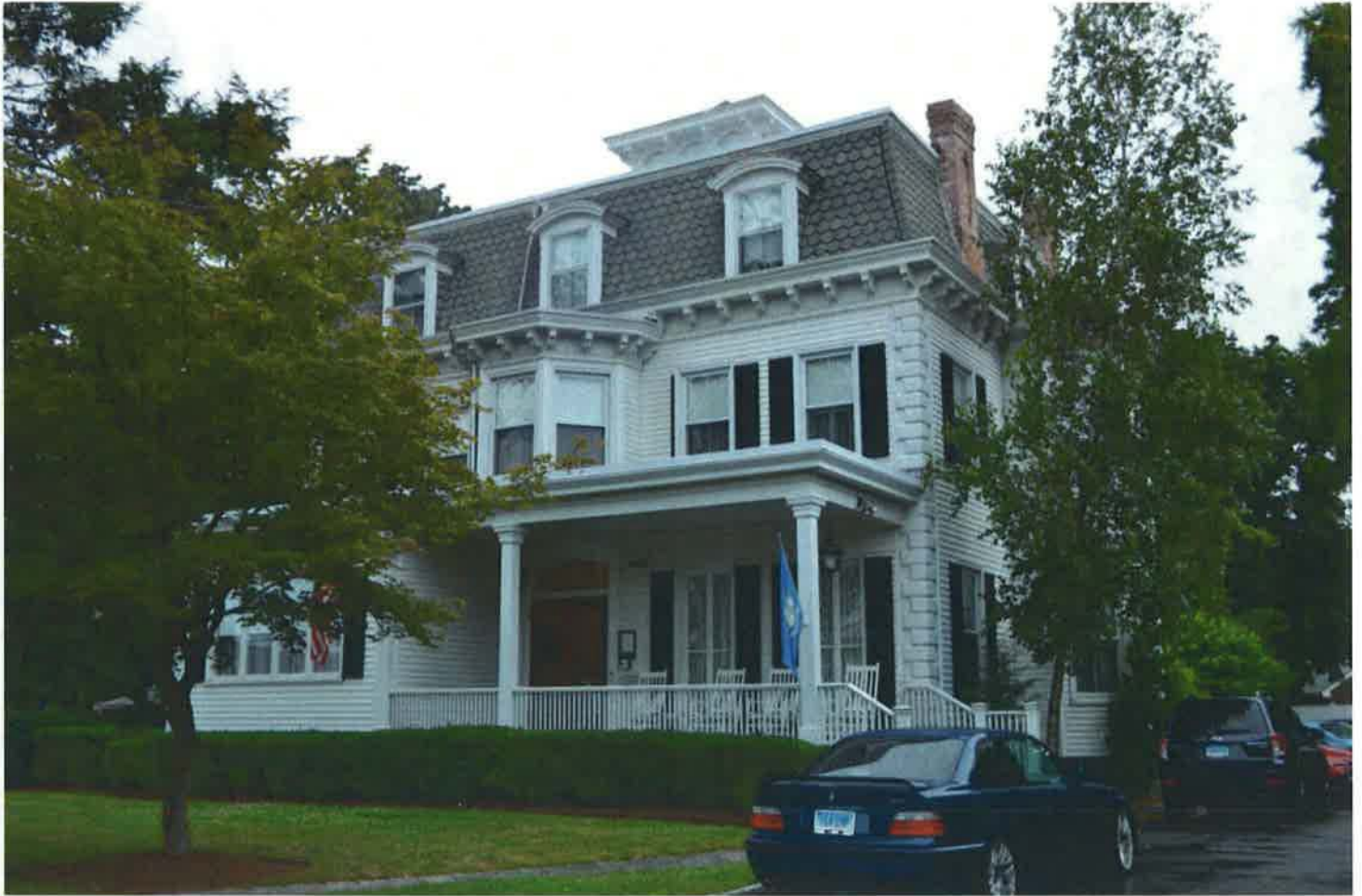
South (front) and east (side) elevations of 50 River Road, 1874, showing façade, porch, roof, and window details. Camera facing northwest. Photograph 20 of 22.
