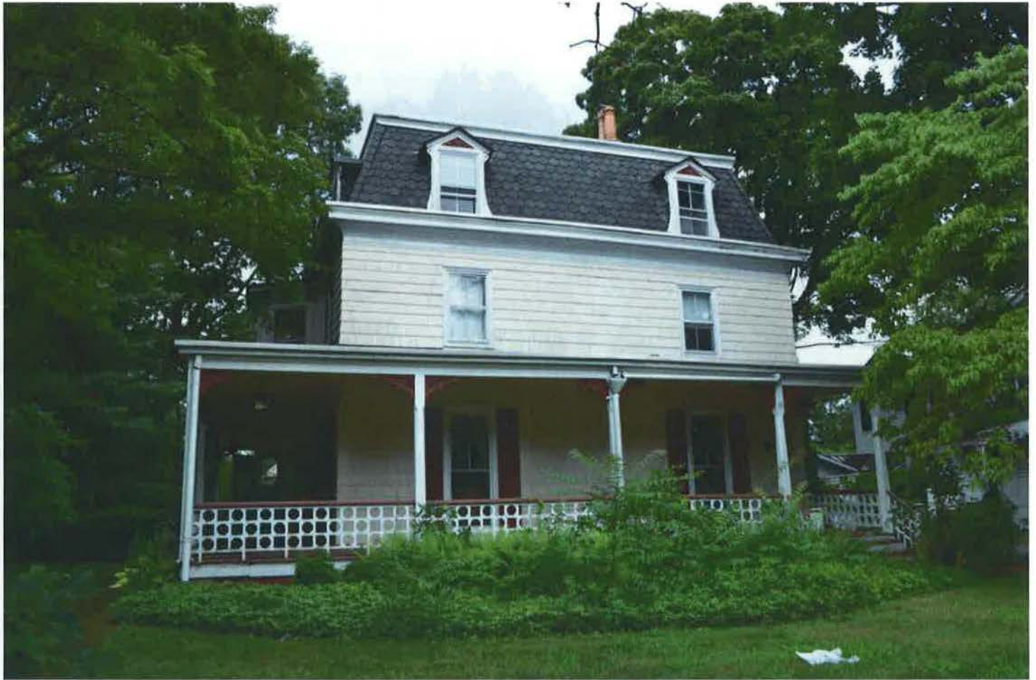
East (side) and south (front) elevations of 35 Mead Avenue, c. 1858, showing porch, roof, and window details. Camera facing west. Photograph 14 of 22.
