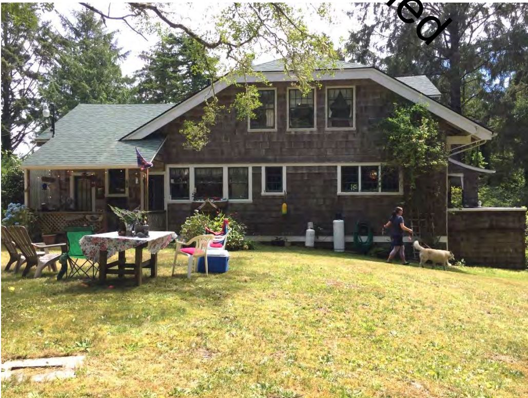
3 of 16 North facade of cottage
