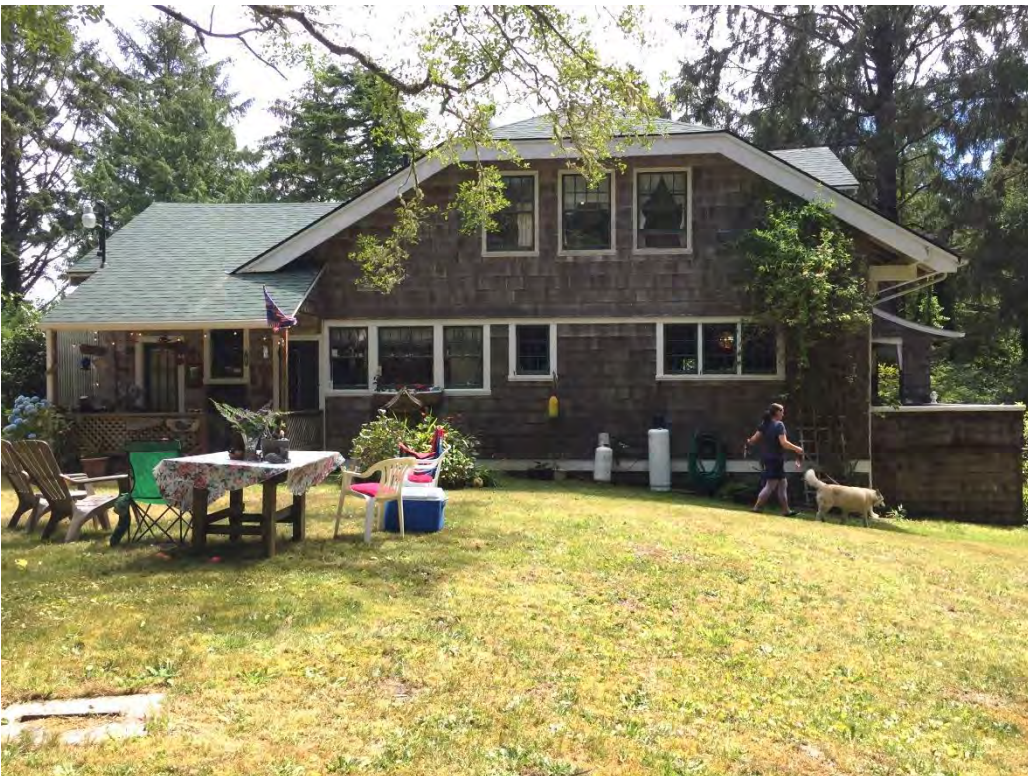
3 of 16 North facade of cottage
