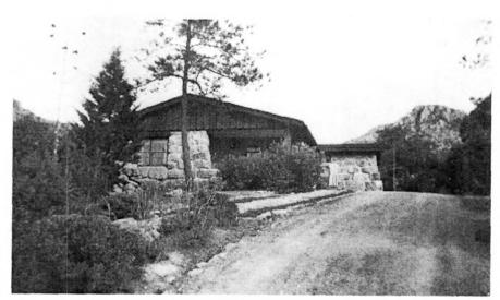
Figure 134. Front of Residence #3 shows stonemasonry with rectangular cut block and strongly battered walls, 1949. Note walkway and vegetation in front yard. View looking east.
