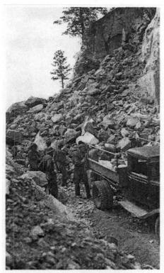
Figure 5. Clearing Bonita Canyon Highway after blasting.
