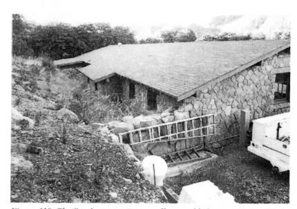
Figure 118. The Southeast retaining wall was added on to existing Equipment Shed, 2003. Note difference in stonemasonry of the Equipment Shed and adjoining utility wall. View looking northwest.
