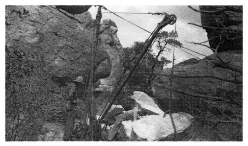
Figure 22. Trail crews used a portable hoist system with boom and winch to move large rocks.
