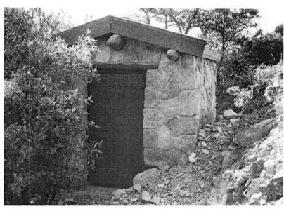
Figure 86. Second Cap Magazine with steel door, vigas, and replaced roof, 2003. View looking west.
