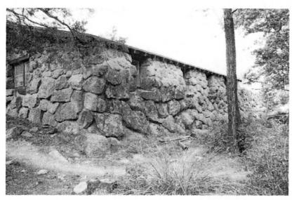
Figure 117. Northeast corner of the utility wall is constructed with largely uncut, uncoursed boulders, 2002. The wall is strongly battered. Note Warehouse incorporates wall in east and north faces. View looking southwest.
