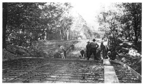
Figure 87. CCC enrollees lay wire mash prior to pouring concrete in first campground "dip," 1935. View looking southwest.
