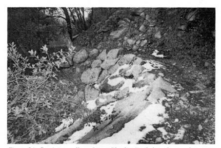
Figure 24. Retaining walls on Lower Rhyolite Trail show damage from rainstorms, 2002.
