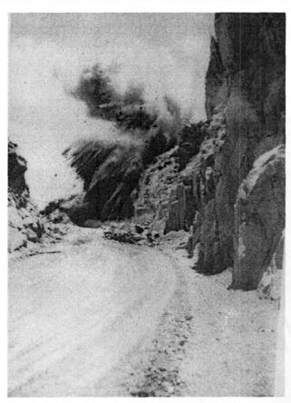
Figure 3. Blasting overhanging rock on Bonita Canyon Highway.
