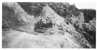
Figure 8. Clearing blasting debris on Bonita Canyon Highway
