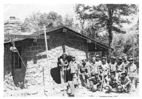
Figure 74. CCC enrollees create opening in Ranger Station to accommodate east wing of Administration Building, 1937. Note excavation for basement on left. View looking northwest.
