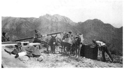
Figure 105. CCC enrollees used mules to haul materials to Sugarloaf Mountain during construction of the Lookout, 1935. Note boxes of dynamite for excavating the Lookout foundation. View looking north
