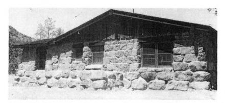
Figure 135. Basement entrance at rear of Residence #3, 1949. Note diminishing size of rock work from foundation up. View looking southwest.
