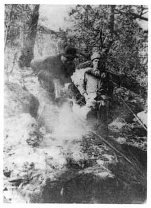
Figure 21. CCC trail crew using air-powered jack-hammer to cut through rock.
