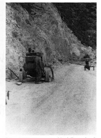
Figure 4. Air compressor used for drilling rock on Bonita Canyon Highway.
