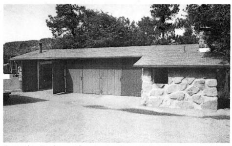
Figure 124. Warehouse with modern bay doors, 1993. Walls are composed of uncoursed stone and are slightly battered. Note the decreasing size of stone from the foundation up. View looking northwest.
