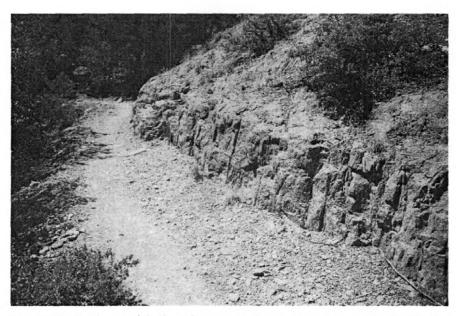
Figure 23. Evidence of drill work in upper slope cuts on Lower Rhyolite Trail.
