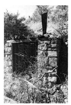
Figure 85. Ruins of first Cap Magazine, 2002. Roof has partially collapsed. Note remains of wooden vent. View looking northwest.
