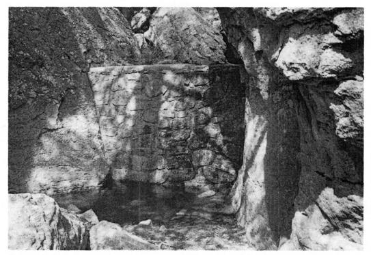
Figure 28. Echo Canyon dam was constructed of concrete and faced with stone, 1993.
