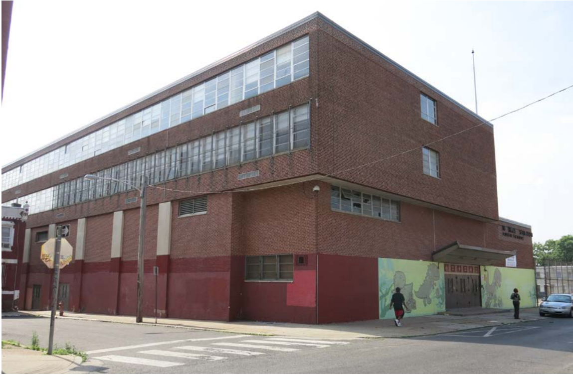
Photo 3: North and west façade of M. Hall Stanton Elementary.
