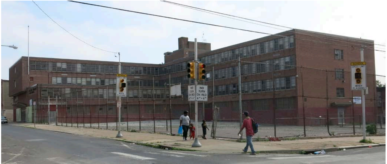
Photo 1: M. Hall Stanton Elementary School. South and West facades. Photo taken from SW corner of N.16 th Street and W. Cumberland. Camera facing NE. Note fenced play area (which doubles as parking) was site of original Stanton School building, demolished c.1967.
