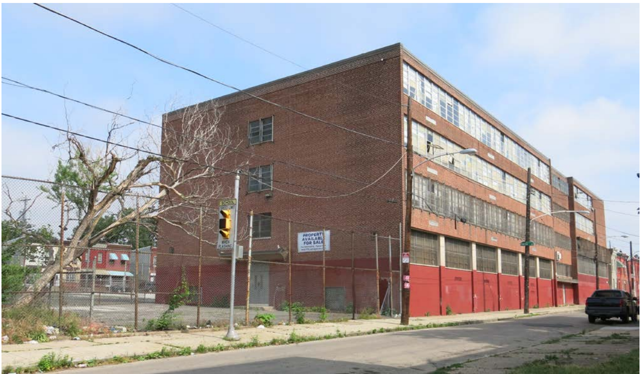
Photo 2: East and south façade of M. Hall Stanton Elementary.
