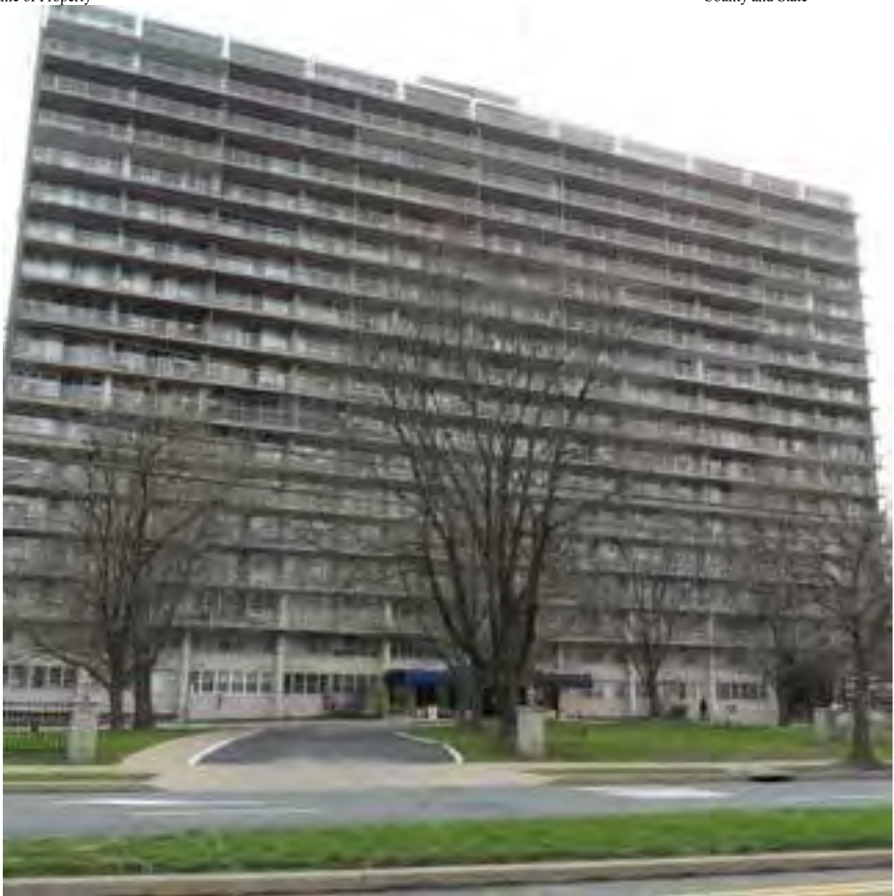
Figure 9 – Chestnut Hill Tower, 7600 Stenton Avenue, Philadelphia, PA. Designed in 1962 by George W. Neff.
