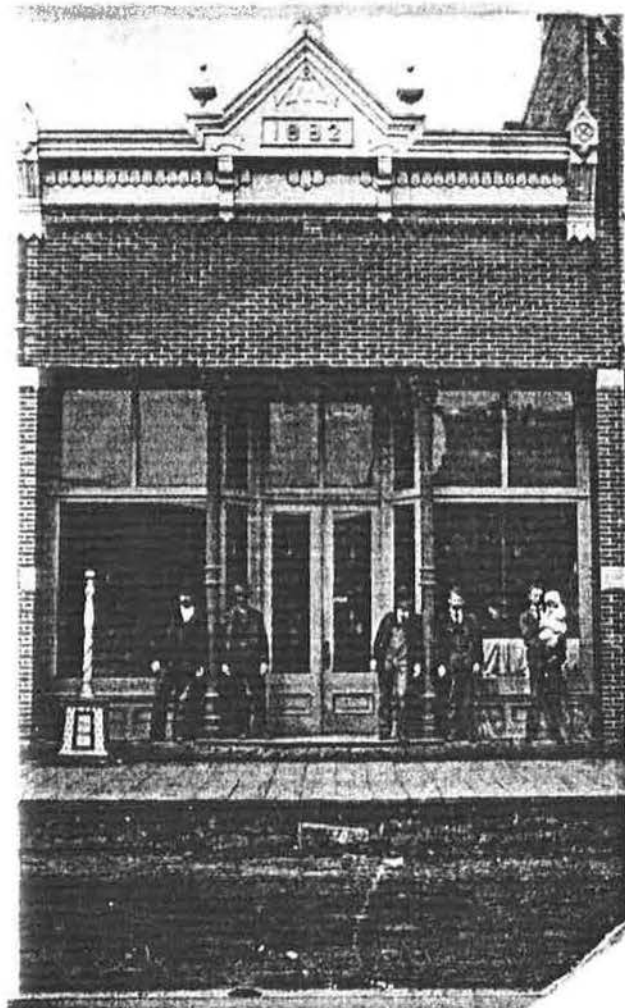
One of the "Four Sisters" at 319 Jackson Street circa 1895. The photograph shows how a limestone foundation elevates the boardwalk well above street grade.
