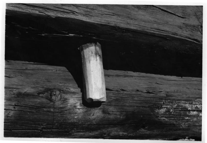
Fix pege used in construction of
