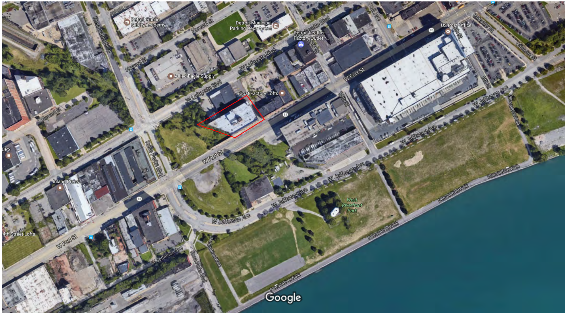
Edson, Moore & Company Building 1702 West Fort Street, Detroit, Wayne County, Michigan
