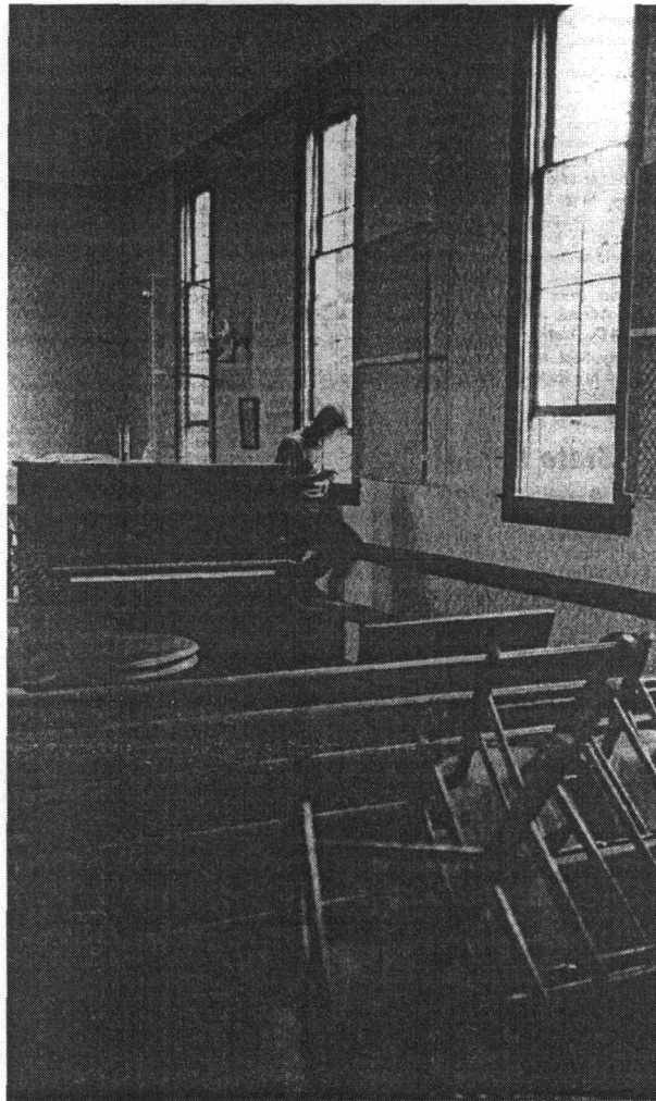
Figure 27: Window repair by County Youth Corps, 1984 (DeWitt Observer , August 18, 1984)
