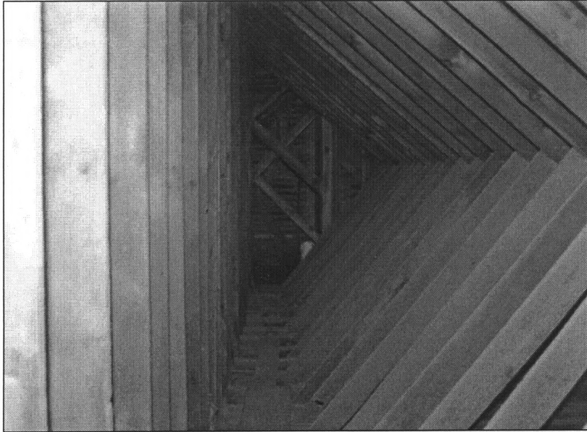
Figure 4: Attic framing, vertical 2x6 posts run down center of plan, angled struts join midway with roof Tower framing visible in background, view northward along east side of attic (photo by Floyd Soenksen)
