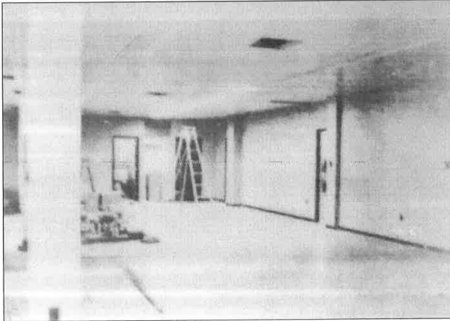
Figure 24: Interior view, third floor looking northeast (Grinnell Herald-Register , December 2, 1957)
