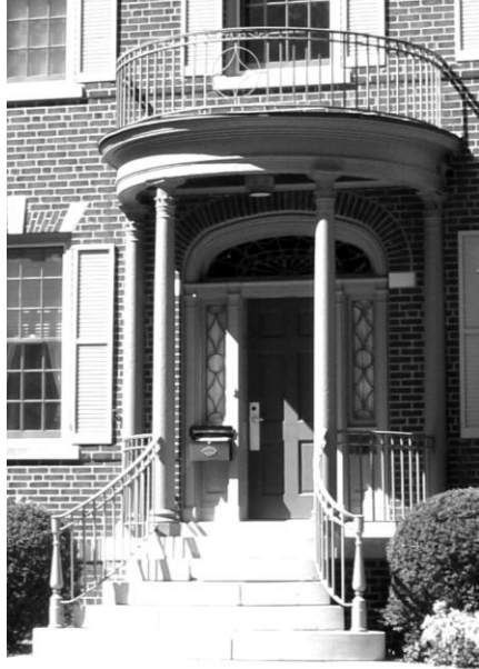
Image J Entrance Portico.
