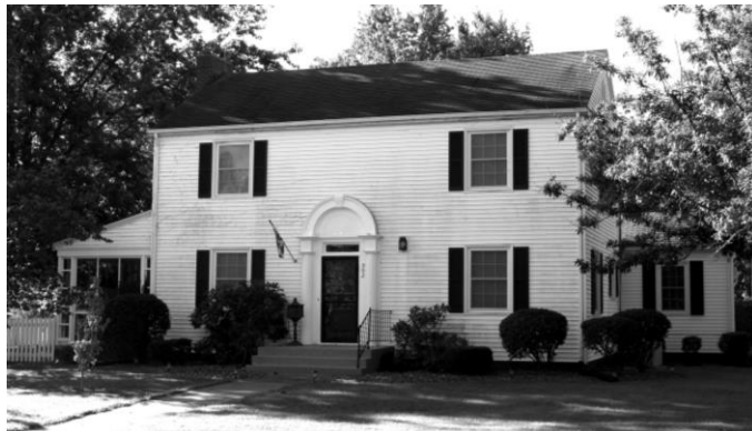
Image W C.C. Thompson House (built 1936). Extant. 902 E. Patterson St.
