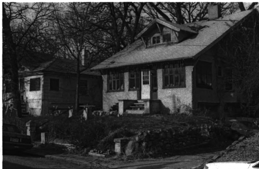
2715 (left, I-B) and 2711 (right) Linden Street (both 1913) (Photo by Jim Jacobsen, December 7, 1999)
