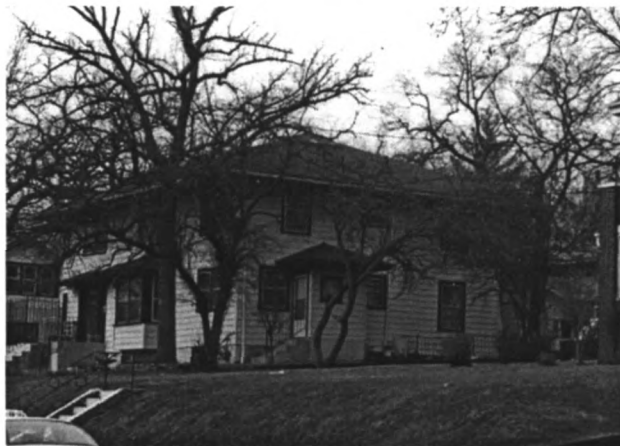
2715 High Street (1921) (photo by James Jacobsen, February 23, 2000)
