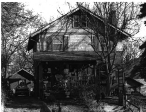
563 28 th Street (1913) (Photo by Jim Jacobsen, December 7, 1999)
