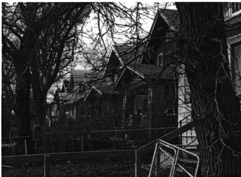
Pattern of gable fronts, Linden Street, view northwest (Photo by James Jacobsen, February 23, 2000)
