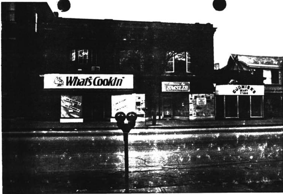
Front of building with context.
