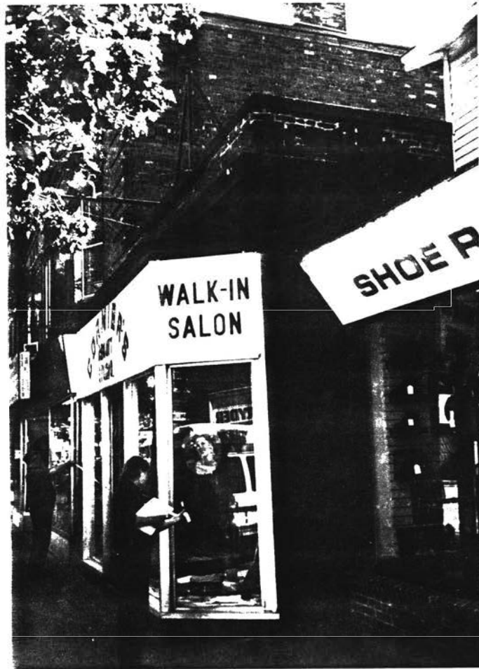
Showing original trim (sign board covers prism glass)
