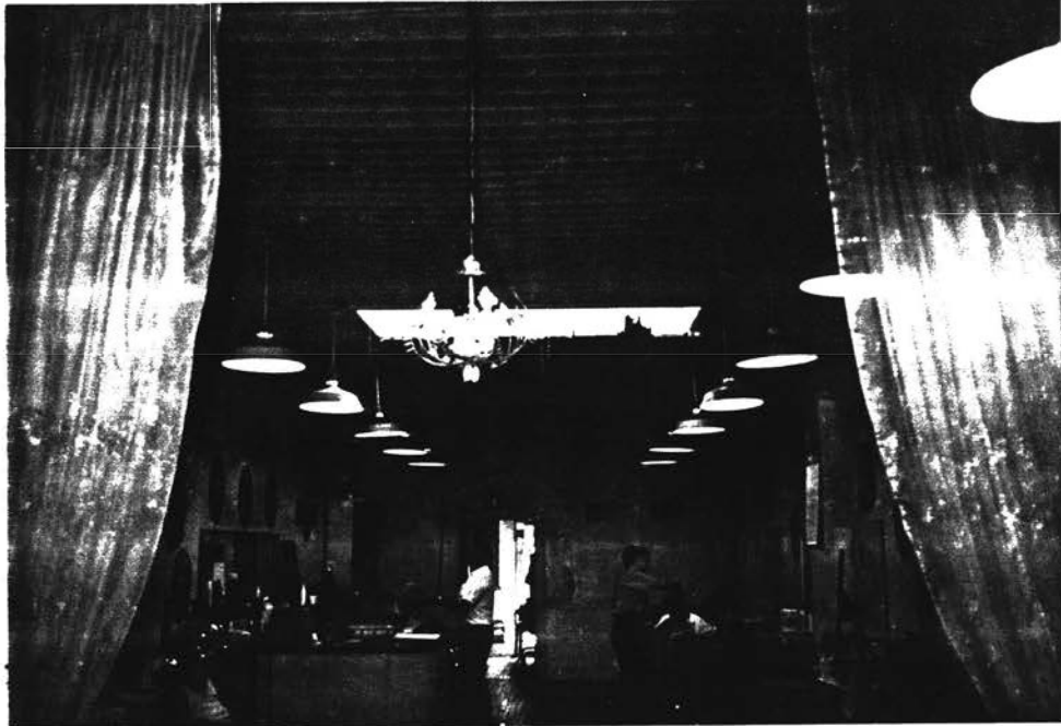
Inside 1 story portion Tin ceiling appears original
