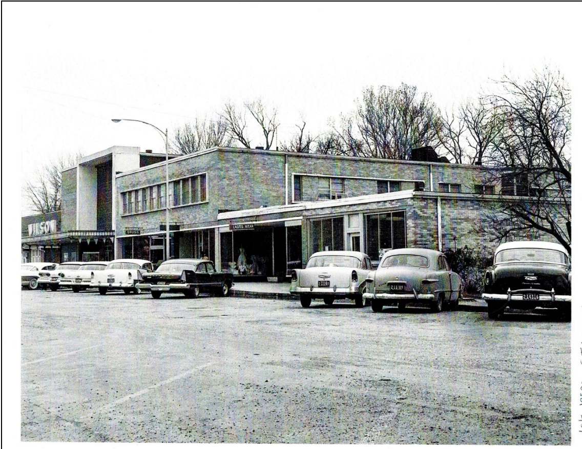
Figure 13: Wilson Theatre and Commercial Building, ca. 1955 (Photo courtesy of the Lawrence Group).
