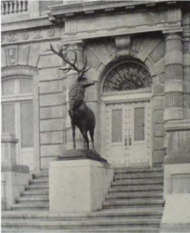
Elk statue and entrance, 1926. Note original door and transom treatment. Source: The Architectural Forum, September 1926
