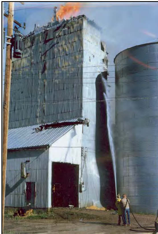
Fire at circa 1950 grain elevator, camera facing northwest, August 1972. (Courtesy: Tammie Delaney personal files, Hayden, CO)
