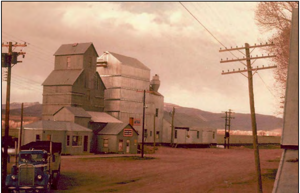
Hayden Grain Elevator shortly after construction of the pellet mill and half of the processing plant, camera facing northeast, circa 1955. (Courtesy: Tammie Delaney personal files, Hayden, CO)
