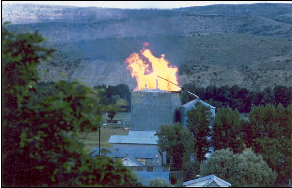
Fire at circa 1950 grain elevator, camera facing north, August 1972. (Courtesy: Tammie Delaney personal files, Hayden, CO)
