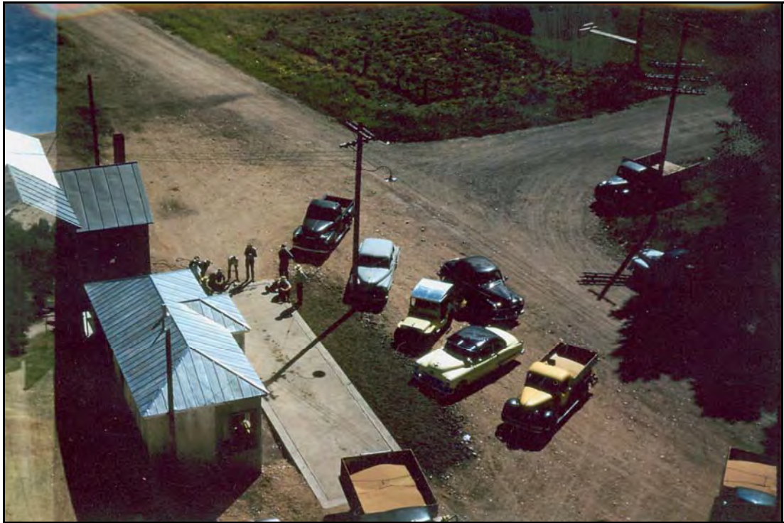
View of scale house and sales office and exterior concrete deck, circa 1953. (Courtesy: Tammie Delaney personal files, Hayden, CO)
