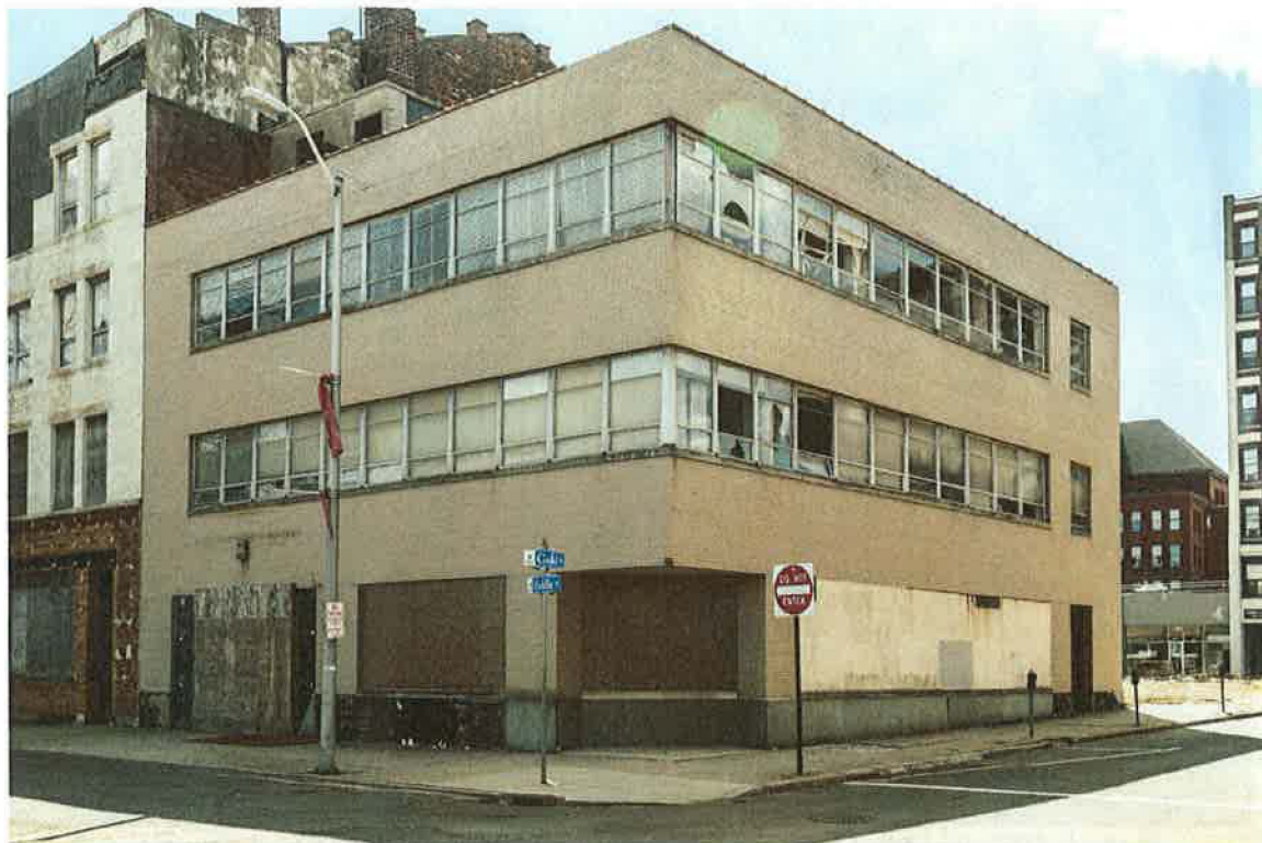
Photo 3. 209-211 Middle Street view southwest showing façade and north elevation.
