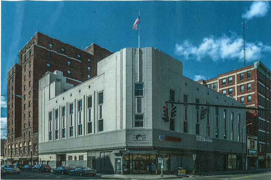
Photo 1. 1087-95 Main Street view northwest showing south and east elevations.
