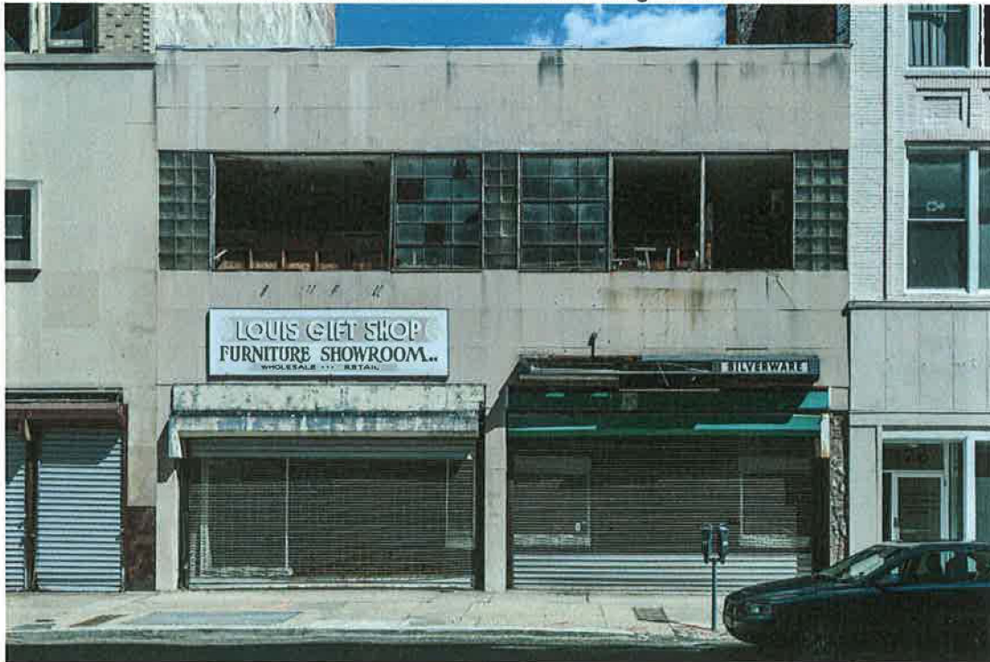
Photo 2. 1128-36 Main Street view east showing façade.
