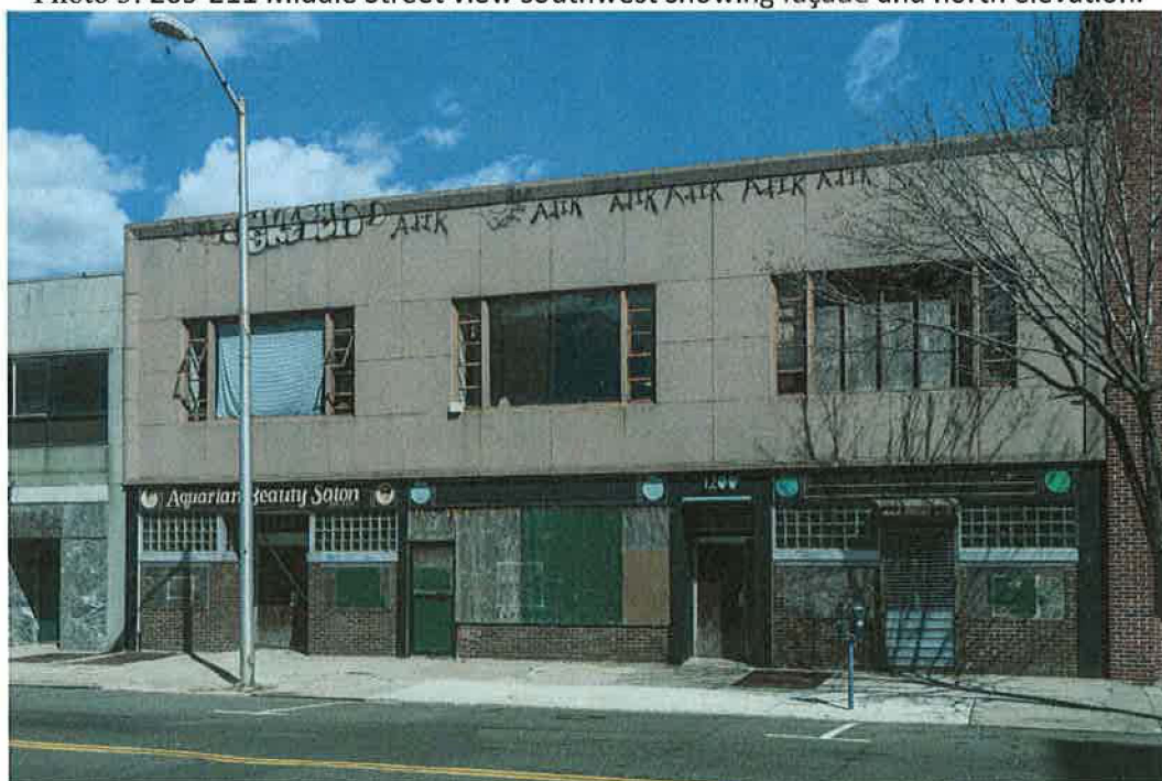
Photo 4. 1200-10 Main Street view east showing façade.
