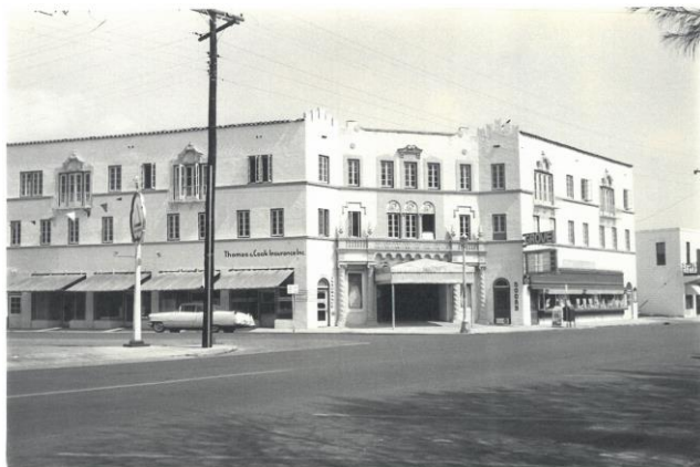
Figure 9: Early 1950s photograph of the Coconut Grove Theater before the Engle/Parker renovations were completed. Note the parapets along the roofline (now removed) and the commercial bays. Source: University of Florida Architectural Archives
