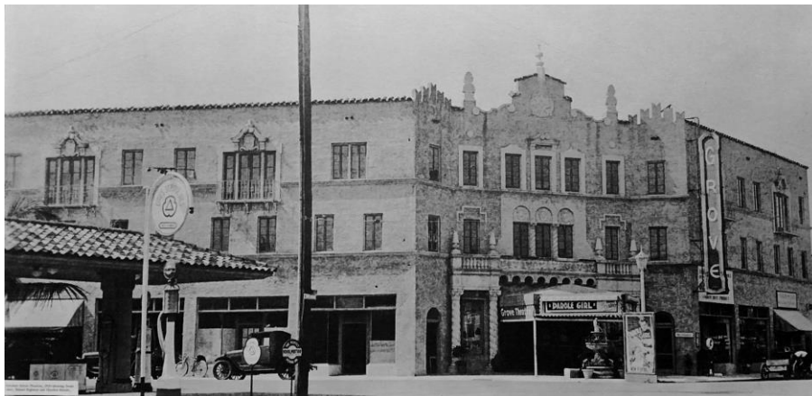
Figure 8: 1930s photograph of the Coconut Grove Theater. Taken from across Main Highway and Charles Avenue, the photograph demonstrates the original Kiehnel and Elliott design, including the building’s pediment, parapets, and original storefronts. Source: Architectonica International Coconut Grove Playhouse Historic Report
