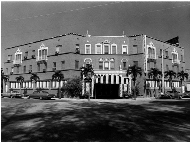
Figure 13: 1971 photograph of the Coconut Grove Playhouse’s exterior. The parapets had been removed, and the commercial bays filled in with ribbon windows. Source: HistoryMiami Archives and Research Center
