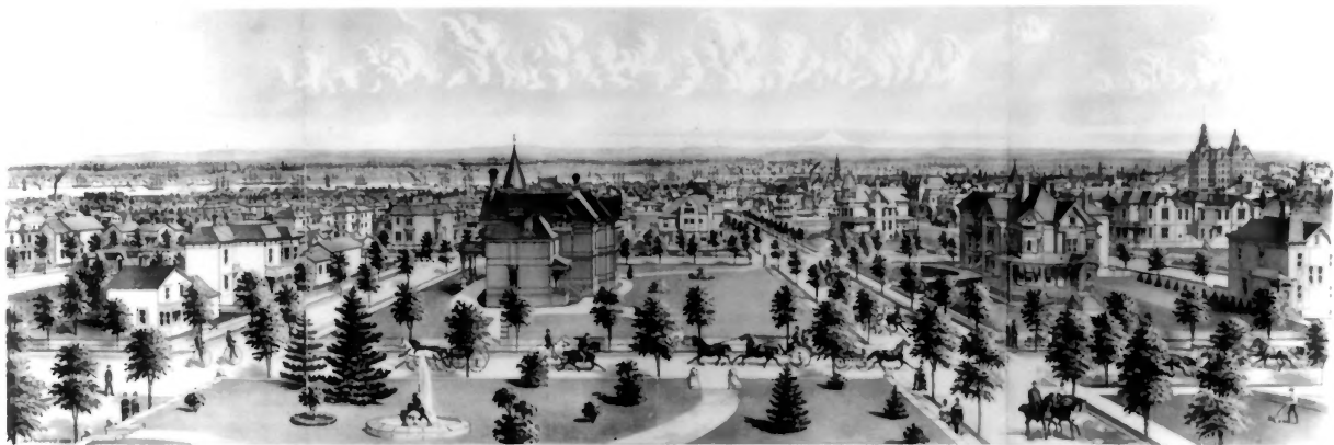
PORTLAND, OREGON THE METROPOLIS OF THE PACIFIC NORTHWEST
