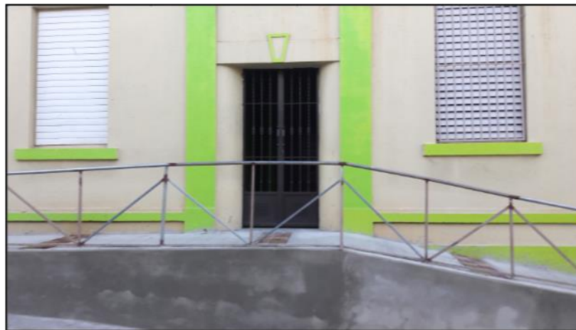
Picture 2: Oliver Hazard Perry's main entrance, facing west (San Blas Street).
