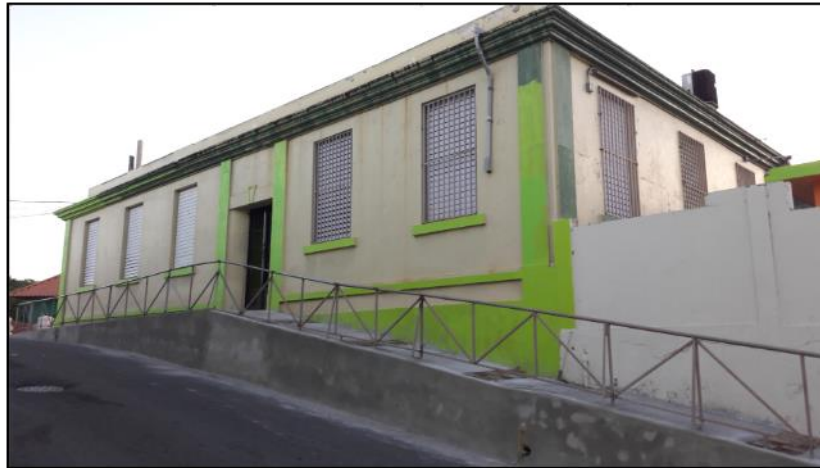
Picture 1: Western façade.
