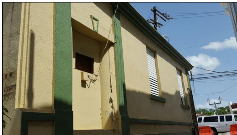
Picture 4: View of the Eastern façade.
