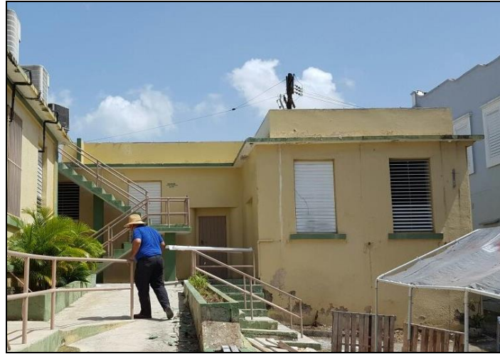
Picture 5: View of the southern façade looking approximately north.
