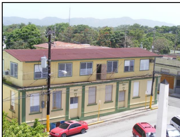
Figure 9: Oliver Hazard Perry School, with second floor built in the 1980. Photo taken from parish church bell tower (2013).
