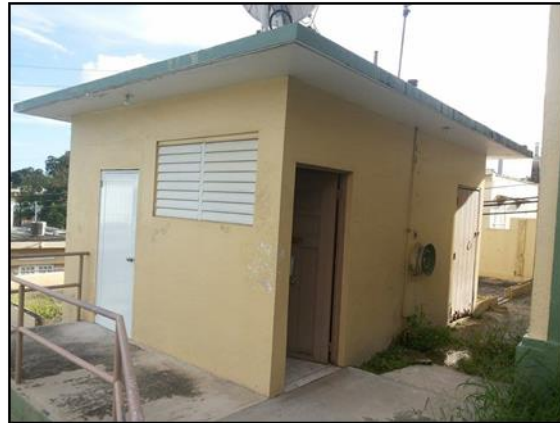
Picture 8: Bathrooms in a small concrete building looking southwest (2015).
