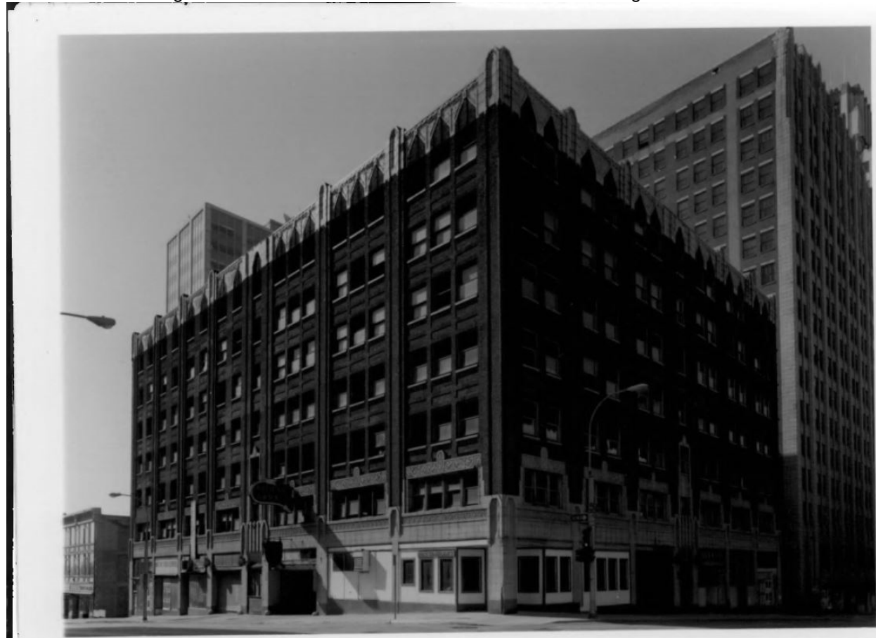
Figure 12: The National Garage, 1100-1110 McGee St, Kansas City, MO. Demolished. Photo from 1999. Source: National Register of Historic Places Nomination: The National Garage.
