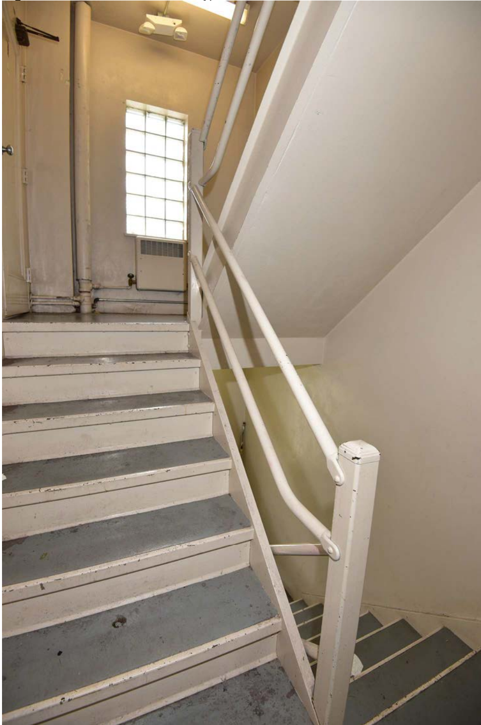
Figure 8: North stair at 3rd floor, typical.
