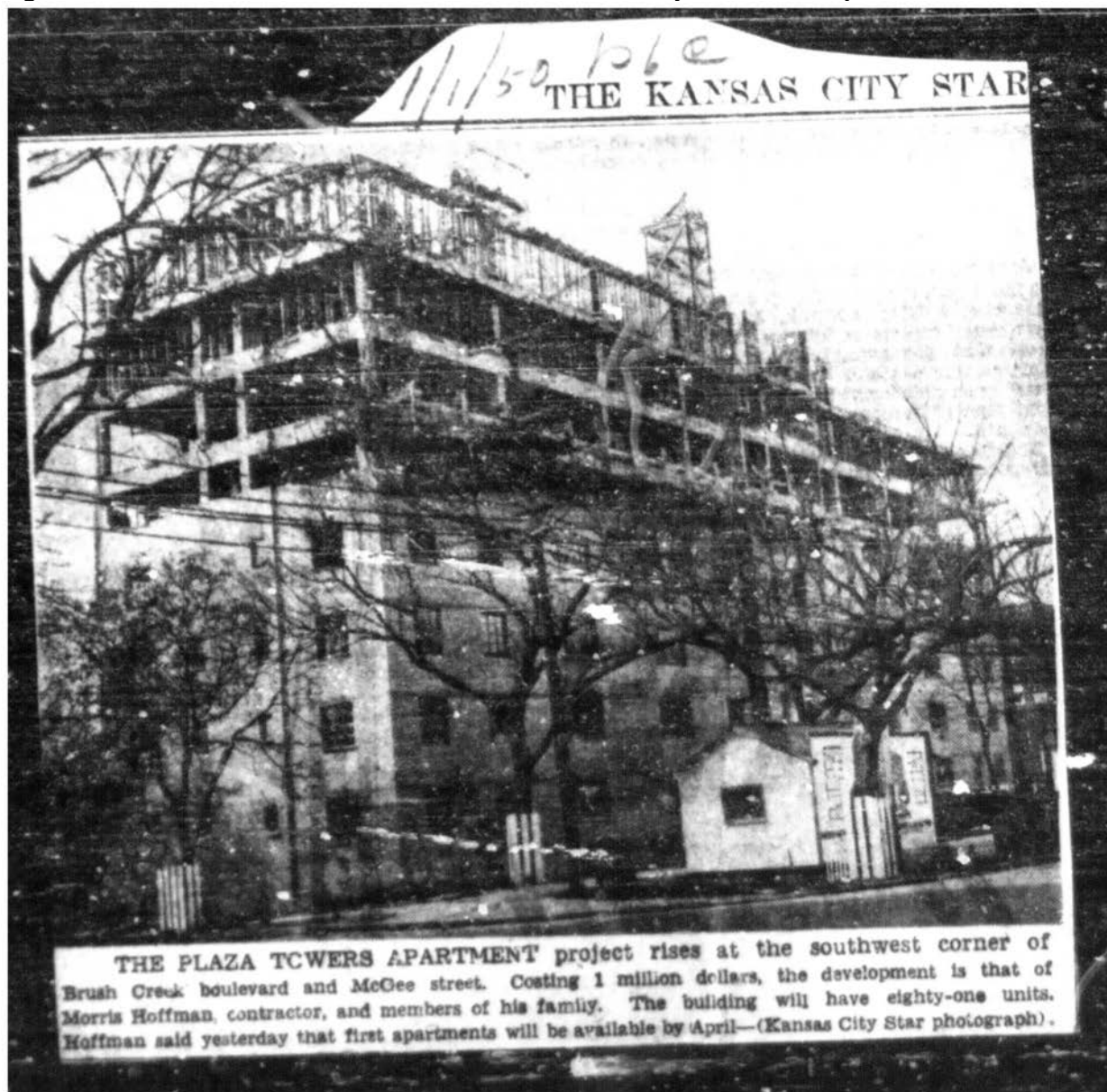
Figure 4: Plaza Towers under construction. Source: Kansas City Star , 1 January 1950.
