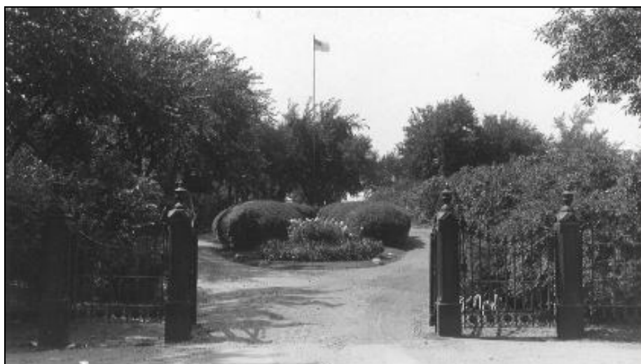
Figure 23. Photograph of the 10 th Street SW entrance with the original metal gates and fence in place.
