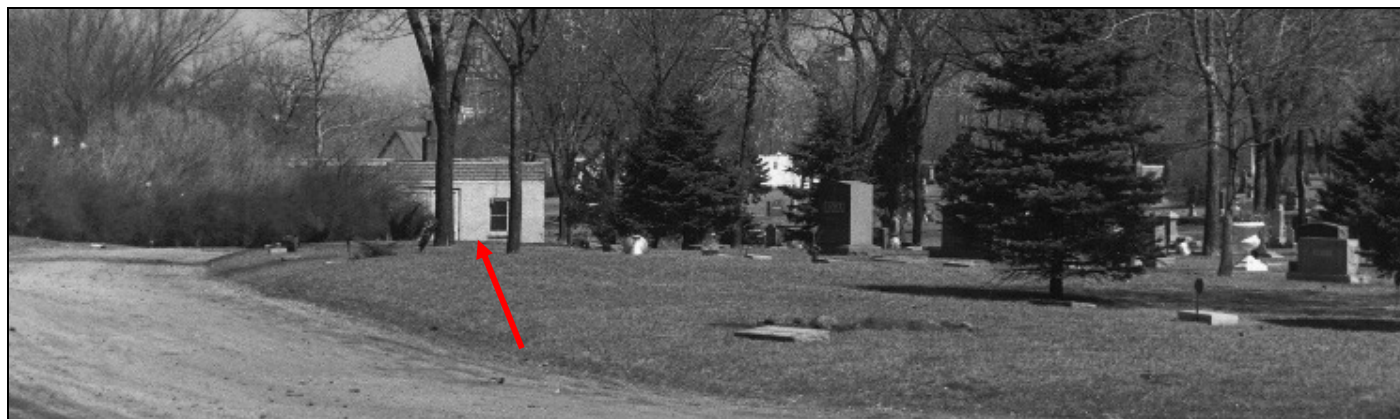
Figure 38. Circa 1950(?) photograph of the Oakland Section looking NNE, with the flat-roofed stucco and tile block maintenance building in the background (red arrow). Copy provided by the Lee P. Loomis Archive of Mason City, Iowa (Safford W. Lock Collection Photo #26517-A).
