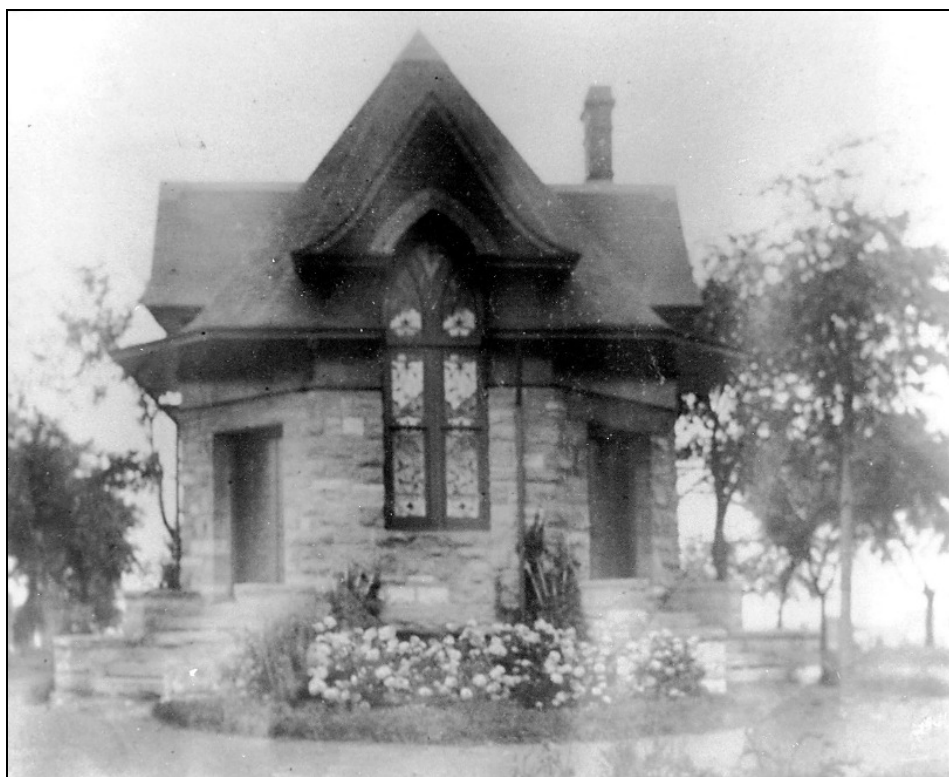
Figure 24. Photograph of the stone chapel at Elmwood Cemetery built in 1895.
