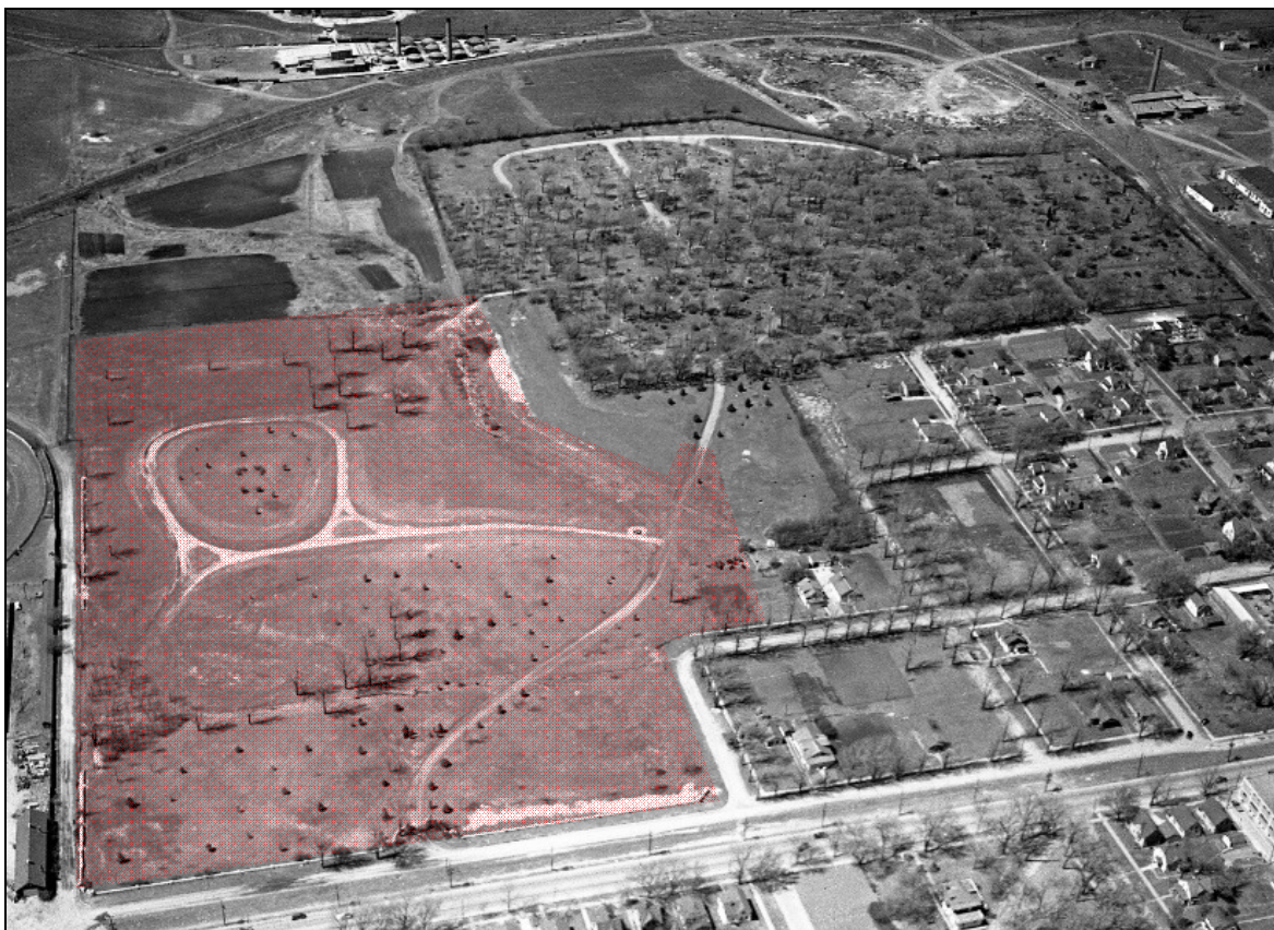
Figure 31. 1948 Aerial view of the Elmwood-St. Joseph Cemetery looking to the WNW showing area under construction (red shaded). South Federal Avenue is in the foreground. The older sections of Elmwood and St. Joseph cemeteries are in the upper right corner and the newer south addition to Elmwood is in the lower left corner. Copy provided by the Lee P. Loomis Archive of Mason City, Iowa (Safford W. Lock Collection SL18142).
