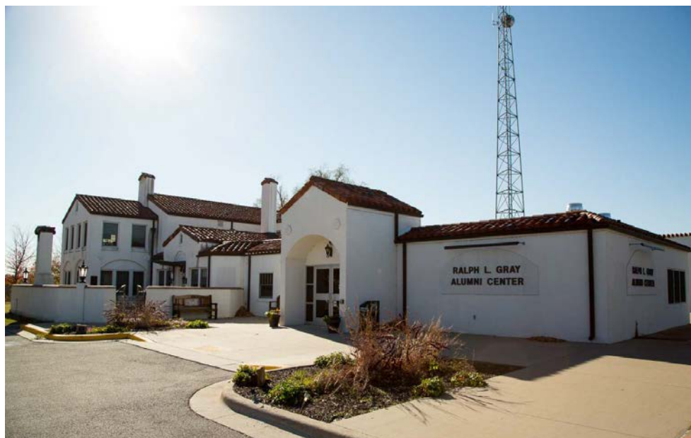
Figure 6: Northeast elevation facing southwest.
