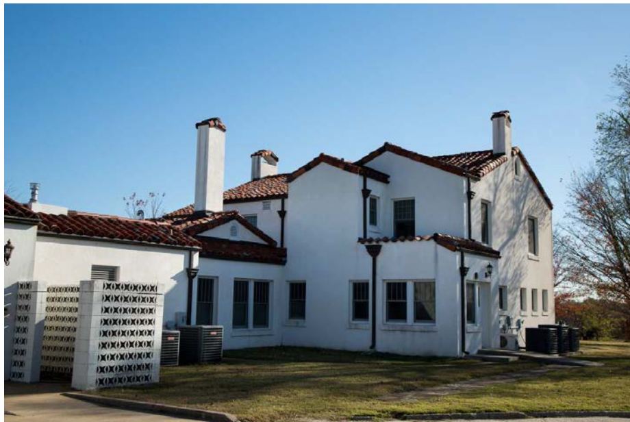
Figure 12: West elevation facing southeast. This side breaks from the symmetry of the south and east elevations.
