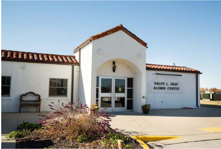
Figure 7: East elevation facing northwest. This photograph highlights most of the 2009 renovations, where this new space was created, taking the footprint of the former 3 car garage.
