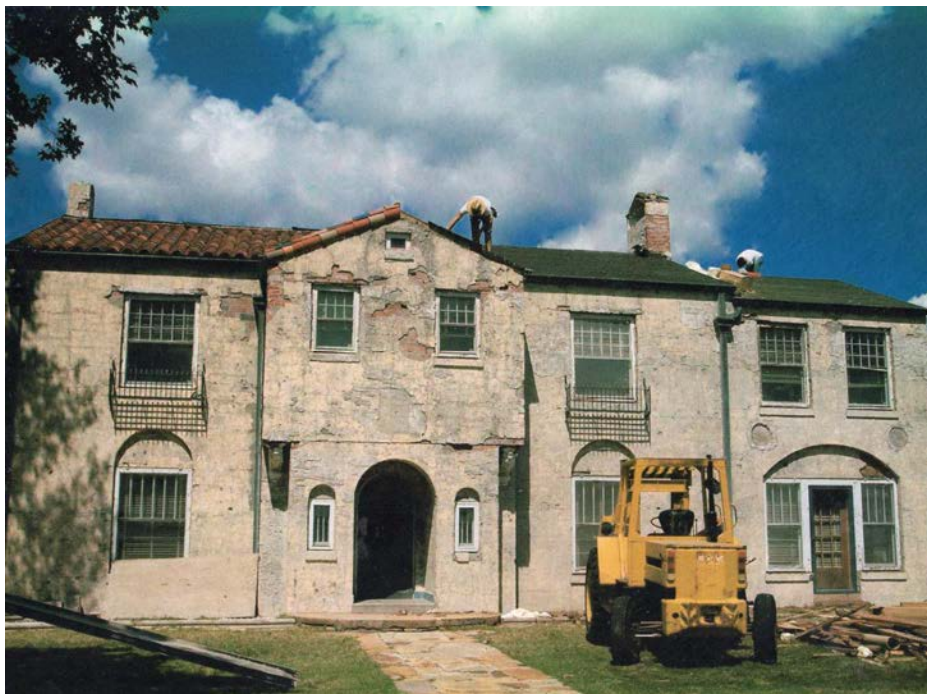
Figure 30: South elevation facing north during the 2006 exterior renovations. The original clay roof tiles were removed, restored, and reapplied. The exterior stucco was replaced. The windows and gutters were removed, and replaced with replicas that matched the original 1926 elements. Courtesy of MSSU Archives
