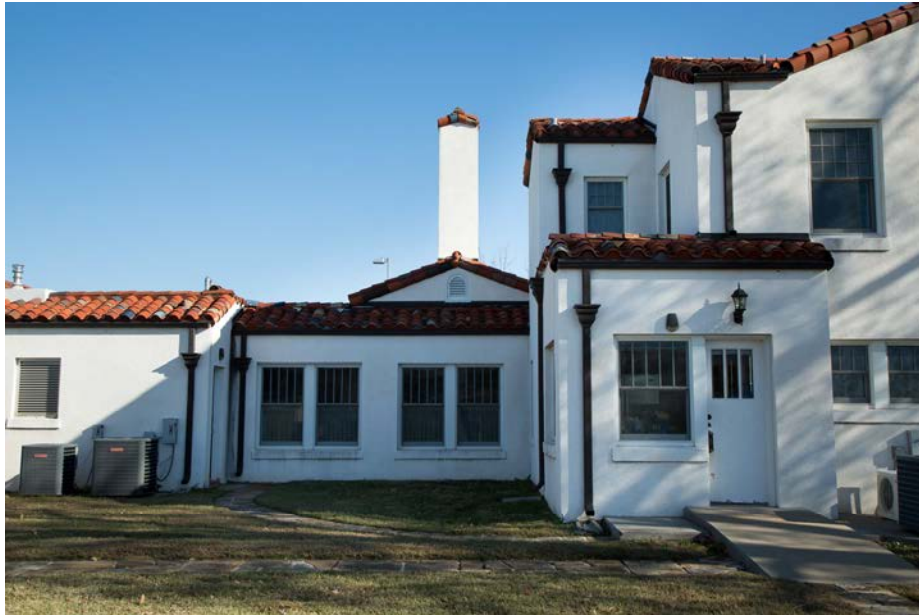
Figure 13: West elevation facing east.
