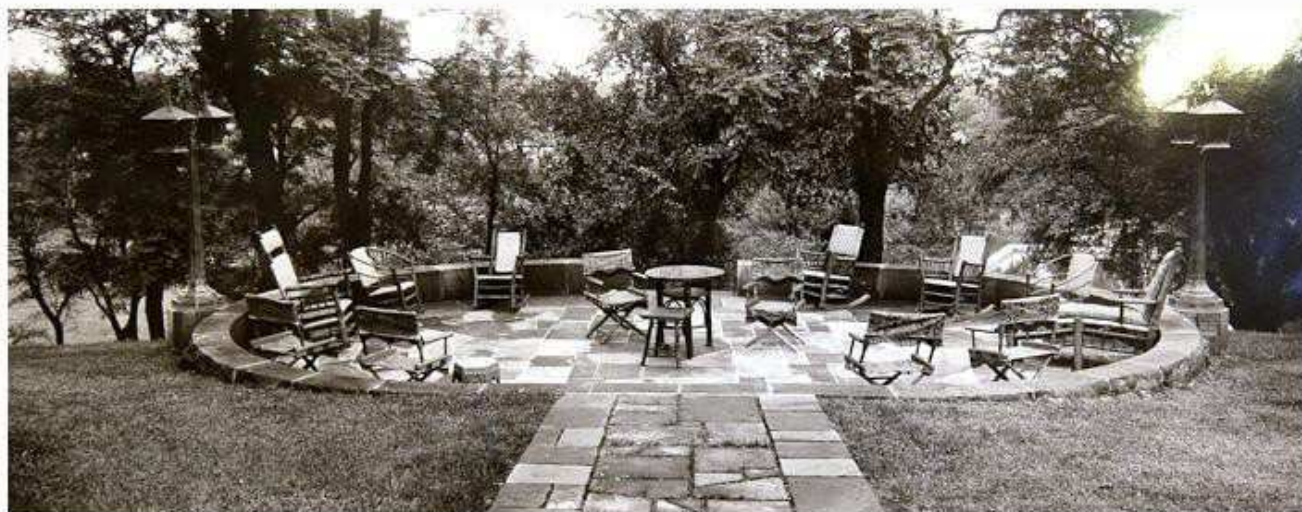
Figure 21: Original sand stone walkway and patio, c. 1930s, south approximately 40 yards of the south elevation. Both elements remain intact. Courtesy of MSSU Alumni Association
