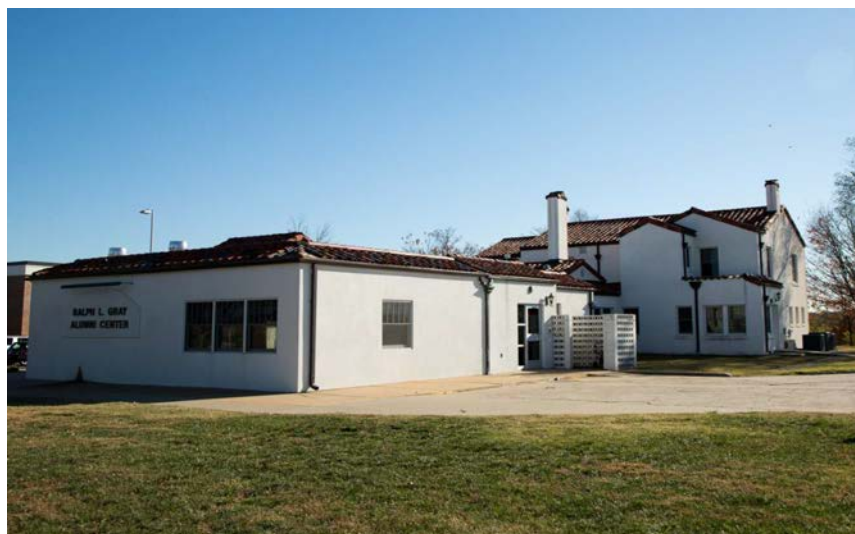
Figure 15: North and west elevations facing southeast.
