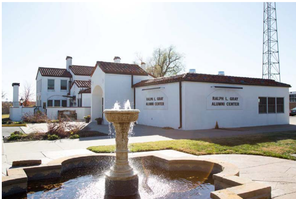
Figure 5: Northeast elevation facing southwest. The fountain in foreground is original to the Hare and Hare landscaping from 1926.
