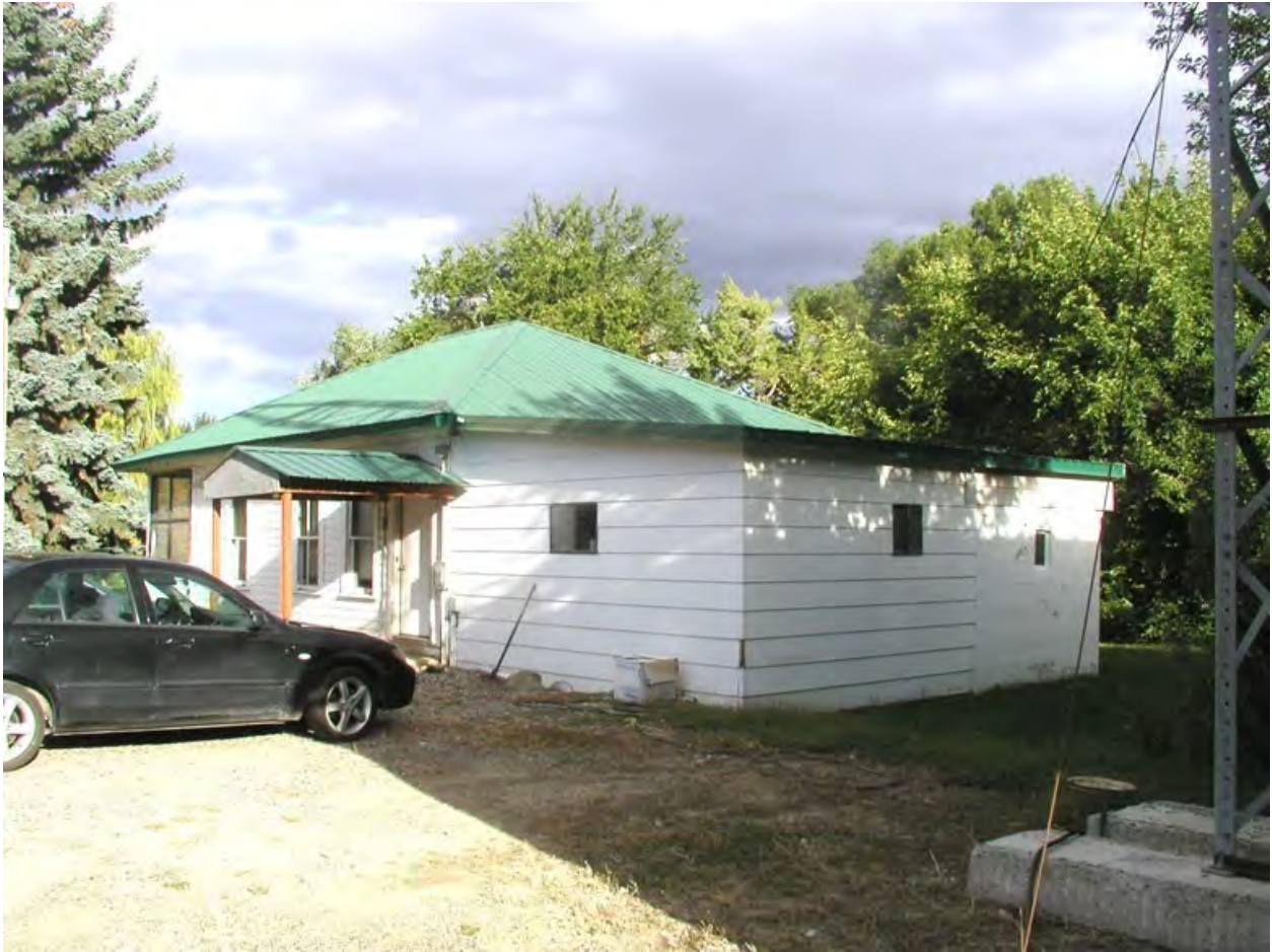
Description and view of camera: South and East elevation, view to northwest Photograph: MT_YellowstoneCounty_HuntleyProject Office_0005
