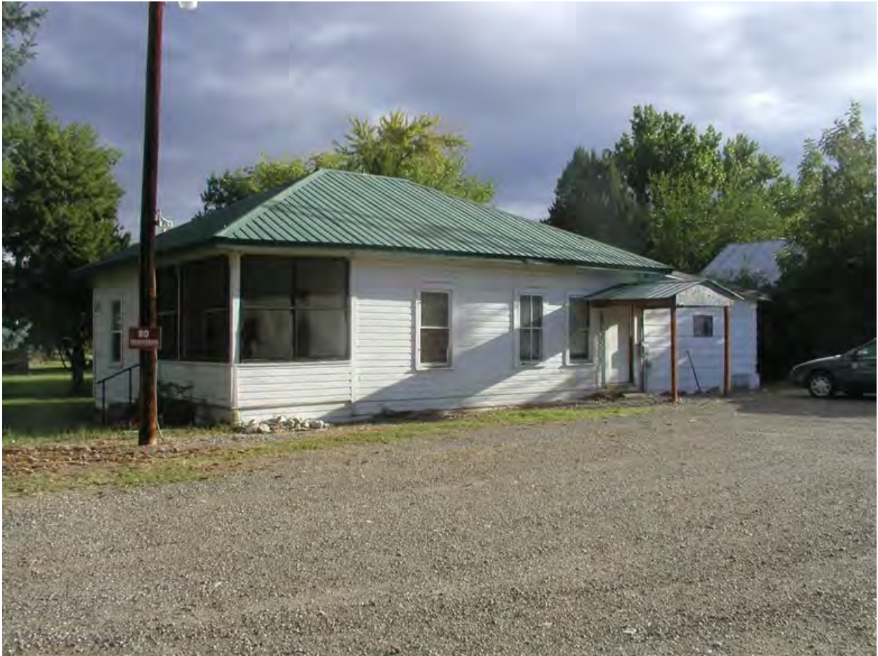
Description and view of camera: South and West elevations, view to north/northeast Photograph: MT_YellowstoneCounty_HuntleyProject Office_0001
