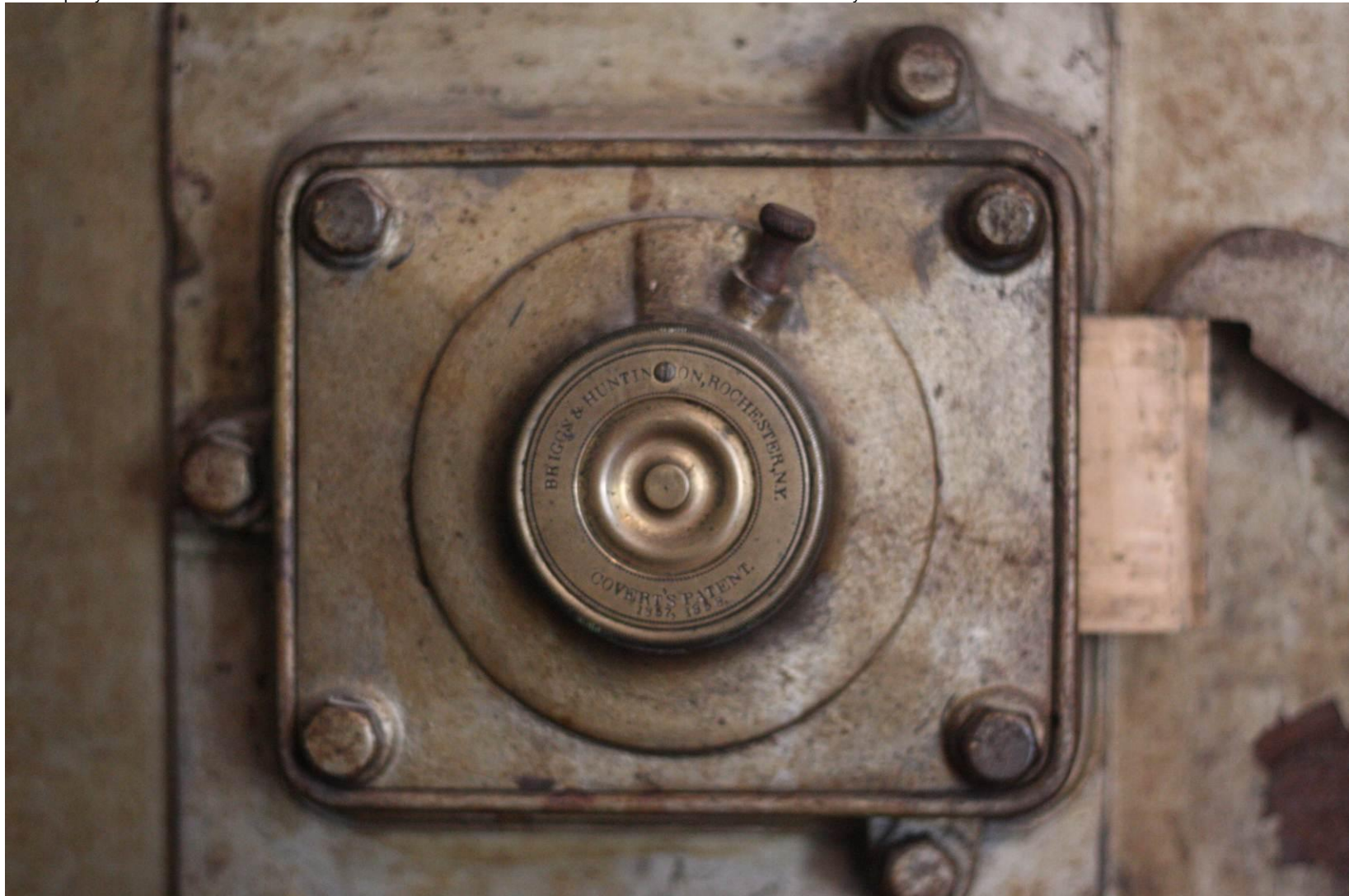
6 of 10 – Looking at a detail of the vault lock.
