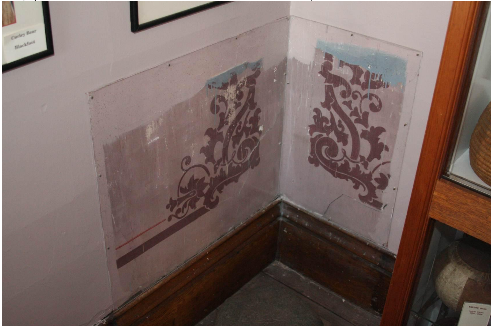
9 of 10 – Looking at a portion of the revealed stenciling located in the southwest corner of the banking room.
