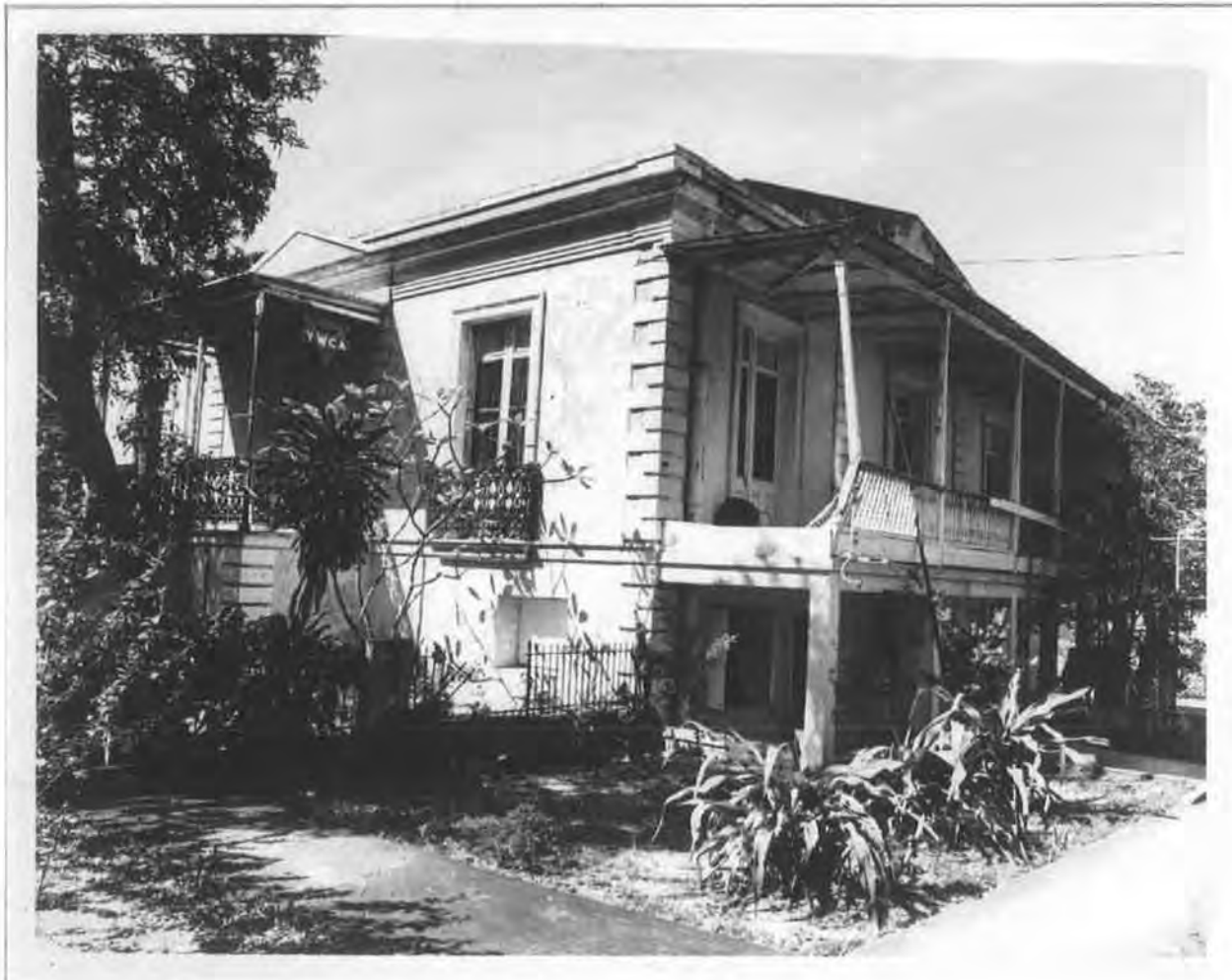
Figure 5. Villa Victoria's eastern façade, after 1979's storm damage; 1979 ca. (Source: YWCA's Archives)
