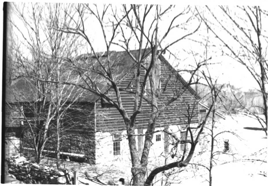
JOHN JAY HOMESTEAD -- MAIN BARN
