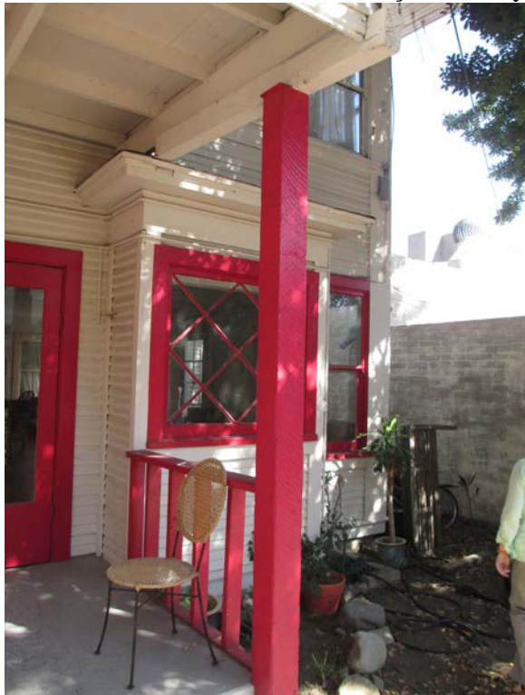
18 of 30. Exterior: Partial west façade, Hollywood School for Girls, view southeast
