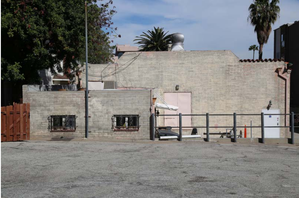
3 of 30. Exterior: West façades of Hollywood School for Girls and Woman's Club from parking lot, view east
