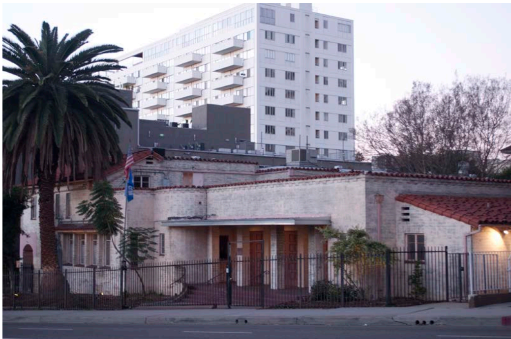
2 of 30. Exterior: East (front) and partial north façade, Woman's Club of Hollywood, view southwest
