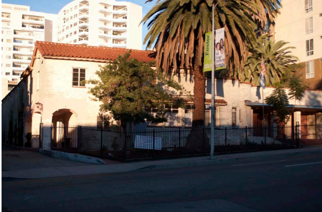
1 of 30. Exterior: Main (east) façade and partial south façade, Woman's Club of Hollywood, view northwest
