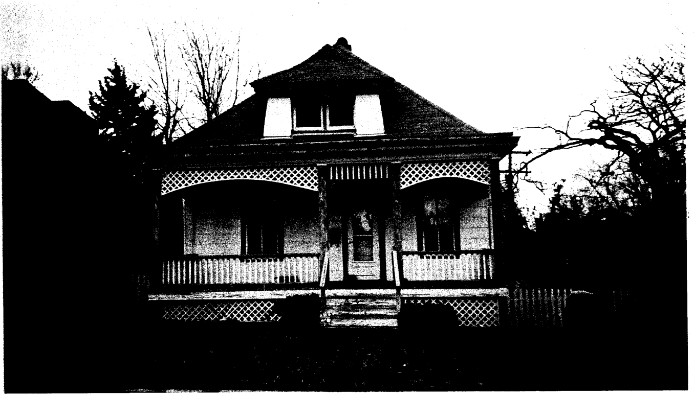
Before removal of the non-historic siding
